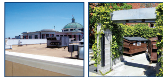
Equipment and trash bins are concealed or enclosed.
