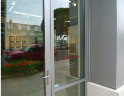
Gallery entry detail where glazing meets metal panel and stone base.
