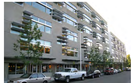
The detailing, craft and quality of design in these fenestrations helps to animate the building and provide for horizontal and vertical variety while not seeming repetitive. The staggered brise soleil and operable windows also serve as sustainable solutions to solar cooling.
