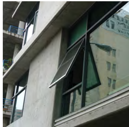
Window detail. Met Lofts building.
