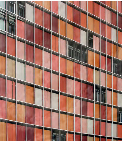
Innovative use of color and active solar building controls.
