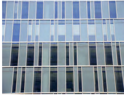
Curtain wall system. LAPD Headquarters building. Architect: AECOM/DMJM.
