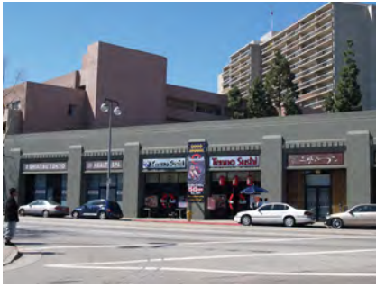
Multi-Tenant Retail Signs. Examples of multi-tenant retail where individual signs are treated in a consistent manner and integrated with the architecture (above).
