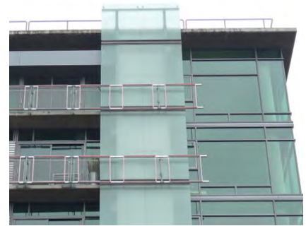
Rooftop mechanical units are not visible.
