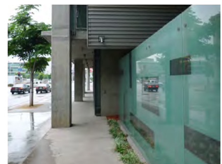
Ground level utilities are screened by this patterned glass wall.
