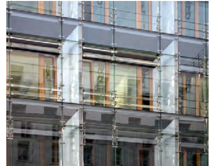
Good example of a glass rain screen that hangs from the structure about five feet from the storefront wall. This solution allows for natural ventilation, sound proofing and modulated privacy for individual units.
