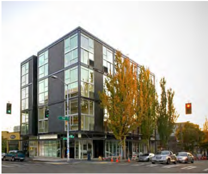
Example of a highly transparent modern facade using a well-detailed window system.
