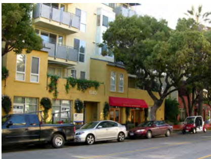
Good examples of an identifiable break between ground level retail and the upper floors.
