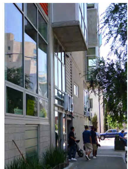
A mix of materials including concrete, concrete masonry units and corrugated metal emphasizes depth and massing.
