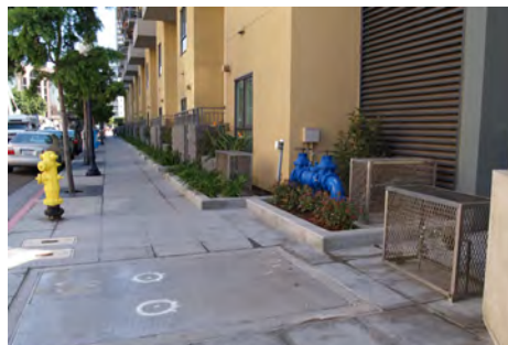
Examples of poor equipment location choices. A primary opening to a courtyard garden is walled off with electric meters (left) and irrigation equipment is in plain view near a building entrance (right).
