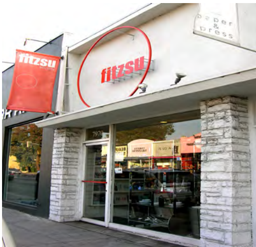
Creative sign enhances building facade.
