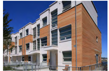
Example of reinforced cement panels on a low-rise residential project.
