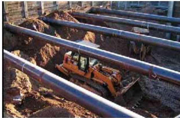
Figure 4-13: Track Loader beneath Struts
