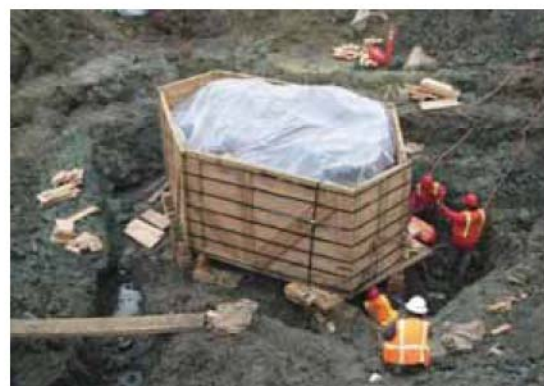
Figure 4-2: Fossil Box Construction at Project 23
