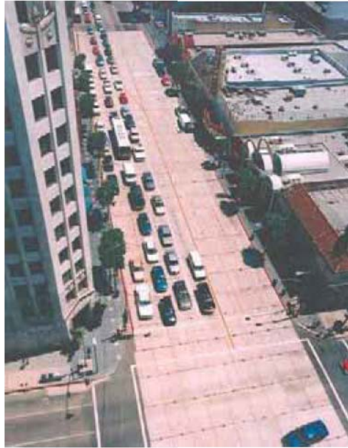
Figure 3-6: Roadway Operations Restored on Temporary Decking System
