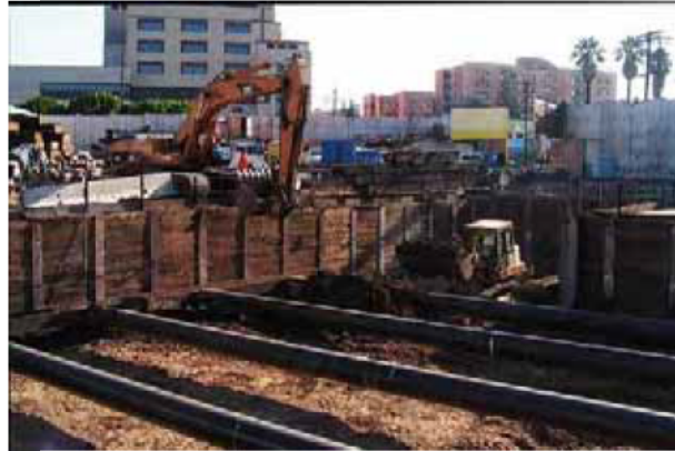
Figure 4-5: Open Cut Excavation of Side Access Shaft
