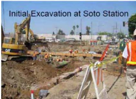
Figure 3-2: Initial Excavation at Soto Station
