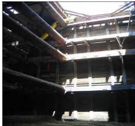
Figure 3-9: Soldier Pile and Lagging
