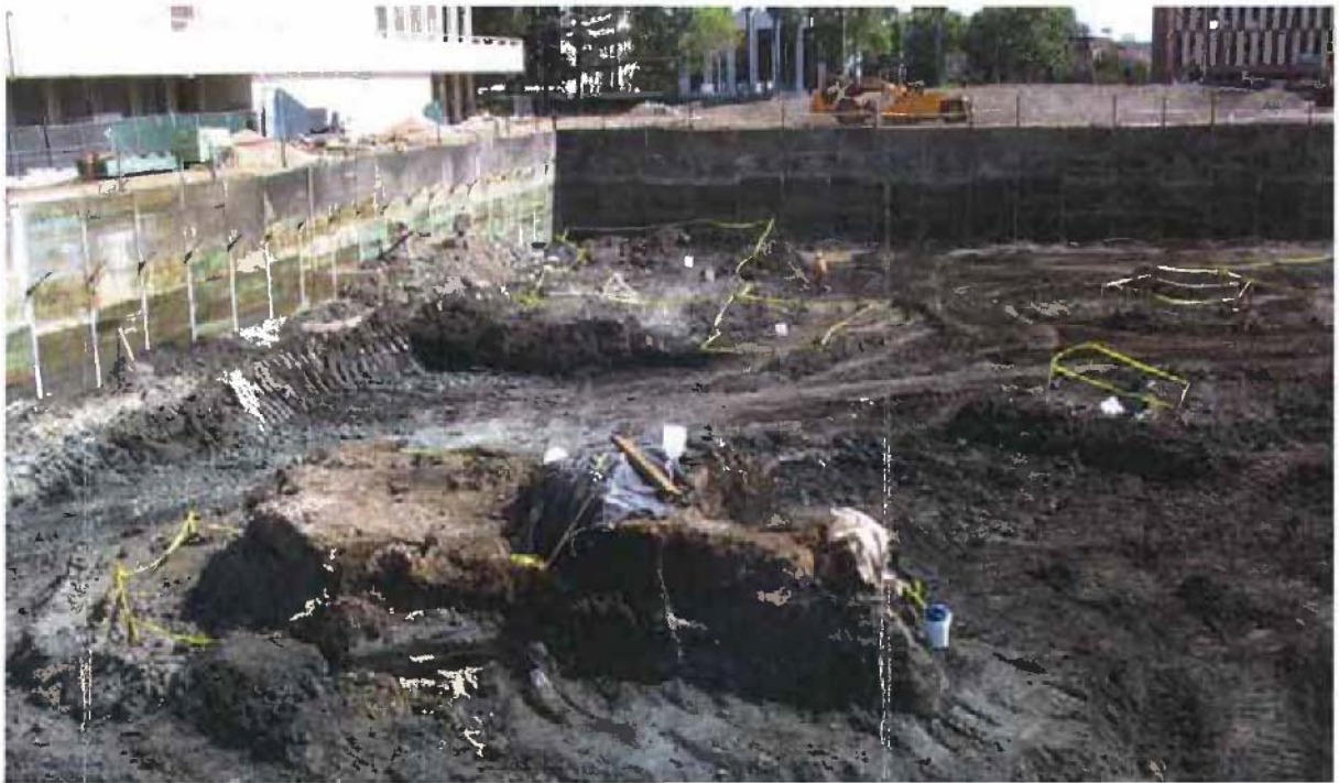
Fig 5: View of east end of LACMA construction site
