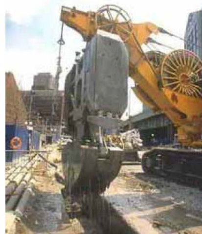
Figure 3-15: Clamshell Digger for Slurry Wall Construction
