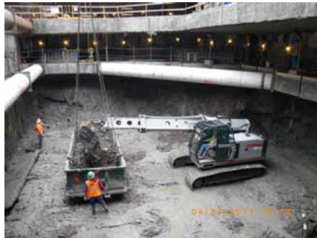
Figure 4-6: Gradall Excavator - East Side Access Project NYC
