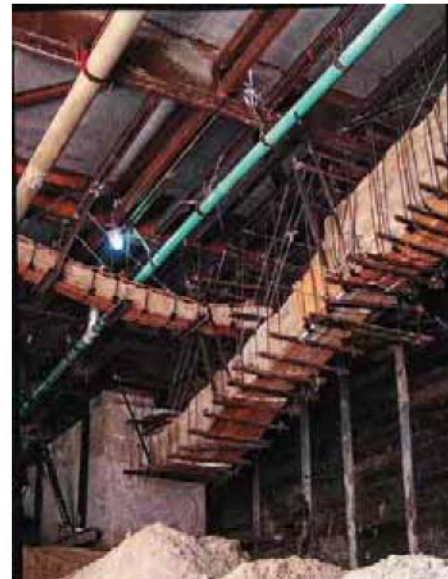
Figure 3-18: Utilities Hung from Deck Beams (Close Up)
