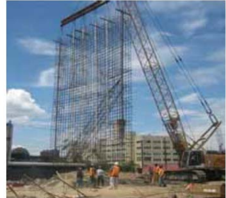
Figure 3-13: Steel Reinforcement Cage for Slurry Wall
