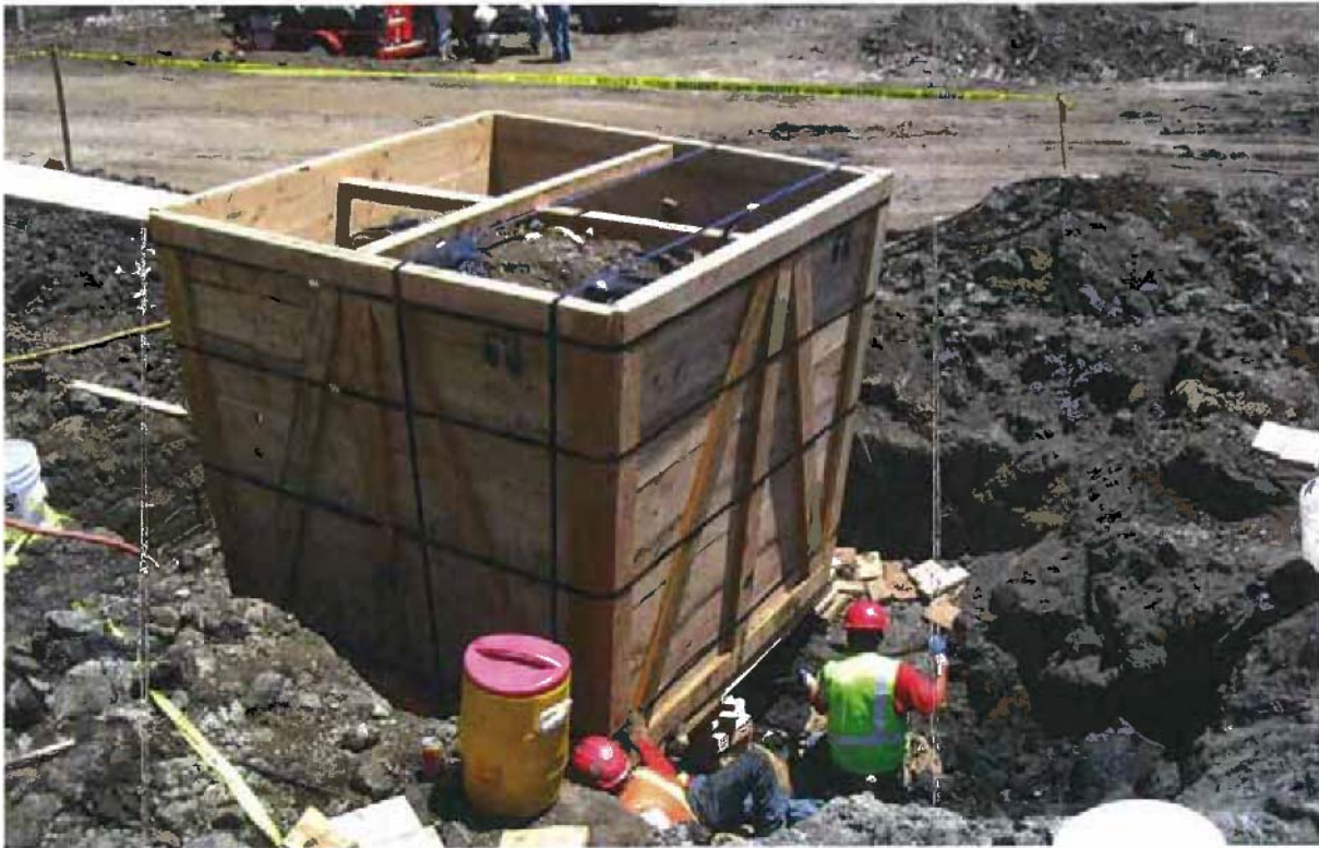
Fig 10: Tunnel under the tree box
