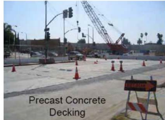
Figure 3-3: Precast Concrete Decking
