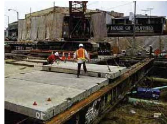
Figure 3-5: Installation of Decking (2 of 2)
