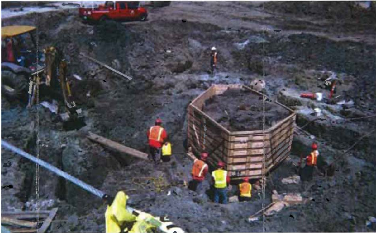
Fig 9: Secure the tree box with metal bands
