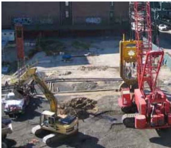
Figure 3-14: Slurry Wall Construction Equipment
