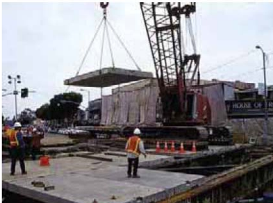
Figure 3-4: Installation of Decking (1 of 2)
