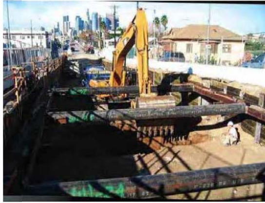
Figure 4-12: Hydraulic Excavator between Struts
