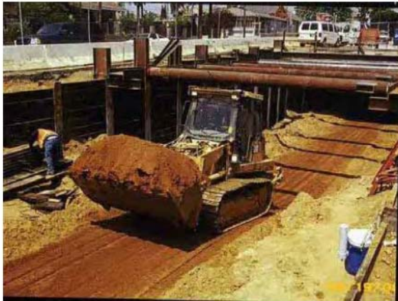
Figure 4-13: Track Loader beneath Struts
