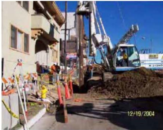
Figure 3-7: Pre-augering for Soldier Pile
