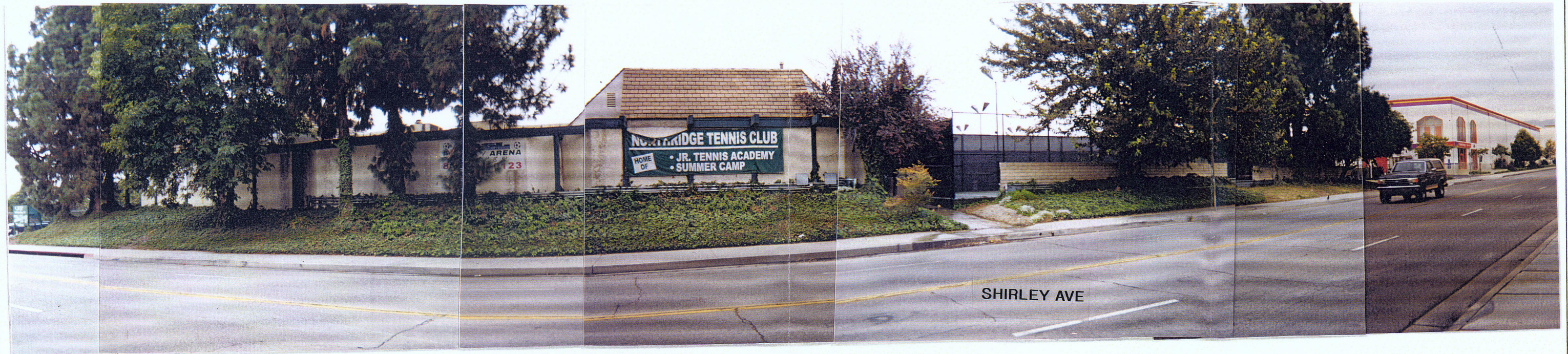
ADD AREA - SHIRLEY AVE LOOKING WEST
