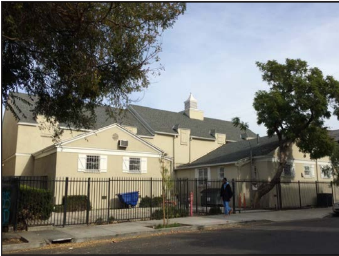
Photo 12: View of existing theatre to remain from Fernwood Avenue, facing northeast.
