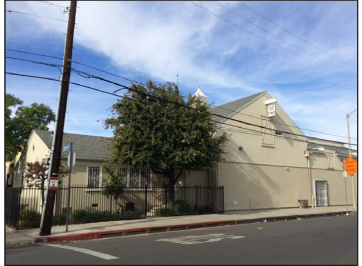
Photo 11: View of existing theatre to remain from St. Andrews Place, facing west.
