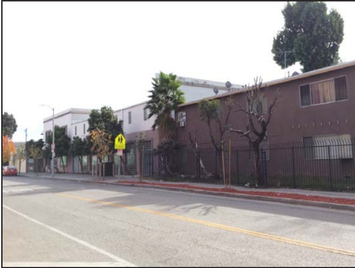
Photo 1: View of westerly adjacent property facing southeast.
