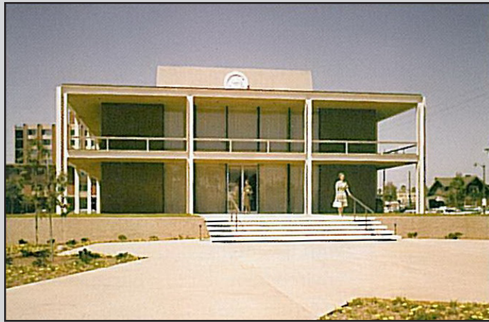
The Registration Building, by Ladd & Kelsey, is an excellent example of the International Style on campus (Courtesy of USC University Archives)
