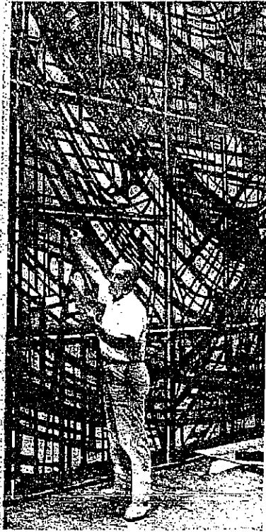
ARTIST—Roger Darricarrere works on master pattern for the 1,300 sq. ft. mosaic skylight for Columbia Savings and Loan Assn.'s Wilshire Office.
