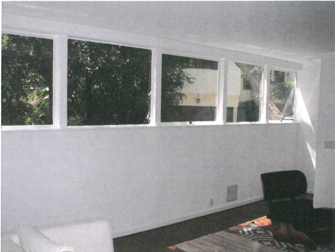
Polito House, window band, 1650 Queens Road April 14, 2014 (Photograph by Charles J Fisher)
