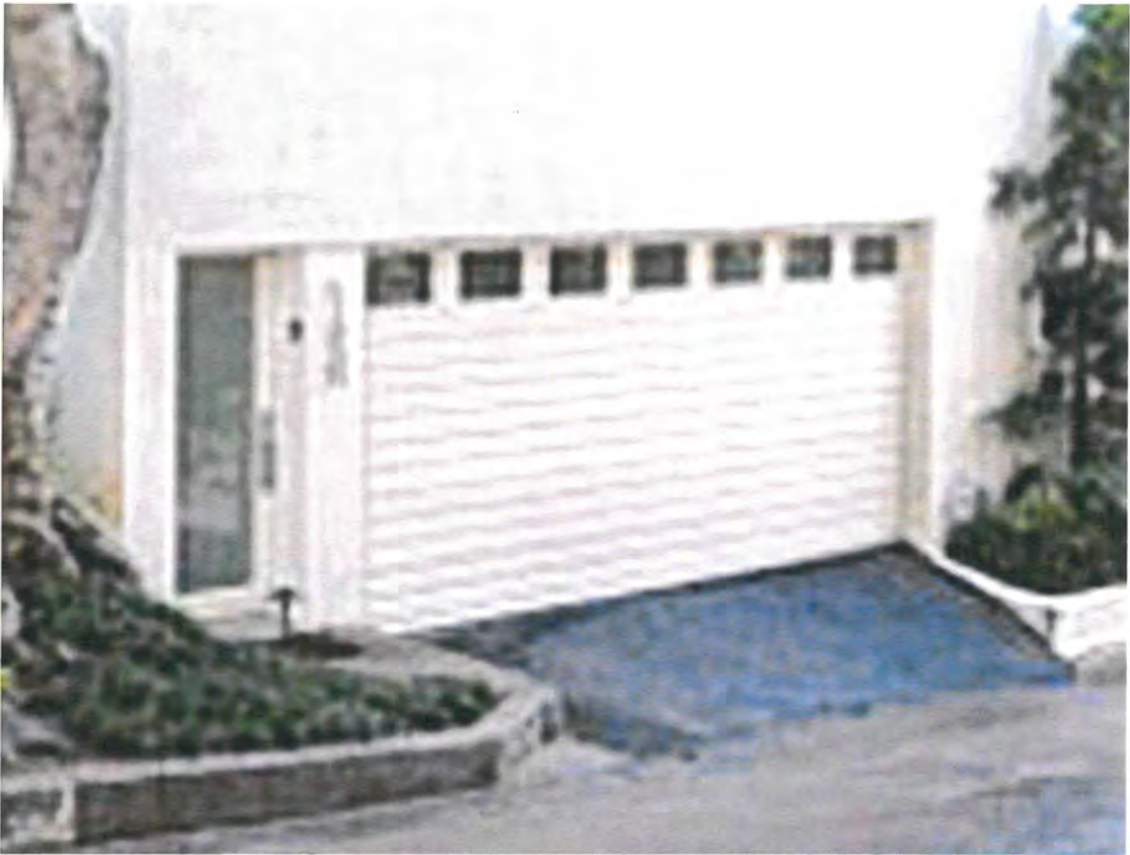
Polito House, front door and garage door, 1650 Queens Road February 10, 2013 (Photograph by David Kubiczky)
