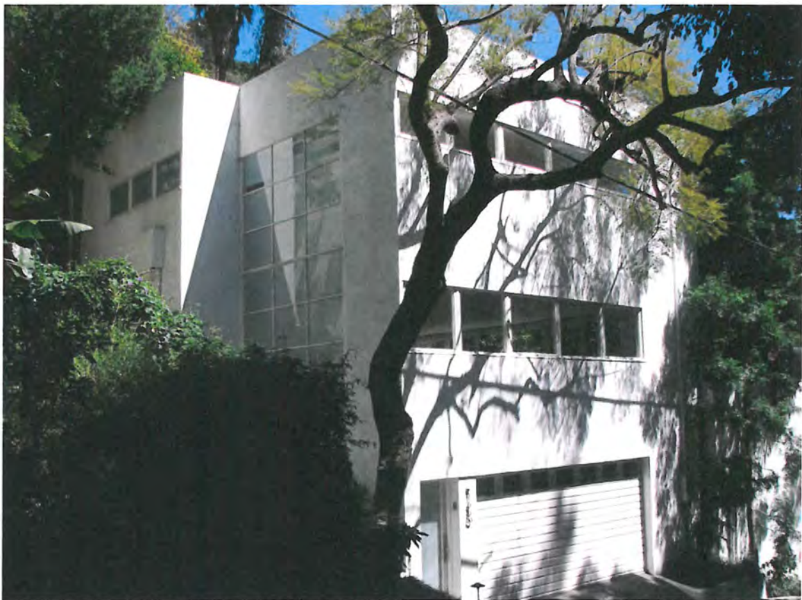
Polito House, West facade, 1650 Queens Road April 14, 2014 (Photograph by Charles J Fisher)
