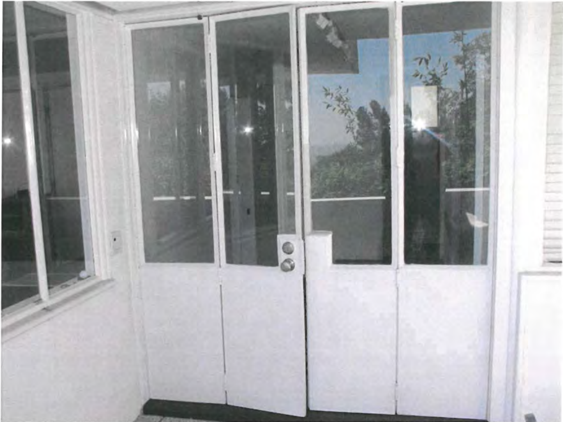
Polito House, original folding doors on East facade, 1650 Queens Road April 14, 2014 (Photograph by Charles J Fisher)
