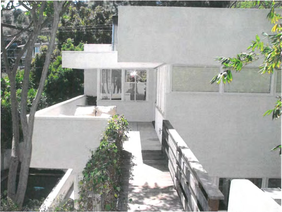
Polito House, view from bridge reminiscent of Lovell Health House, 1650 Queens Rd April 14, 2014 (Photo by Charles J Fisher)
