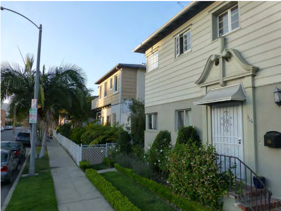
B 4. Sidewalk view of 118-124 N. Flores looking north from Wesley Holler building
