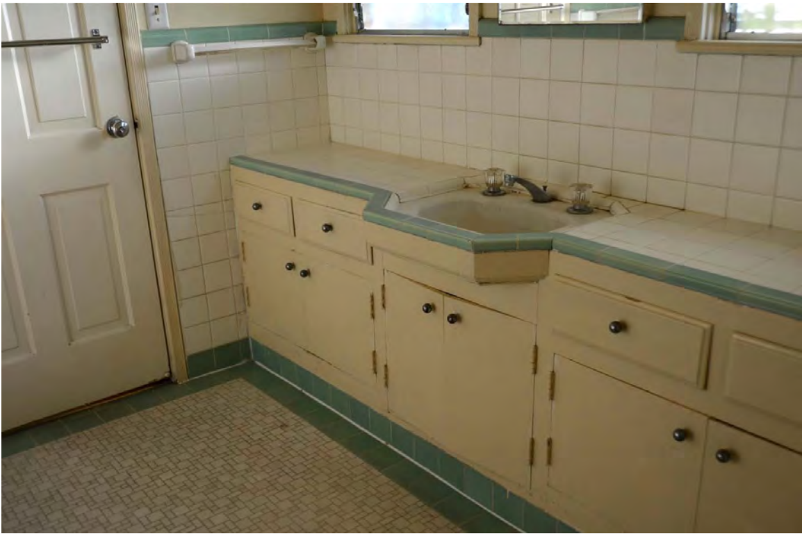
N 6 . Jade colored tile in bathroom of 124 N. Flores with original angled sink cabinet
