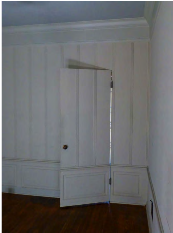
M 13. "Secret door" in dining room paneled wall in 126 N. Flores
