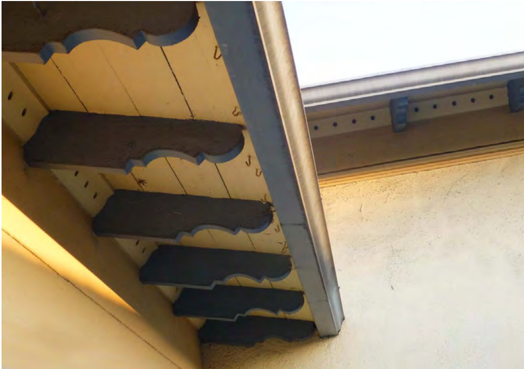
E15. Roof overhang bracket detail on side balcony of 124 N. Flores
