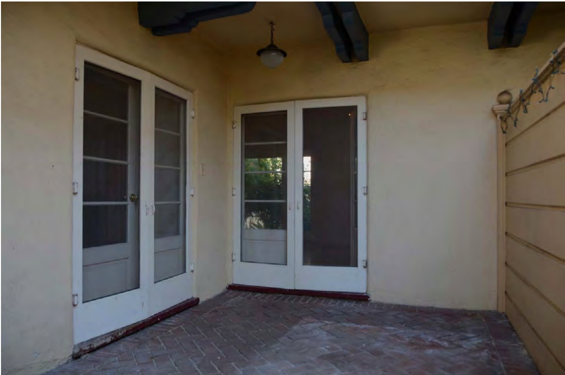
M 10. Private patio of 126 N.Flores with oversized corbels supporting balcony above
