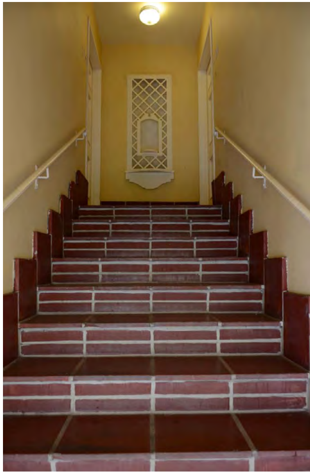
G7. Stair hall for 118 ½ and 120 Flores
