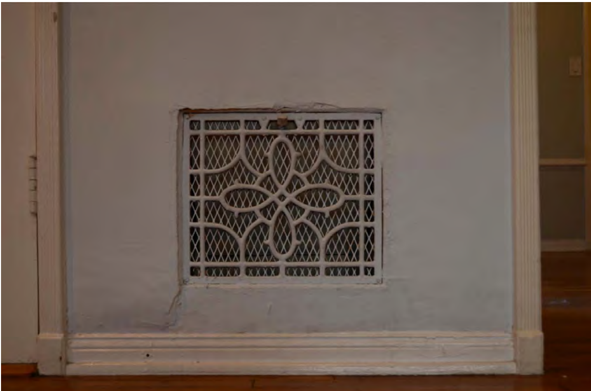
M 14. Heating vent detail in 126 N. Flores
