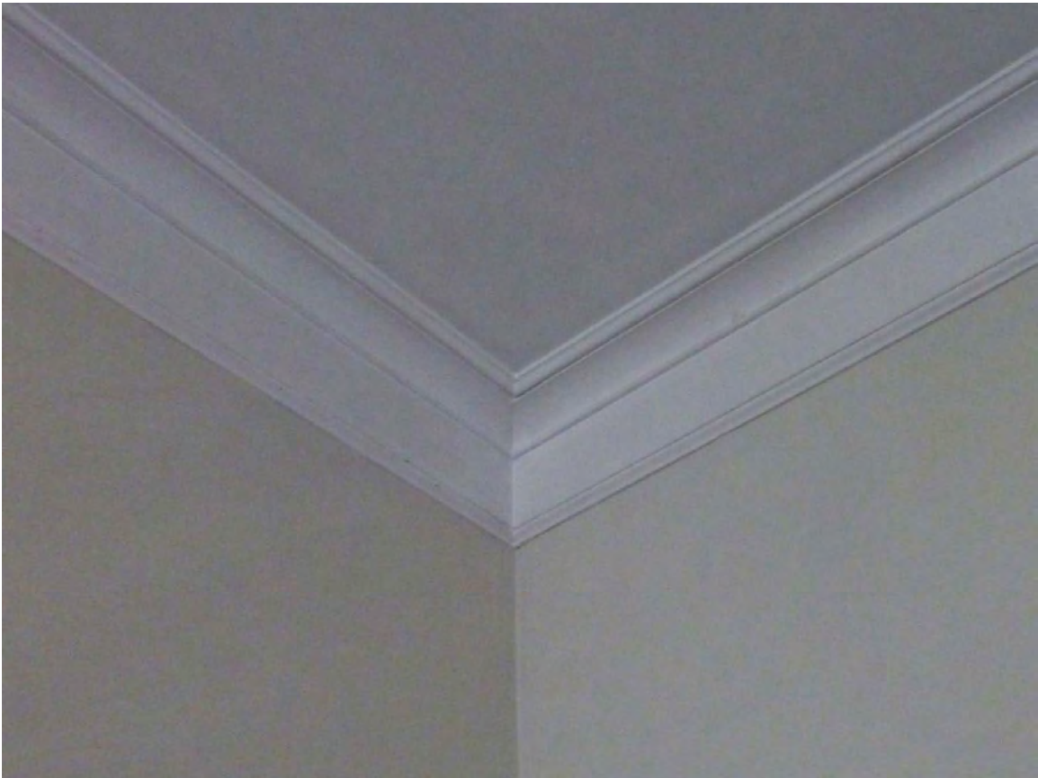
K 4. Ceiling plaster molding in 120 N. Flores
