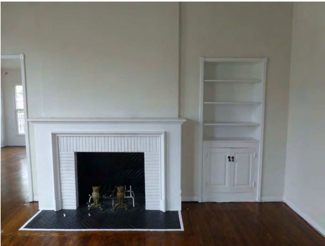
L 2. Colonial style fireplace and built-in cabinetry details in 124 ½ N. Flores
