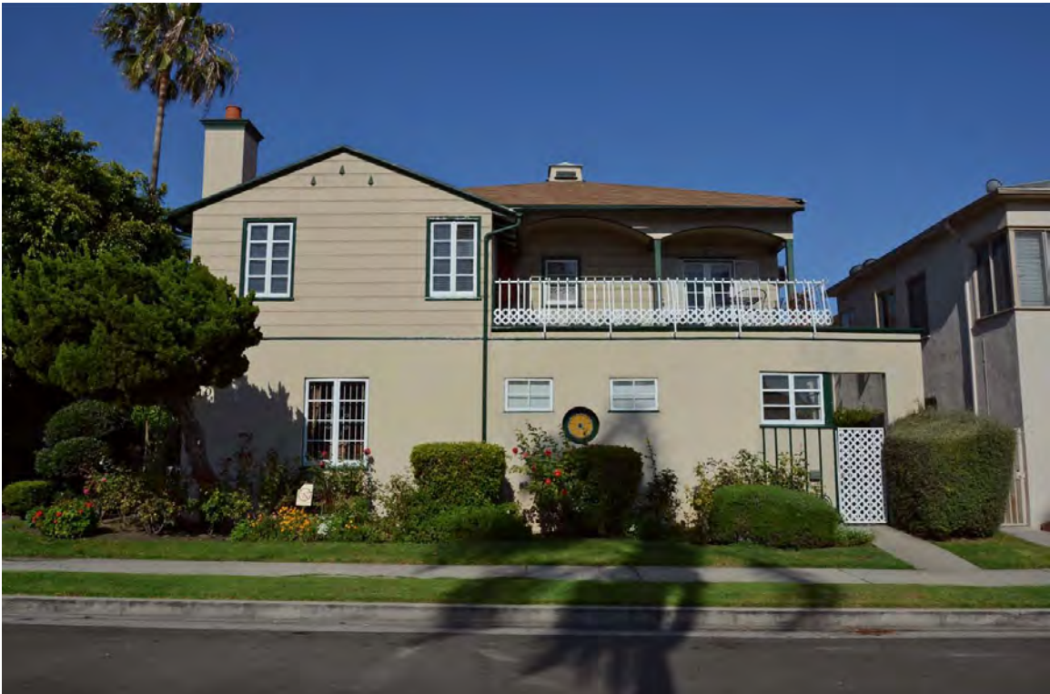
A 2. 106-110 N. Flores, Wesley Holler building two doors from nominated buildings
