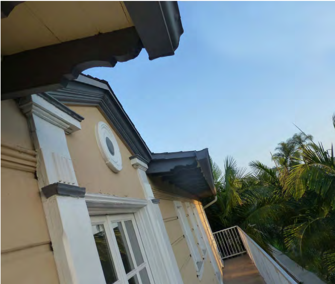
I4. Front overhanging balcony of 126 N. Flores looking south
