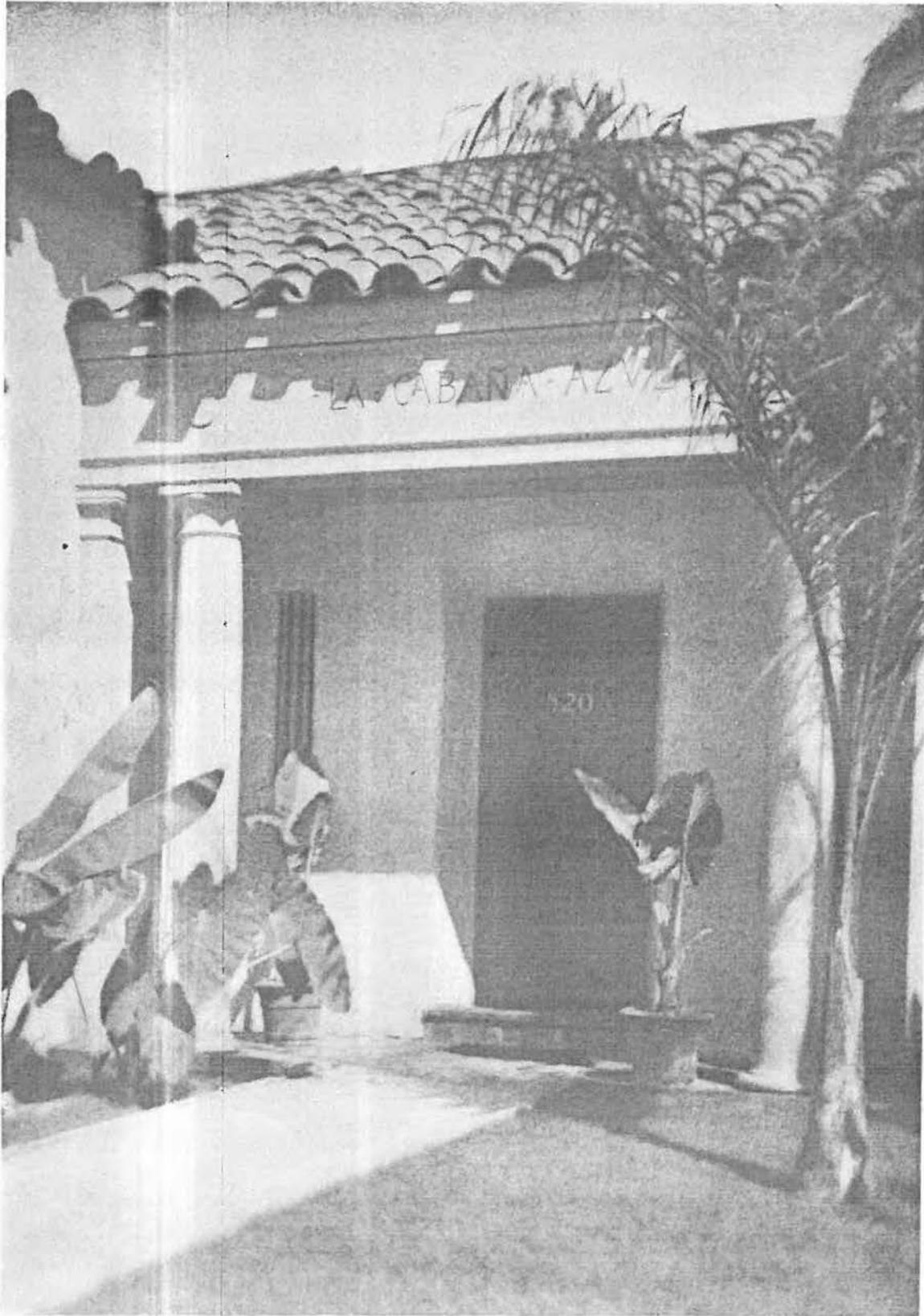
DETAIL OF FRONT ENTRANCE, LA CABANA AZUL, STUDIO OF H. H. WHITELEY, ARCHITECT, LOS ANGELES, CALIFORNIA H. H. WHITELEY, ARCHITECT
