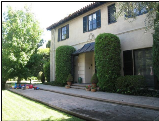
Primary, west elevation, view east
