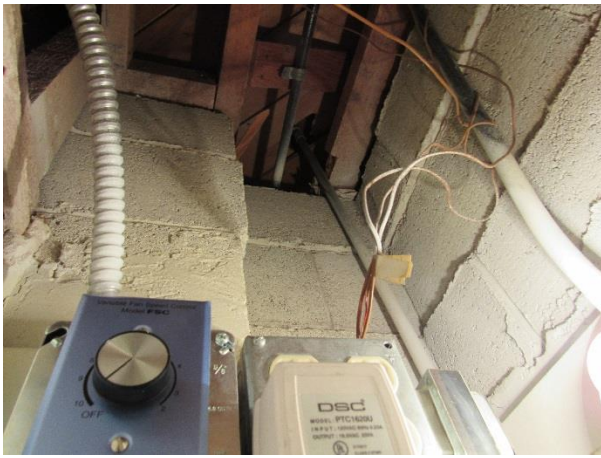
FIGURE 111. Variable fan speed controller.
