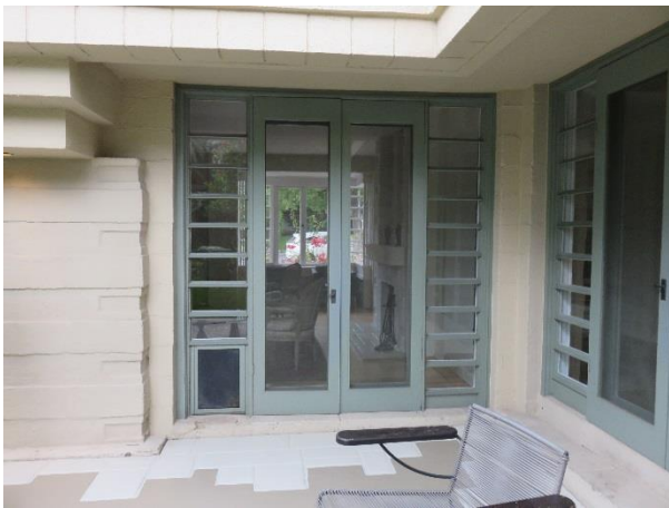
FIGURE 42. First floor exterior door leading to the patio.
