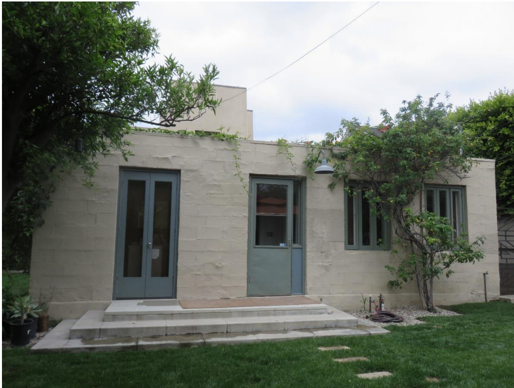
FIGURE 18. View of the north end of the east elevation of the Bollman House.
