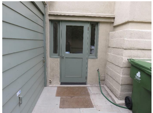
FIGURE 48. North elevation door leading into laundry room.
