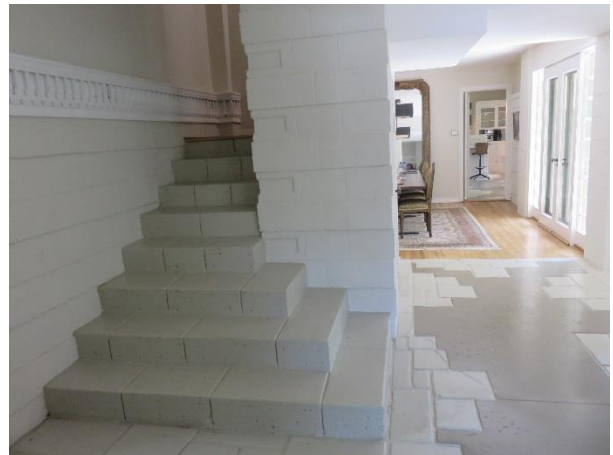
FIGURE 74. Stairs at the north end of the entrance hall.
