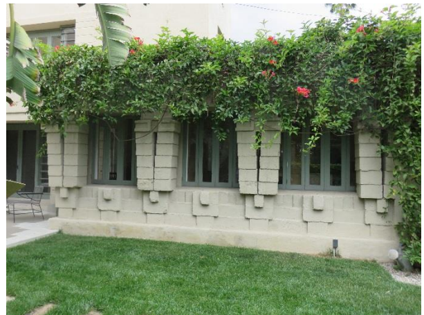
FIGURE 25. Concrete block wall construction at the south wall.
