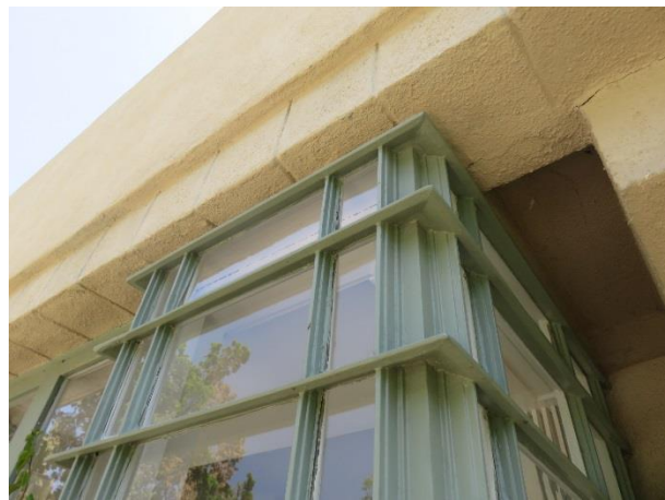
FIGURE 36. Sloped muntins at the corner of the west facade bay window.
