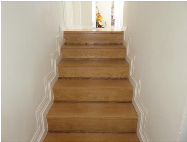
FIGURE 76. Wood treads and risers with wood trim.
