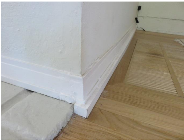
FIGURE 112. Floor grille in the dining room.
