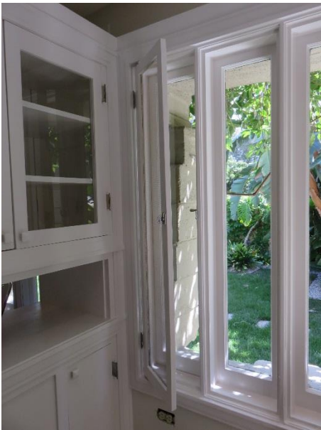
FIGURE 28. Single light casement unit at the pantry.
