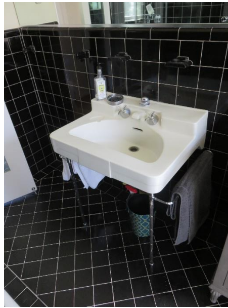
FIGURE 103. Second floor bathroom console sink with brass stand and fixtures.
