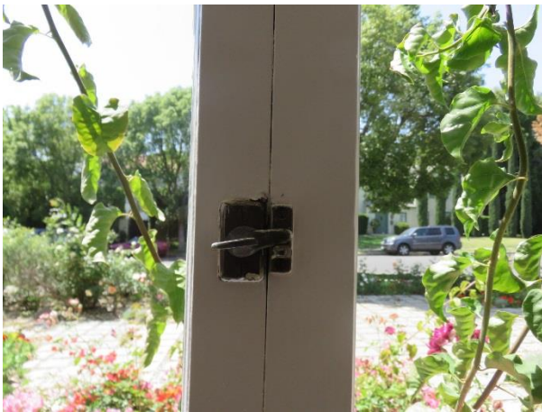
FIGURE 34. Typical window closure hardware.
