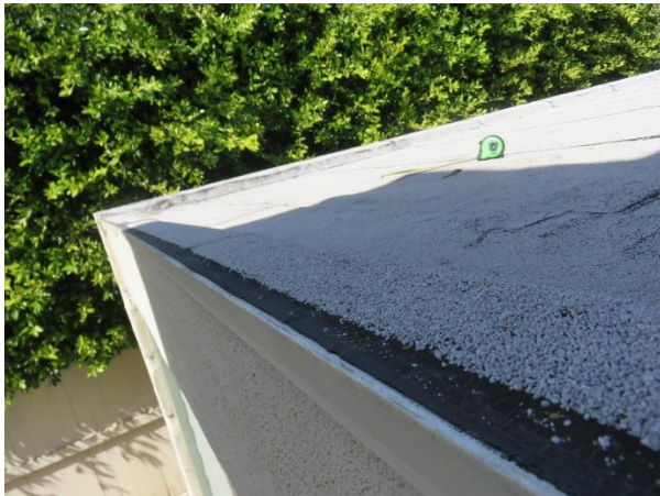
FIGURE 55. Rolled roofing lapped over the sheet metal perimeter flashing.
