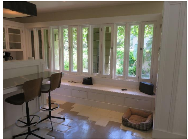
FIGURE 29. Replacement casement windows at the south wall of the kitchen.
