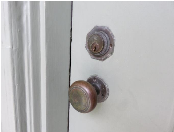
FIGURE 50. Brass hardware on the main entrance door.
