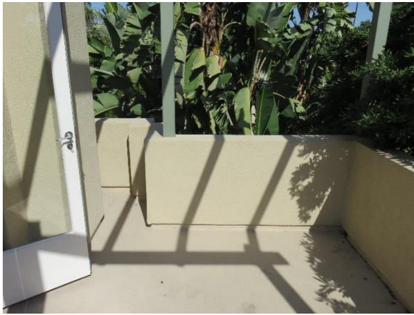
FIGURE 21. Overall view of the south balcony.
