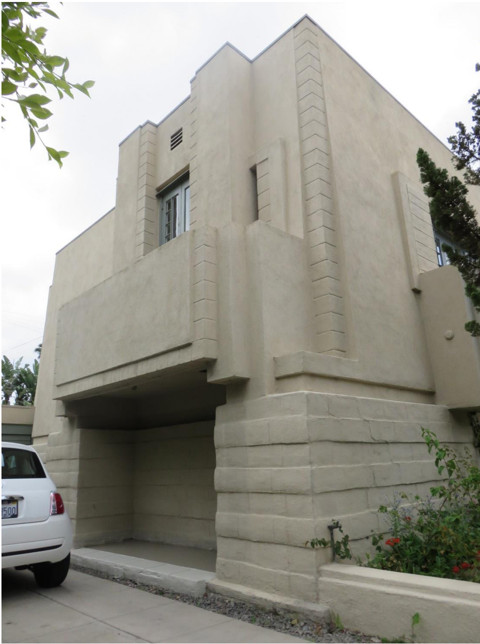
FIGURE 15. Partial view of the north elevation of the Bollman House.
