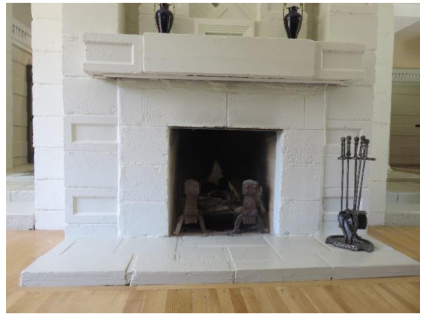
FIGURE 83. Close-up view of the hearth from the living room.
