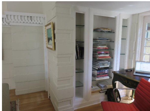
FIGURE 80. Built-in shelving in the nook at the south end of the living room.
