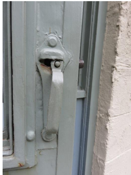
FIGURE 47. Sliding handle on the Kalamein door on the east facade.
