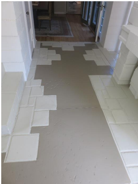
FIGURE 72. Part of the concrete slab at the entrance hall.
