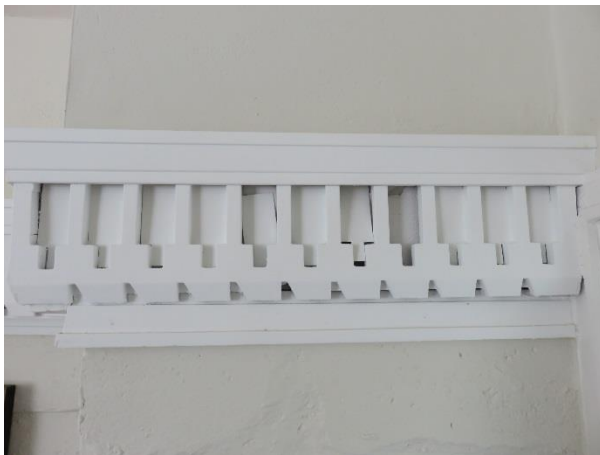
FIGURE 73. Typical wood trim on the first floor.
