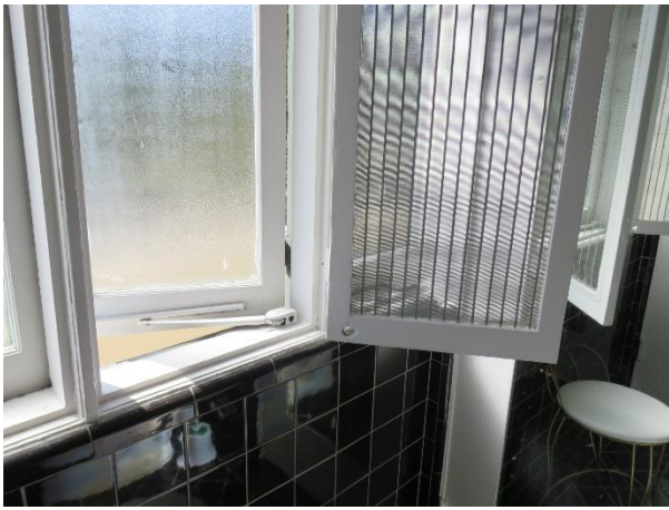
FIGURE 32. Fritted screen at the second floor bathroom.
