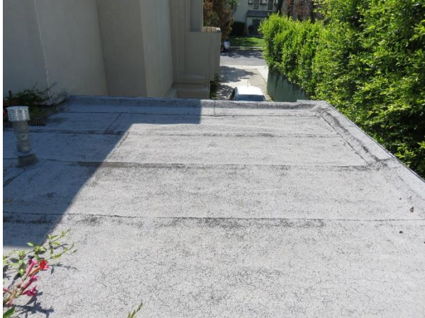
FIGURE 54. North portion of first floor roof.
