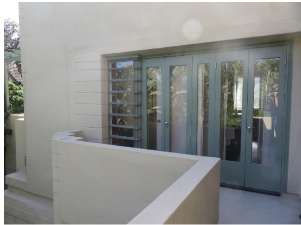
FIGURE 52. Second floor exterior paired door leading to a balcony.
