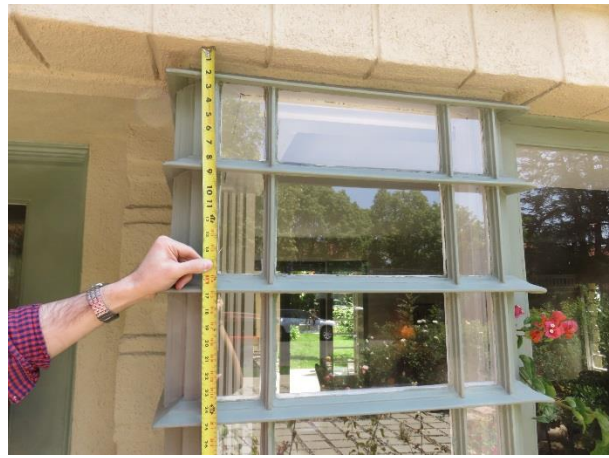
FIGURE 35. Muntin spacing is 8 inches vertically, matching the concrete block joints.
