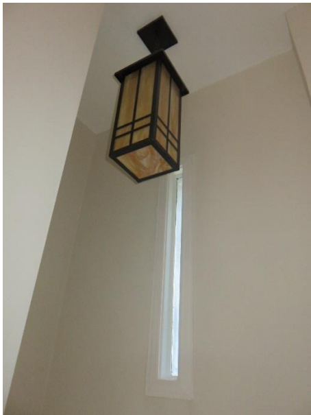
FIGURE 39. Slit window at the north wall of the staircase.
