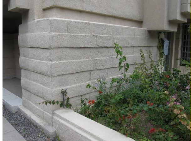
FIGURE 19. Concrete block wall construction at the south wall.
