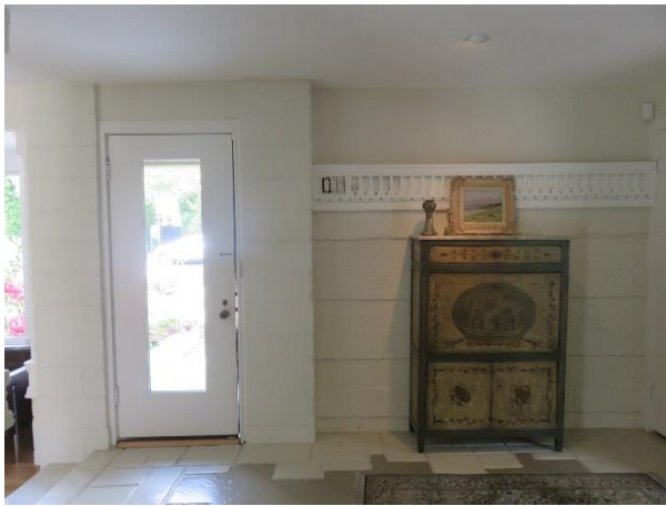
FIGURE 71. West wall of the entrance hall, with the main entrance door.
