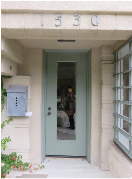
FIGURE 49. Main entrance door on the west elevation.
