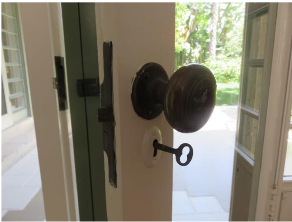
FIGURE 41. Typical exterior door hardware.
