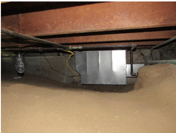
FIGURE 113. Crawlspace below the dining room.
