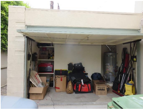
FIGURE 92. Overall view of the garage.
