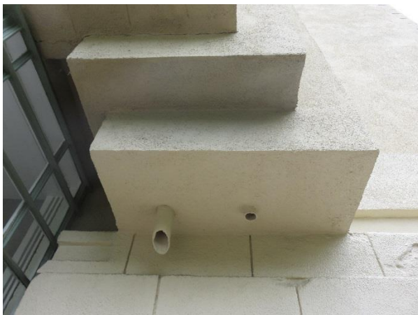
FIGURE 23. Downspout at the underside of the west balcony.
