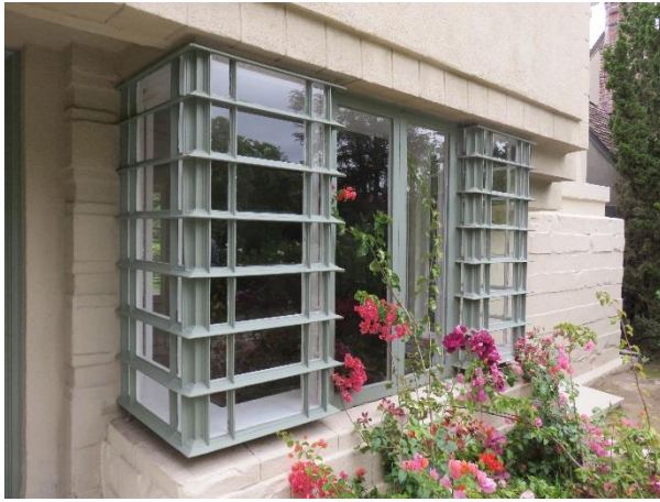
FIGURE 38. Bay window with casement and fixed sidelights, on the west elevation.
