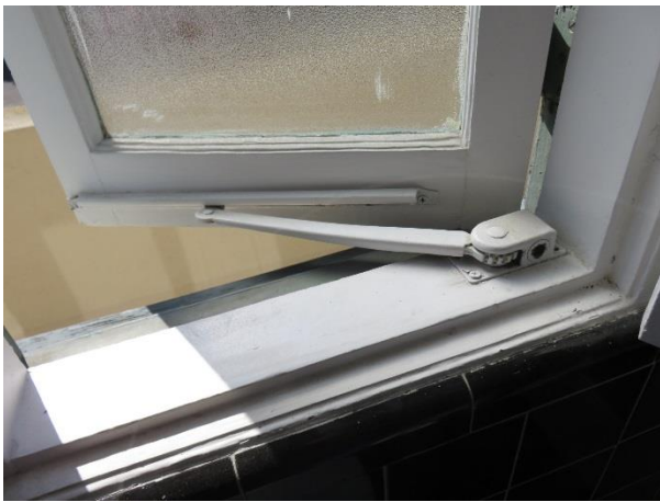
FIGURE 33. Casement window gear crank hardware.
