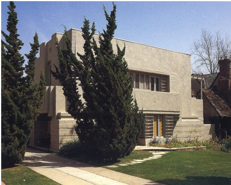
Figure A-2. Front exterior.
