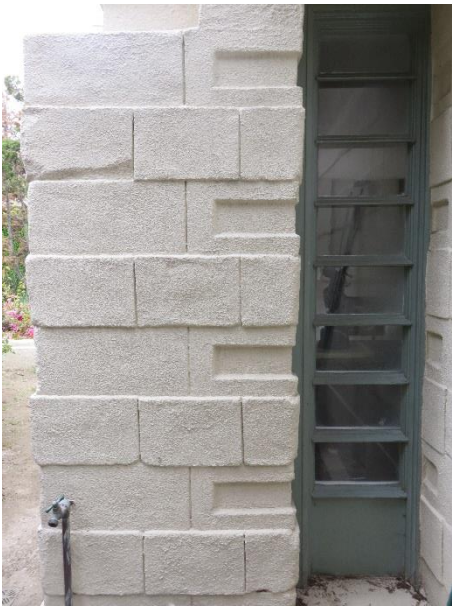
FIGURE 27. Multi-light fixed window at the south wall of the living room.
