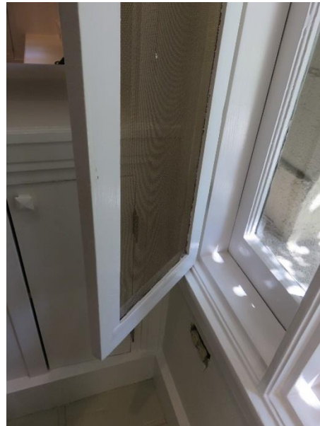
FIGURE 31. Typical wood framed insect screen.
