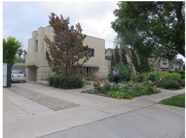
FIGURE 4. View of the Bollman House, with the driveway and sidewalk adjacent to the house in the foreground.
