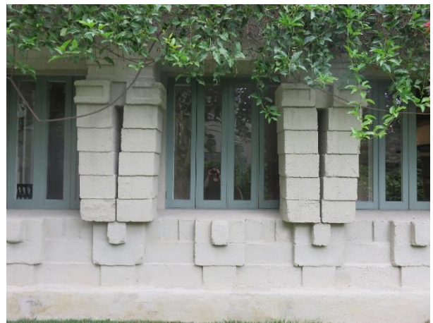
FIGURE 30. Exterior view of replacement casement windows at the kitchen.
