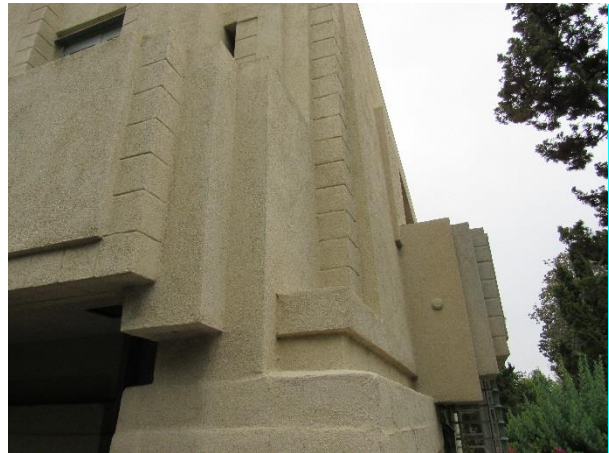
FIGURE 20. Concrete block wall construction at the balconies.
