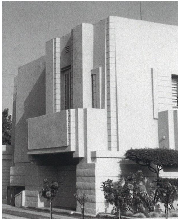
Figure A-5. Exterior detail, 1960.
