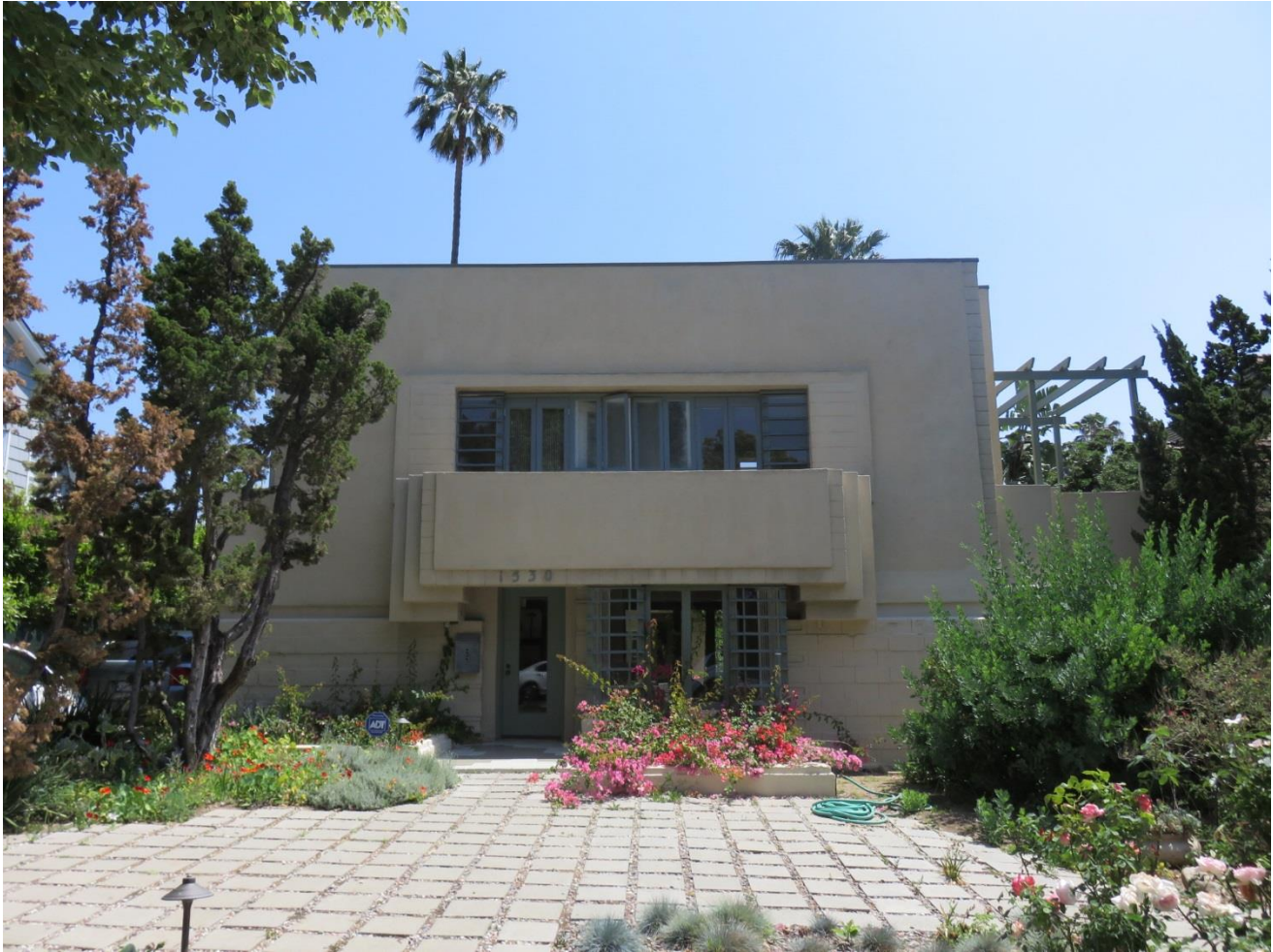
FIGURE 14. Overall view of the west elevation of the Bollman House.
