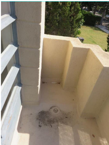
FIGURE 22. Typical deck drain leading to downspout through deck.
