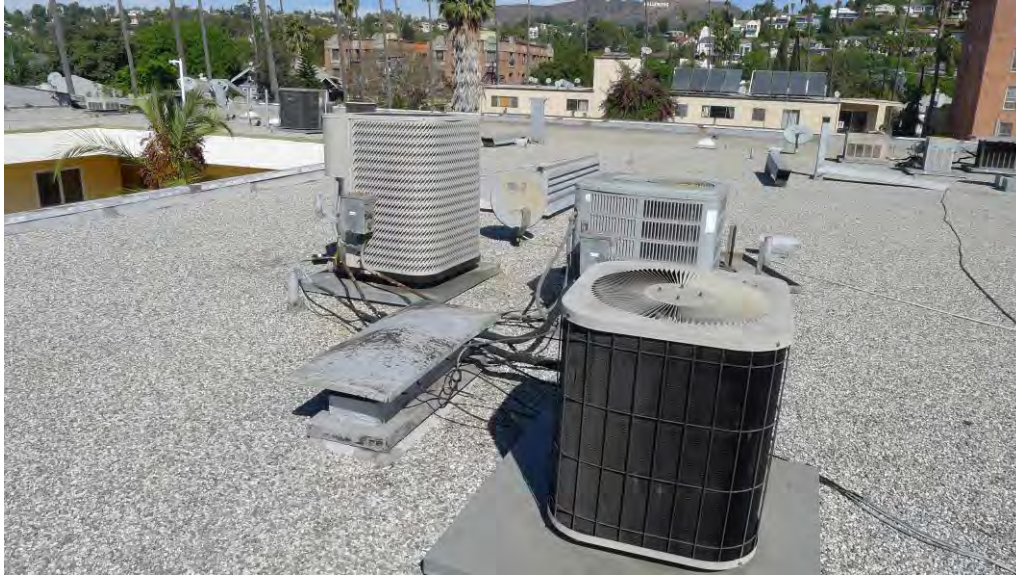
Figure 5: Units with no visible anchorage
