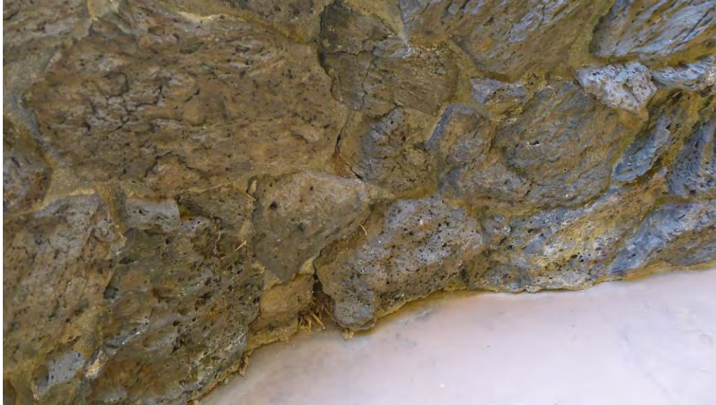
Figure 15: Roots growing out of cracks of the planter
