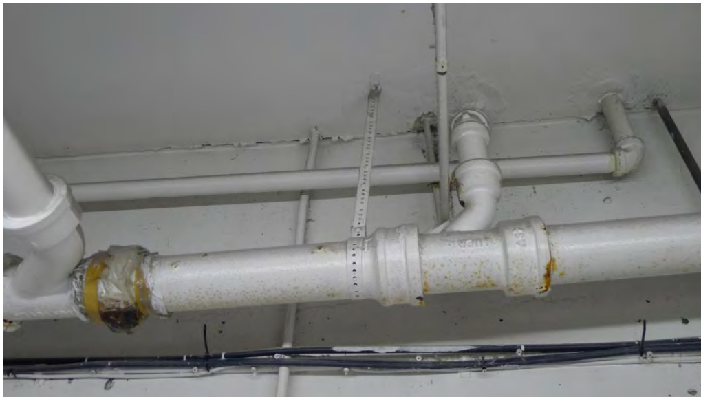
Figure 20: Previous patch work at penetration of concrete structural slab
