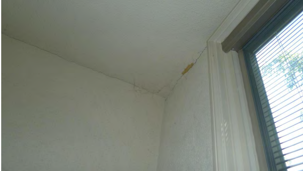
Figure 19: Minor cosmetic crack inside unit
