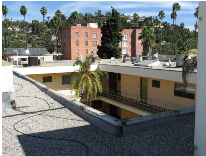
Fig. 2-31 Ballasted flat roofing
