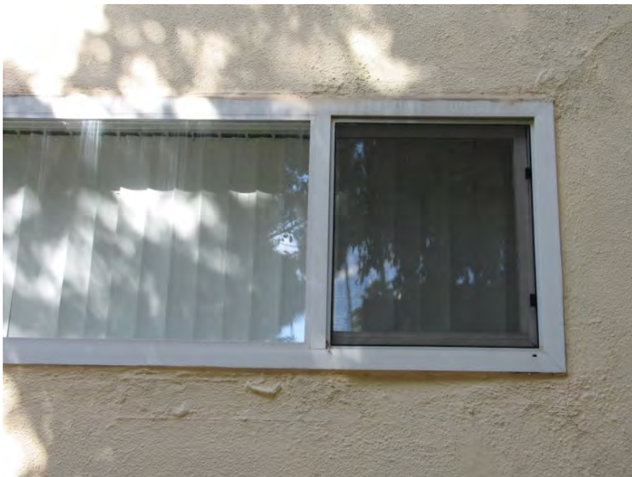
Fig. 2-26 Newer vinyl slider window on North facade
