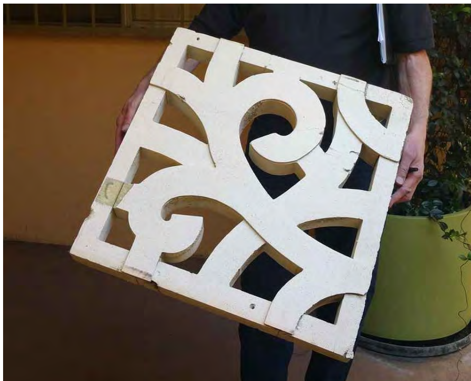
Fig. 2-7 Architectural screen panel blown down in a recent windstorm
