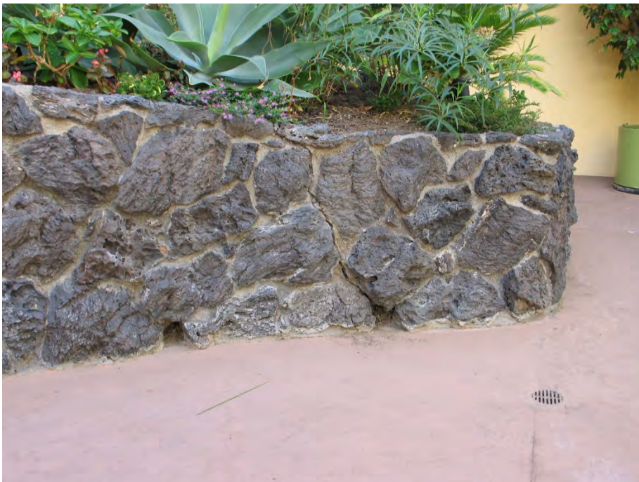
Fig. 2-18 Crack in lava stone planter
