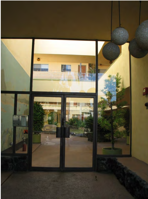
Fig. 2-9A Aluminum storefront style entry door
