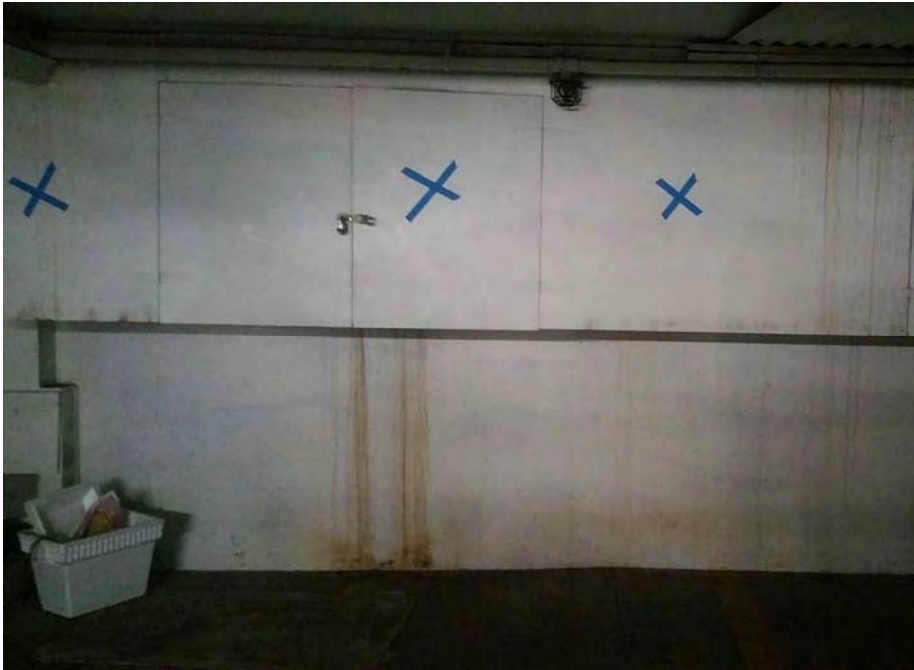
Fig. 2-23 Rear wall of garage showing water damage from rear podium cracks
