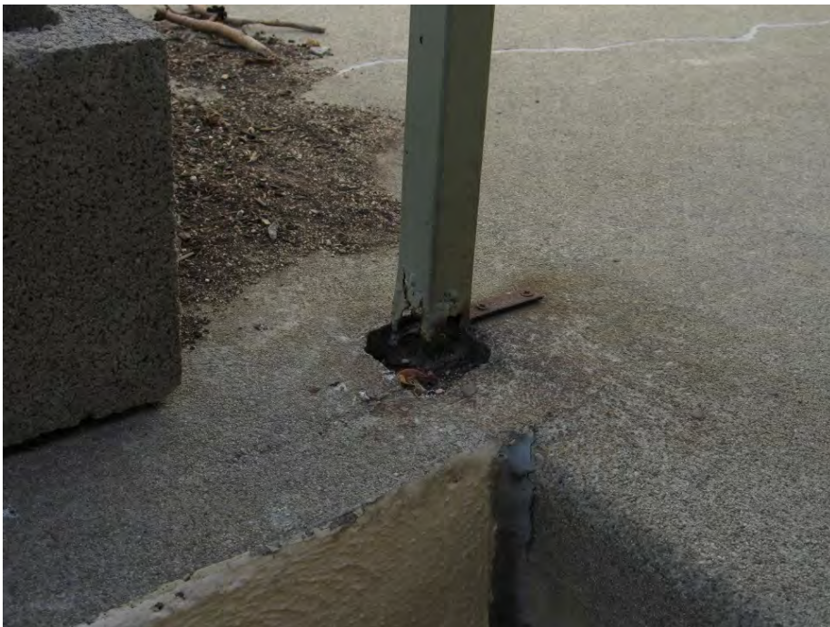
Fig. 2-22 Railing with extensive corrosion
