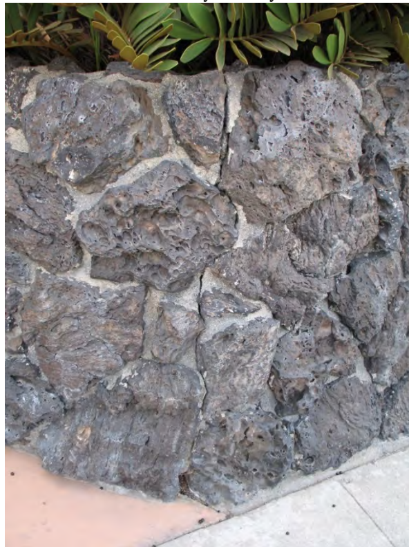
Fig. 2-12 Street entry Lava stone planter with crack
