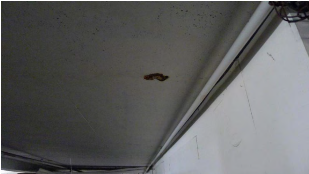
Figure 22: Rust stain at concrete structural slab in garage
