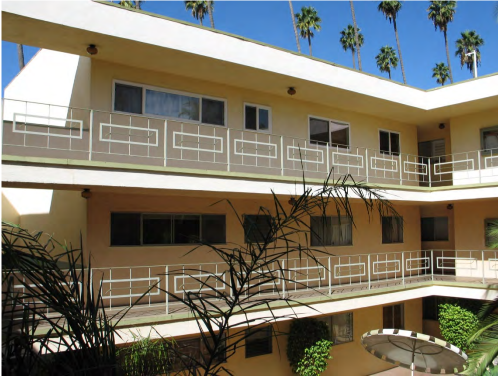
Fig. 2-15 Cantilevered walkways with guardrails. Note upper apartment with newer vinyl slider windows
