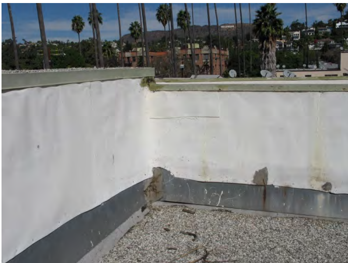
Fig. 2-32 Ballasted flat roofing and parapet (facing street)
