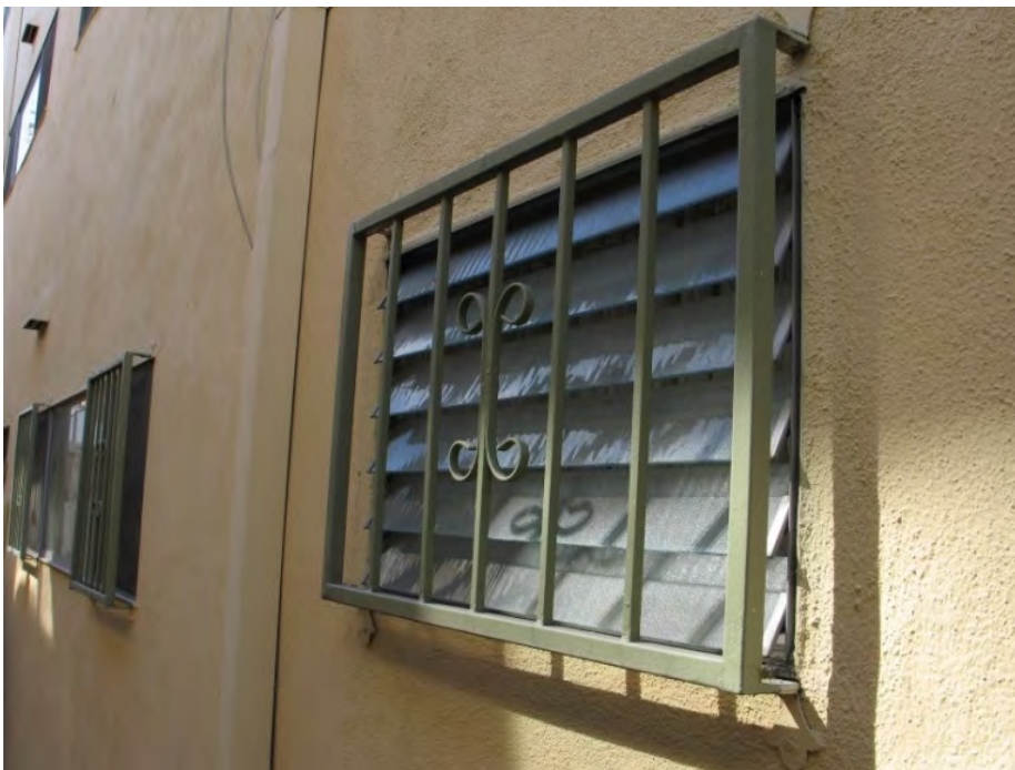
Fig. 2-24 Original jalousie window on North facade
