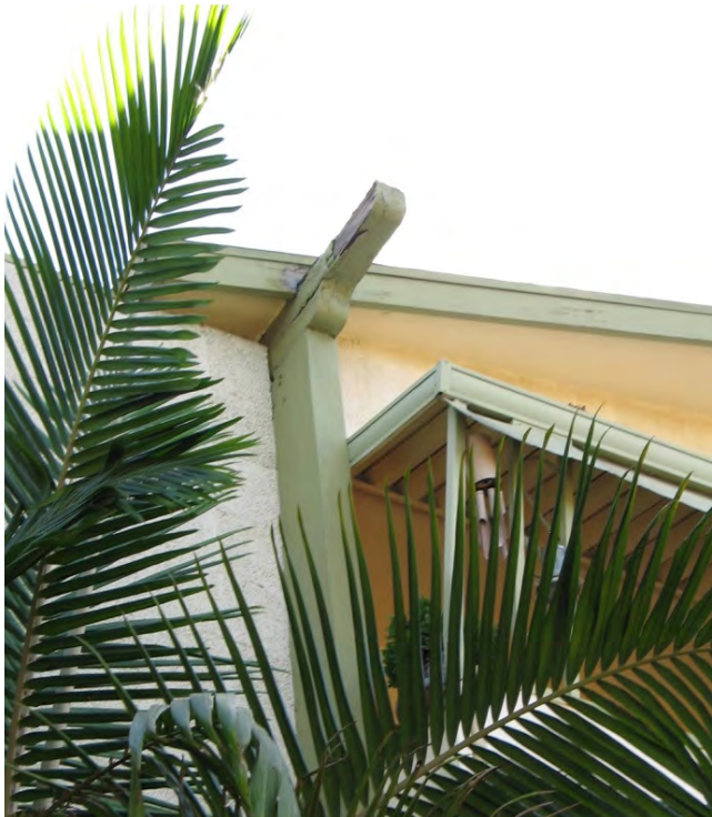
Fig. 2-29 Painted fascia and outrigger - rotting
