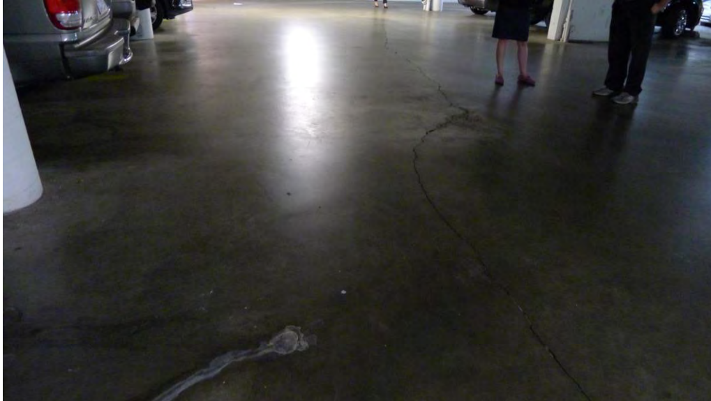
Figure 23: Cracked concrete in basement with evidence of previous patchwork
