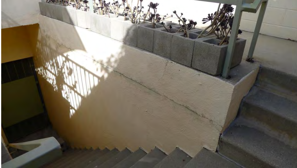
Figure 27: Crack in concrete and rusted railing
