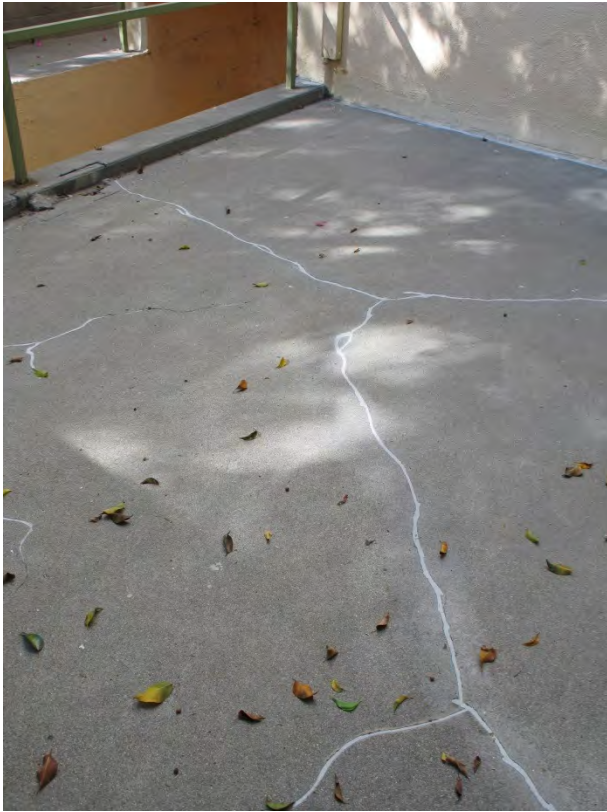
Fig. 2-20 Rear podium deck cracking
