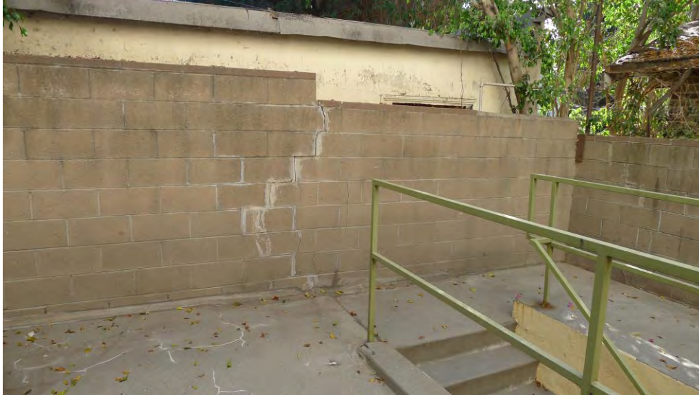
Figure 25: Cracked CMU wall at back of property
