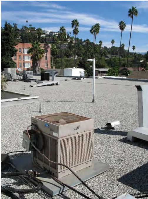
Fig. 2-30 Ballasted flat roofing
