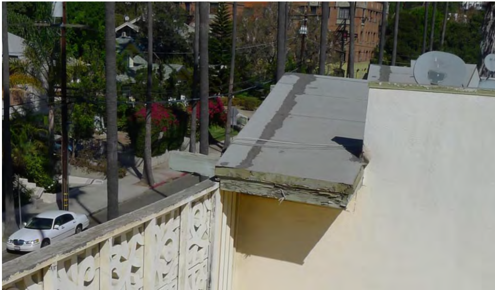
Figure 6: Deterioration of exposed roof beam
