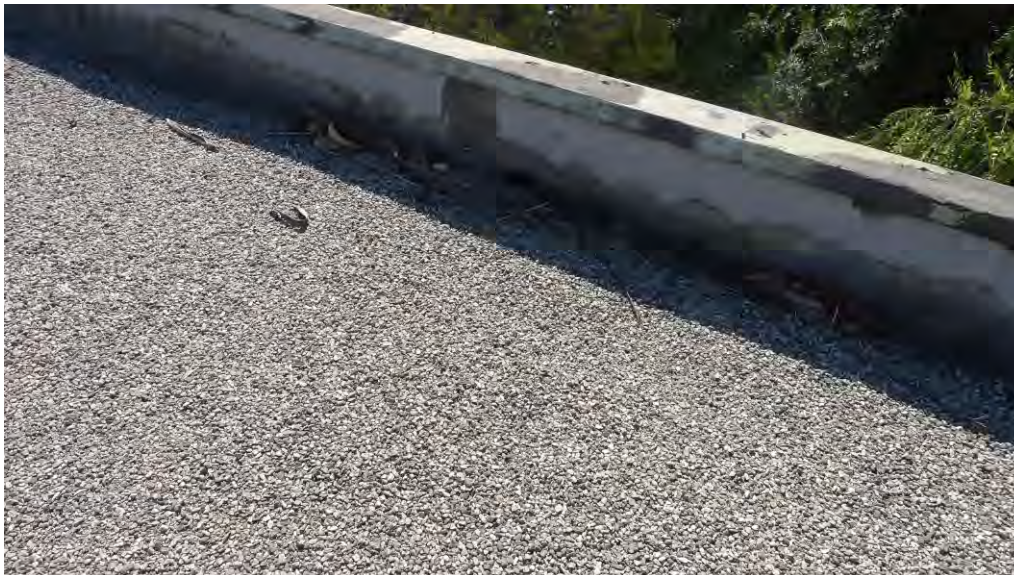
Figure 4: Debris at scuppers at multiple locations
