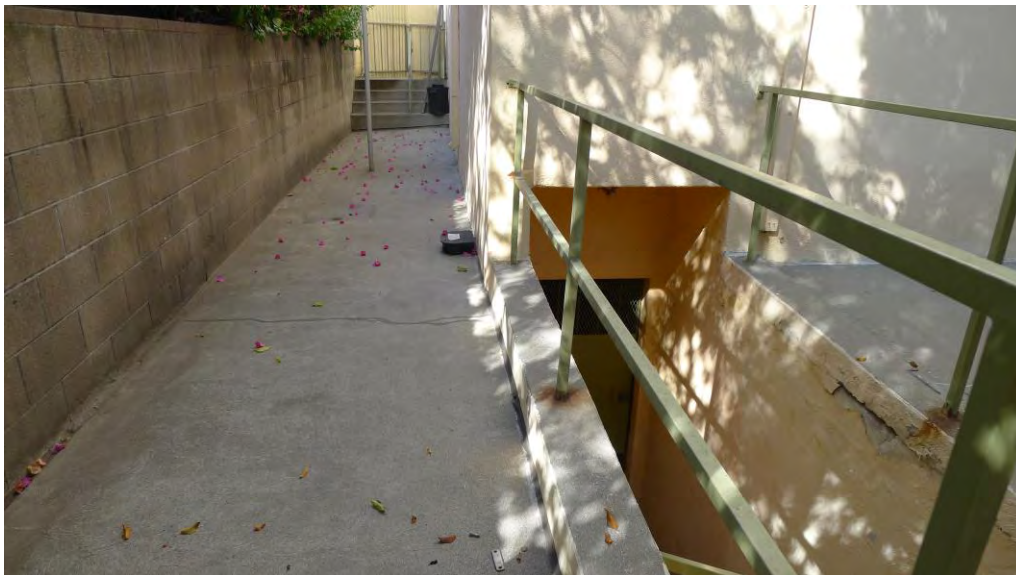
Figure 26: Rusty railing at embedment point
