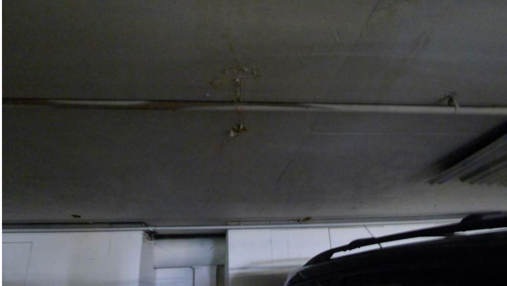
Figure 21: Water stain at concrete structural slab in garage
