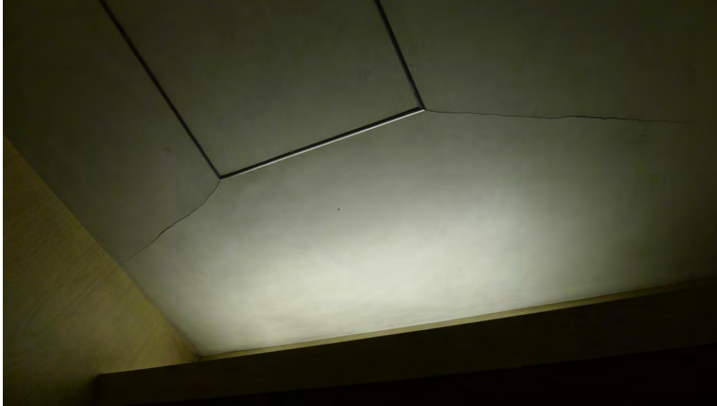
Figure 17: Cosmetic cracking in the ceiling at the common area
