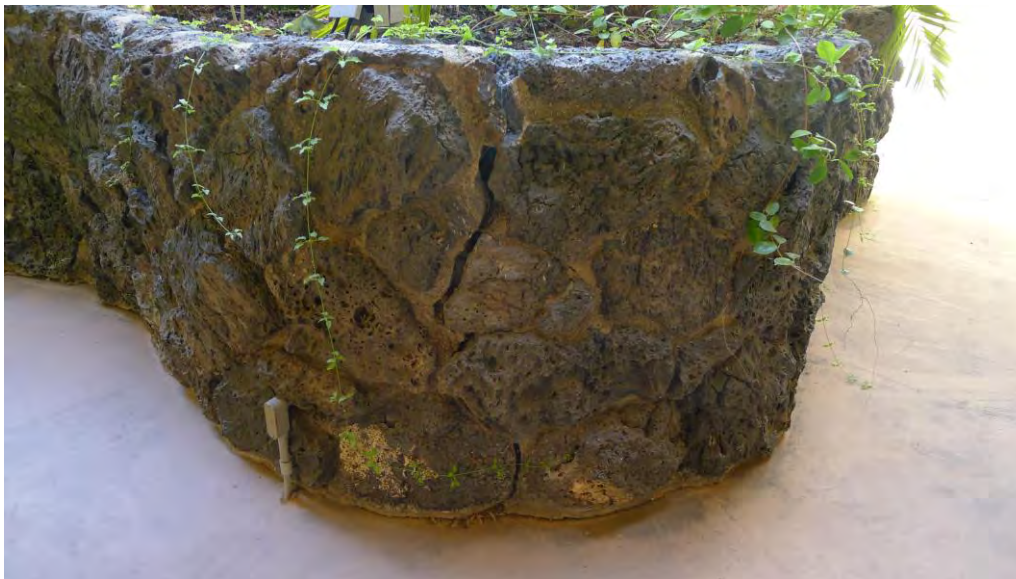
Figure 16: Large crack in planter
