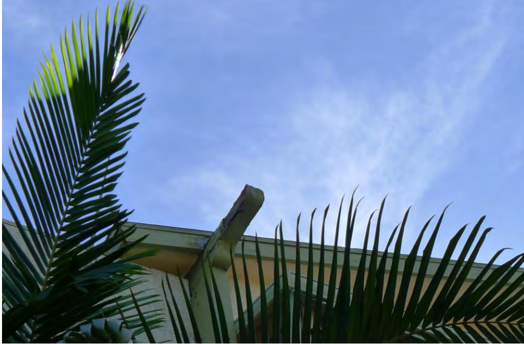
Figure 7: Paint peeling from cantilever overhang
