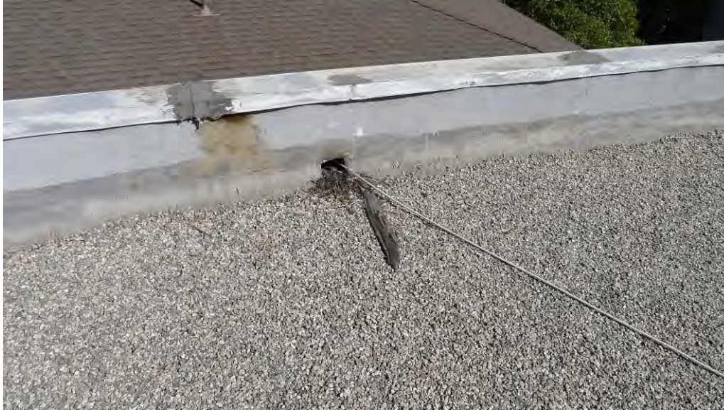
Figure 3: Roof scupper with cable and debris
