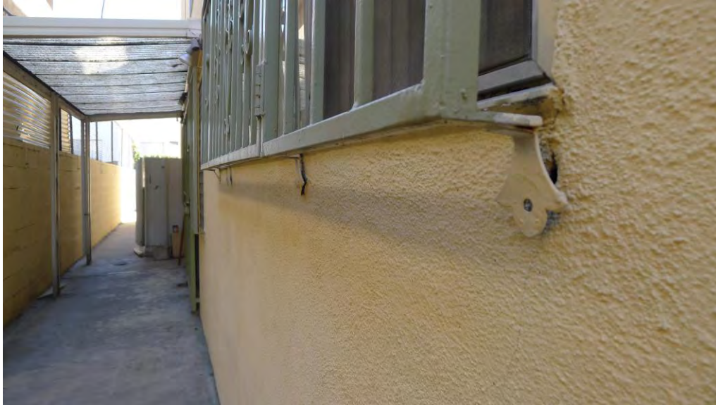
Figure 9: Missing anchorage from security bar
