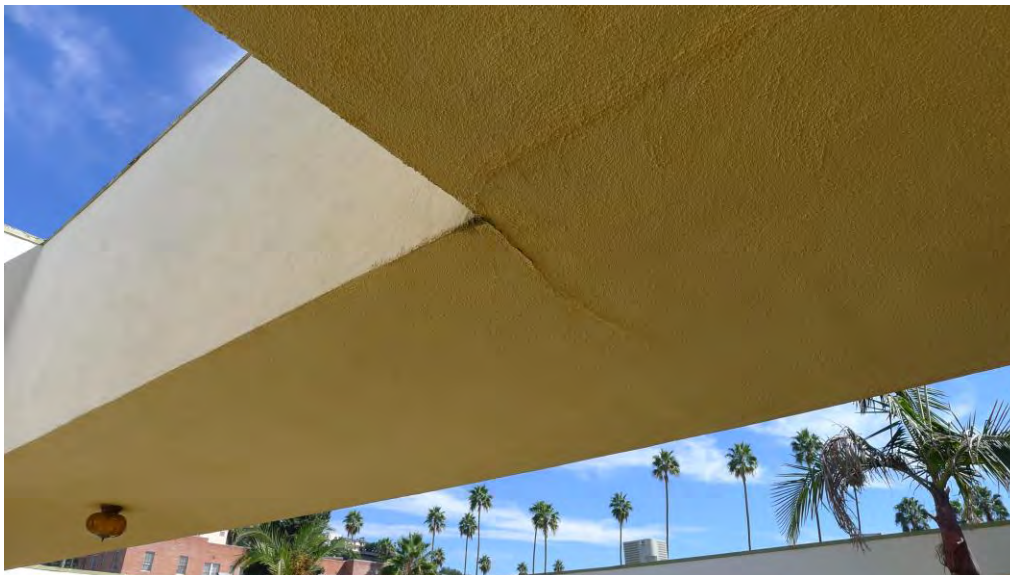
Figure 18: Cosmetic crack at walkway
