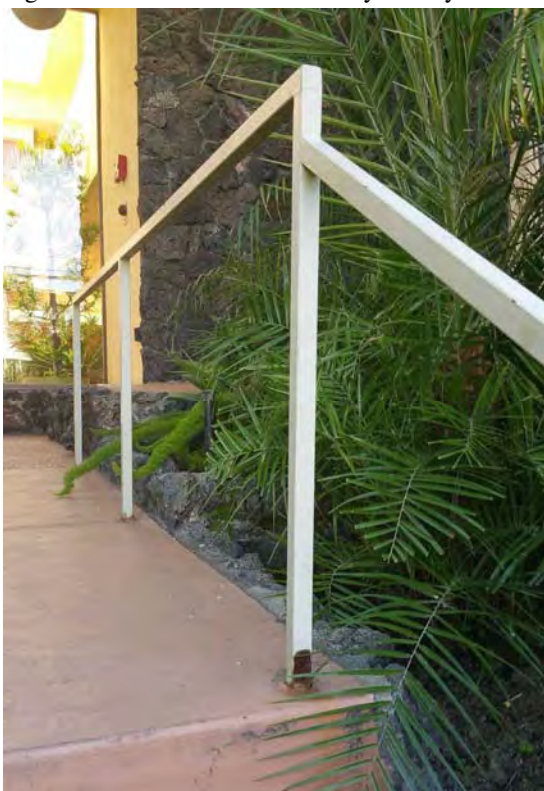
Fig. 2-11 Railing at courtyard entry with rust at base
