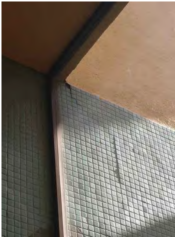
Fig. 2-9 Mosaic tile mural with crack
