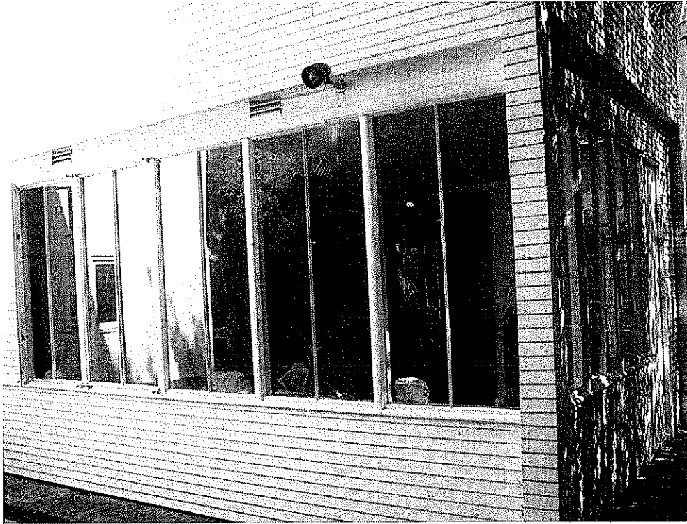
Arensberg-Stendahl Home Gallery, Richard Neutra patio addition-1933, 7065 Hillside Avenue, March 19, 2010 (Photograph by Charles J. Fisher)
