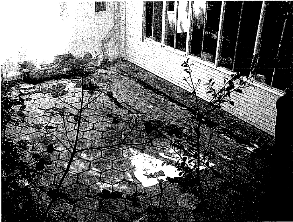
Arensberg-Stendahl Home Gallery, rear patio behind Neutra & Ain additions, 7065 Hillside Avenue, March 19, 2010 (Photograph by Charles J. Fisher)
