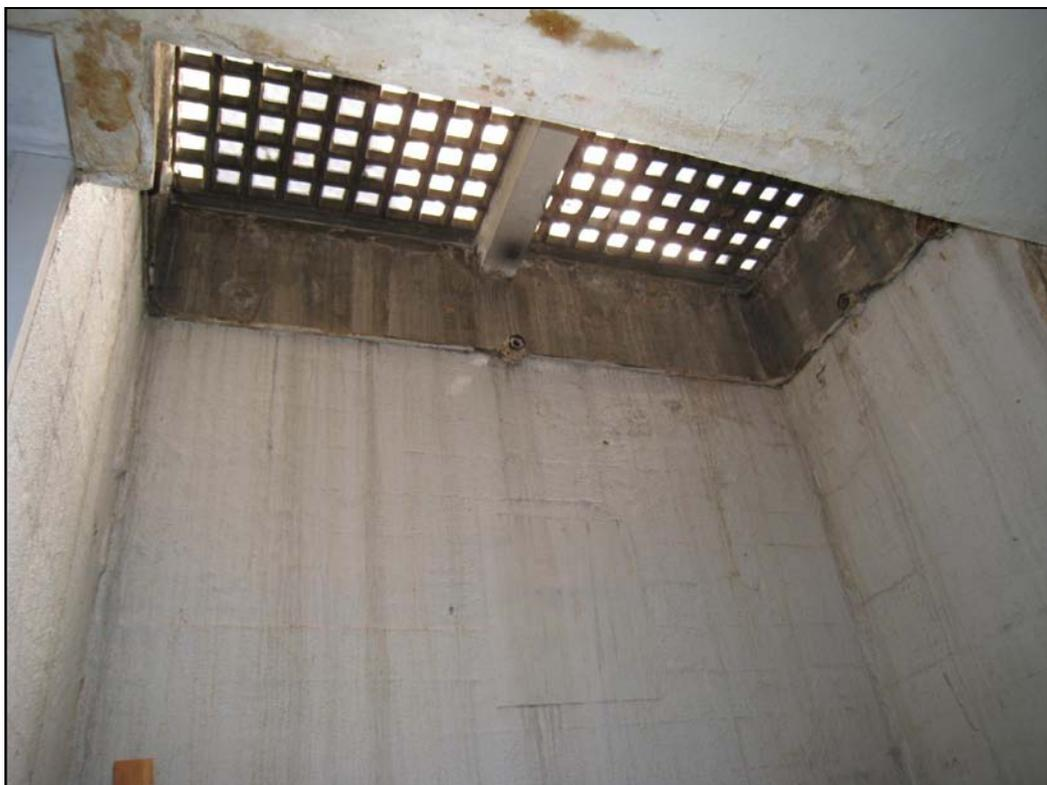
**Photograph 16:** Typical basement area showing sidewalk light. (Chattel Architecture, October 2008)
