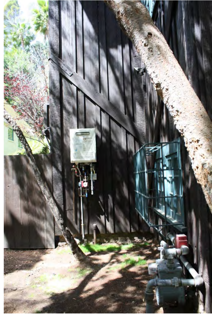
South elevation: Portion of garage and return of house; gate to main section of south elevation, view west.
