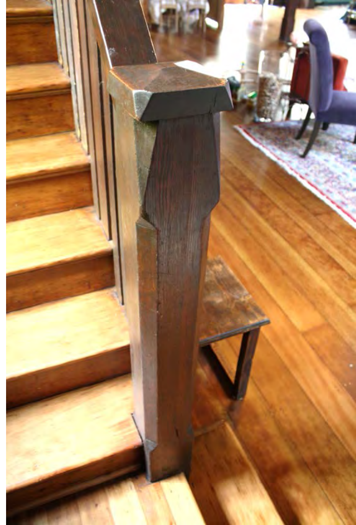
Detail: Original newel post transformed by Vreeland's design & work of the carpenter. 10" wide hardwood floor laid-in with hand hewn nails are the flooring.
