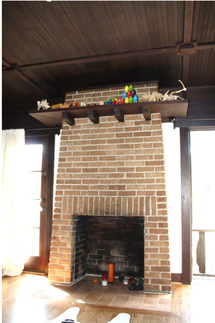
Second floor office: Original brick fireplace, tile hearth; high mantel supported by shaped brackets; doors to small balcony at either side (east closed, west open); tongue & groove ceiling with overlay of wood trim pieces topped by low pyramidal squares, view south.
