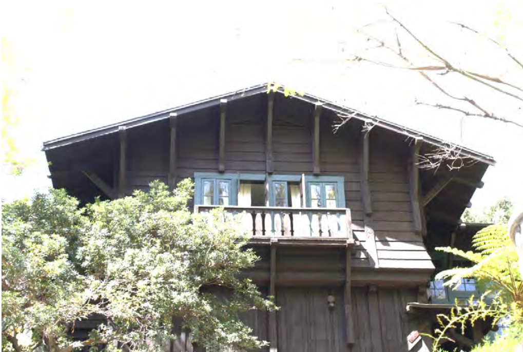
East façade beneath deep eaves: Brackets frame windows/balconette with four sets outward opening casement windows and shaped balustrades, another graduated group support balconette; second floor flares and is clad in uneven trimmed clapboards; first level clad in bat-and-board, view west.
