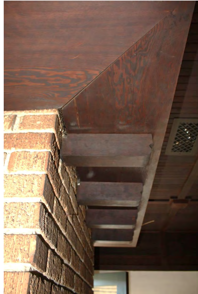
Detail: Office fireplace brick work; underside mantel with shaped brackets; tongue & groove ceiling with wood overlay topped by pyramidal squares, register.
