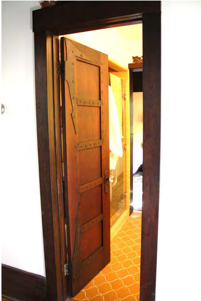
Detail: Original stock door transformed by Vreeland's design & work of the carpenter & black smith.
