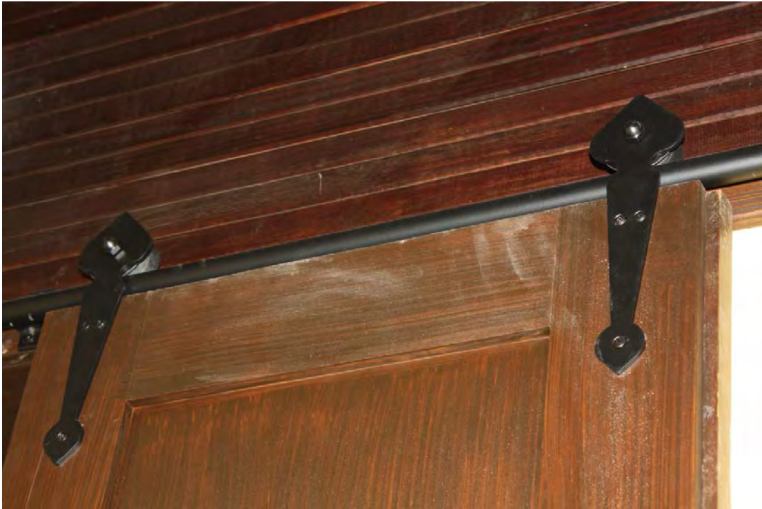
Detail, original studio level space of unknown use: Doors mounted on barn door track.
