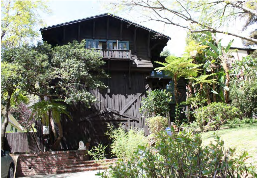
East façade: 2207 Fern Dell Place, view west.
