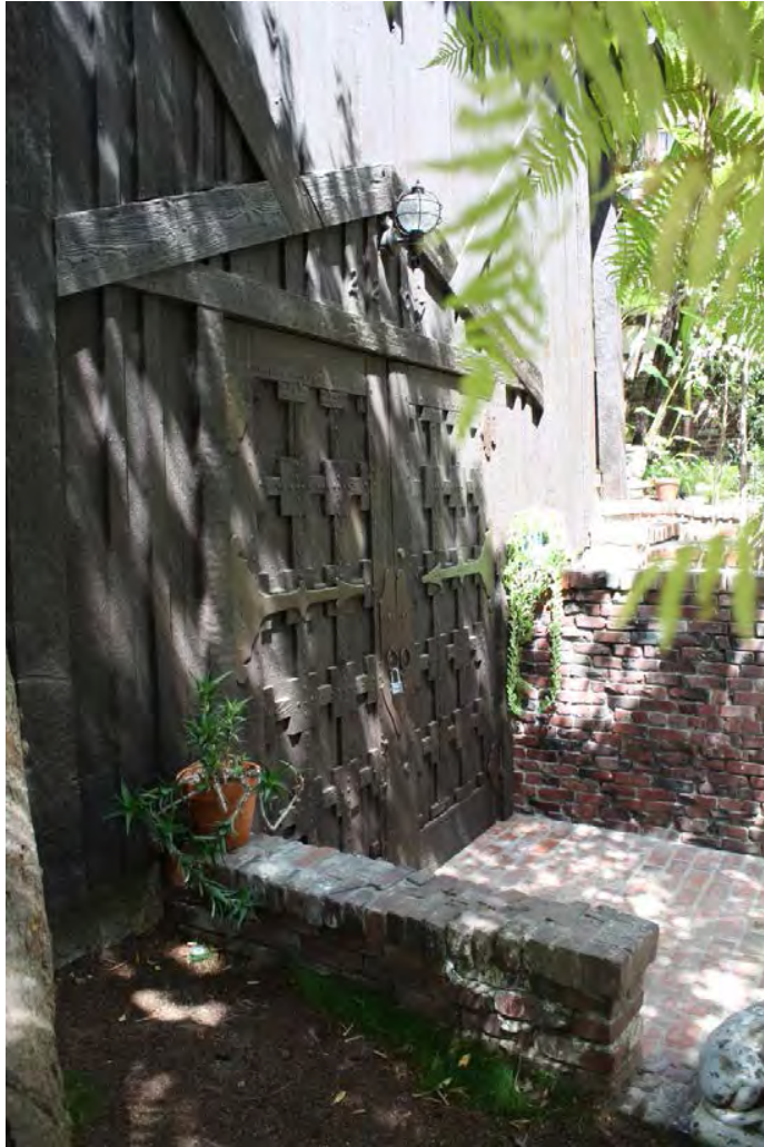
Garage Doors: Added brick walls; stock garage doors with hand-forged nail studded detail & black-smith crafted Vreeland-designed oxidized brass hinges; simple pediment above doors, view north.
