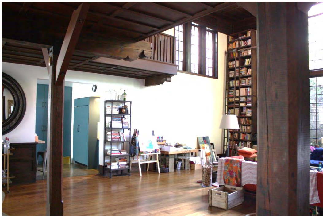
View from area now utilized as dining room: Original wrap, at west, living quarters balcony; high windows at west replace original mural/bookcase wall; original stock windows stacked in north wall, view northwest.
