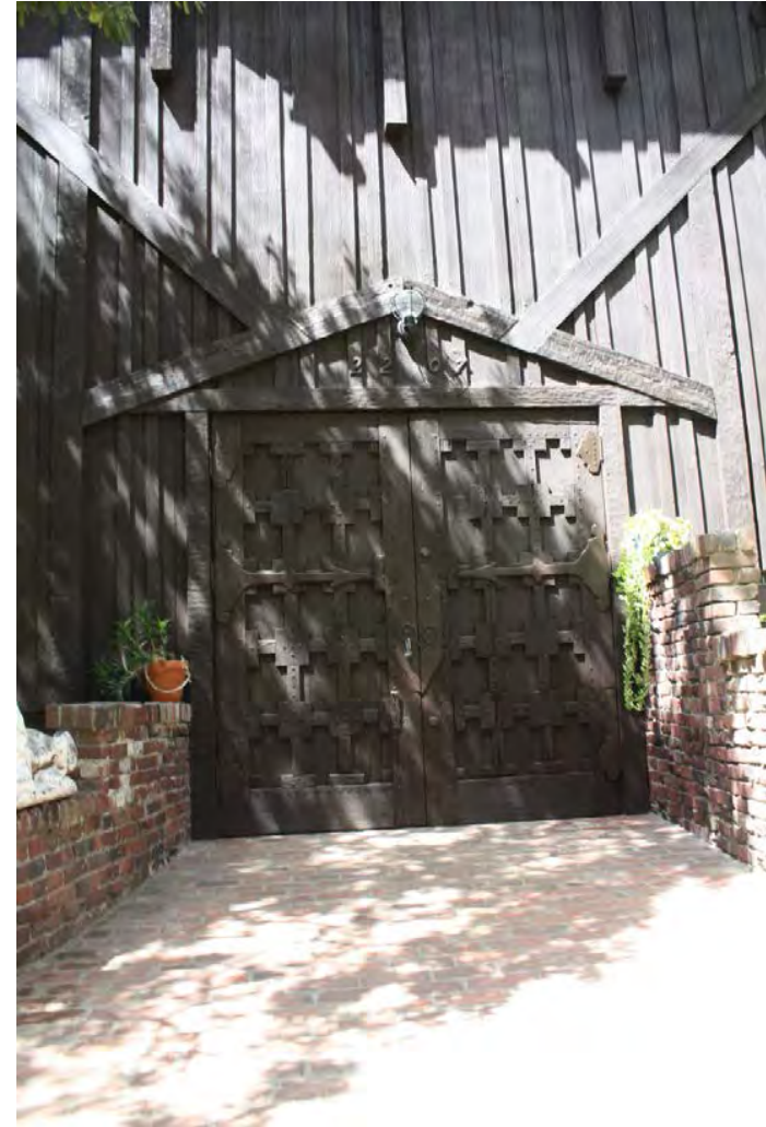
Garage Doors: Added brick walls; stock garage doors with hand-forged nail studded detail and black-smith crafted Vreeland-designed oxidized brass hinges ; simple pediment above doors, view west.
