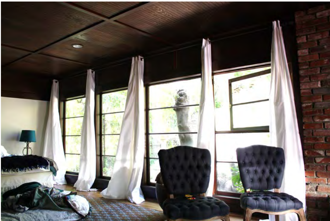
Master bedroom: Southwest corner; ribbon of sliding and one half-casement windows; ceiling/battens/frieze; beginning of fireplace, view southwest.
