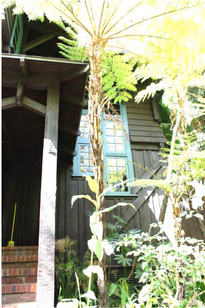
Original covered entry stairs w/ bracketed eaves: Vertical bat & board cladding at first level with stacked stock windows along interior stairs; flared second level ripple edge clapboard cladding, view west.
