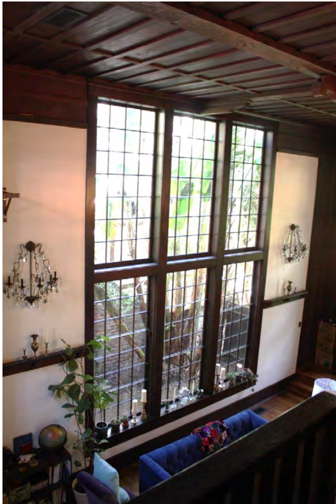
Original stacked stock windows at north wall provide natural North light to Vreeland, 12" board ceiling with battens, shelves at either side of windows, 10" lumber floor laid with hand forged nails, view northeast.
