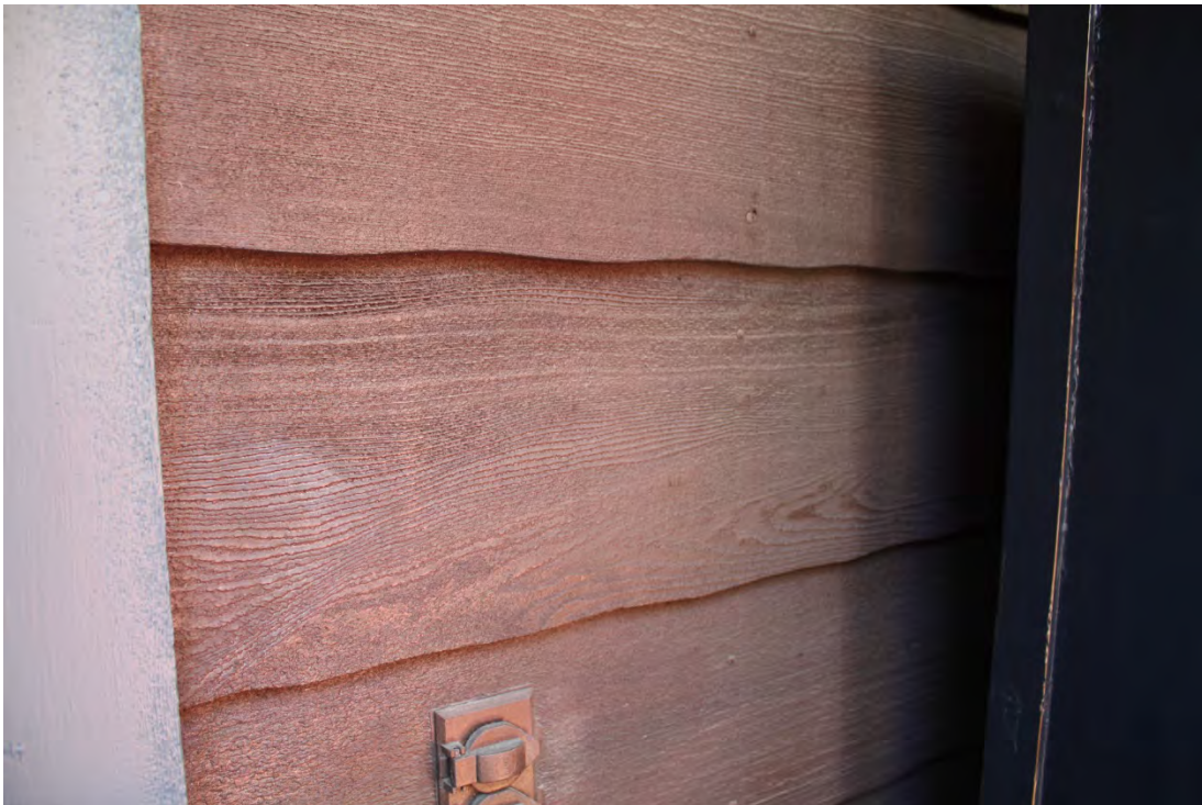
Original detail: Hand adzed clapboard cladding at second level.
