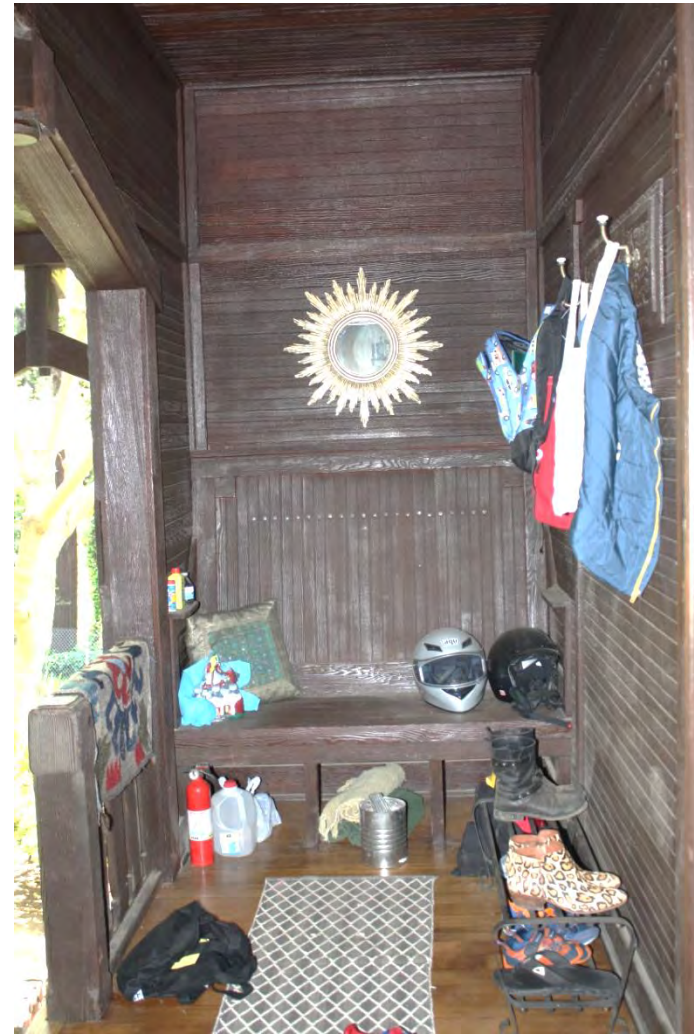
Raised entry porch: North porch balustrade; east tongue & groove wall, built-in seat of vertical tongue & groove studded w/ hand-forged nails; south tongue & groove wall; hardwood floor, view east.
