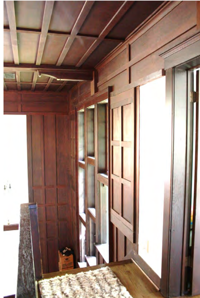
East wrap of original living-rooms/balcony, top of stairs connecting living level to double level studio: Ceiling frieze, decorative bracket; north wall at background; east wall stacked stock windows paneling, frieze, view north.
