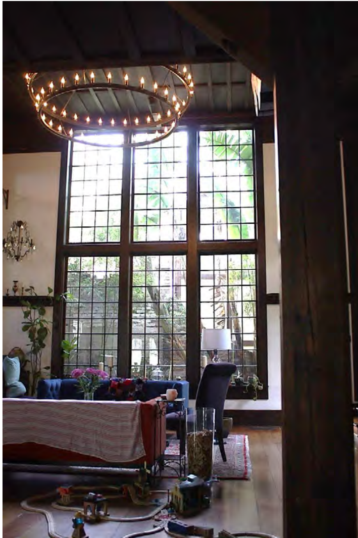
Double height original studio: North stock stacked windows; ceiling with 1 x 3" batten overlay; wood shelves at either side, view north.
