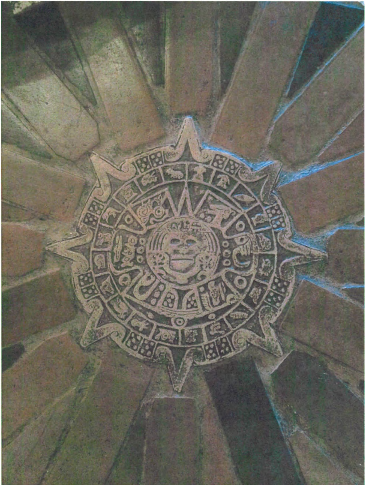
Casa de Mi Sueño, tiles laid by Sophie in front entry, 3820 San Rafael Ave, Aug 30, 2013 (photograph by Peter Luttrell)
