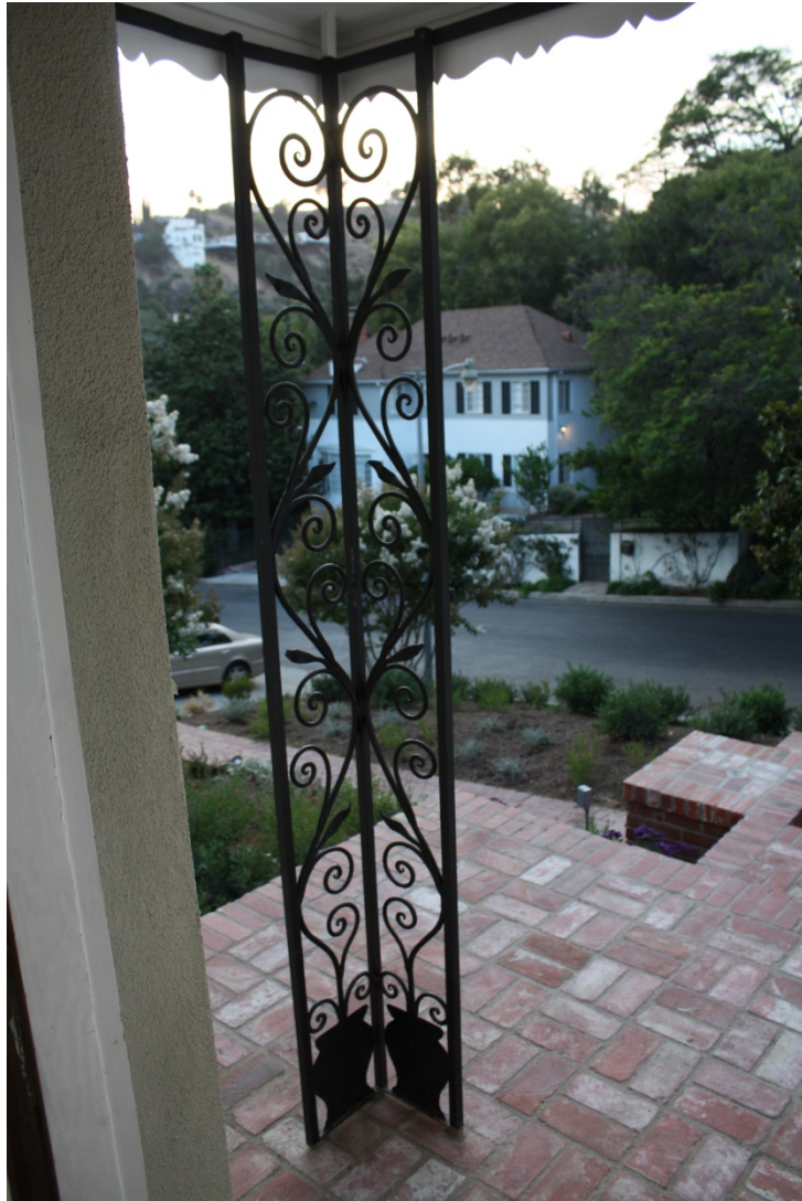
Original, restored open-work potted plant corner piece and supports for scalloped porch awning, view northwest across brick porch, steps and walkway.
