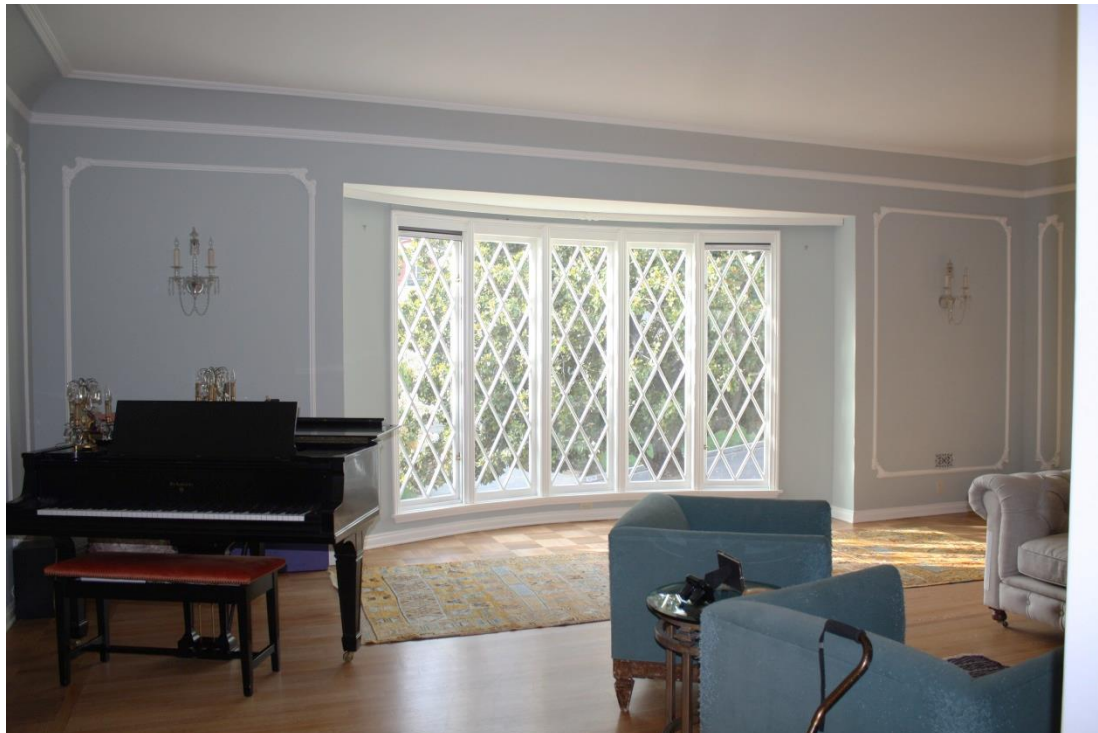
Original sunken living room: North wall restored diamond pane curved bay window; Restored parquet and regular flooring, restored sconces, view northeast.
