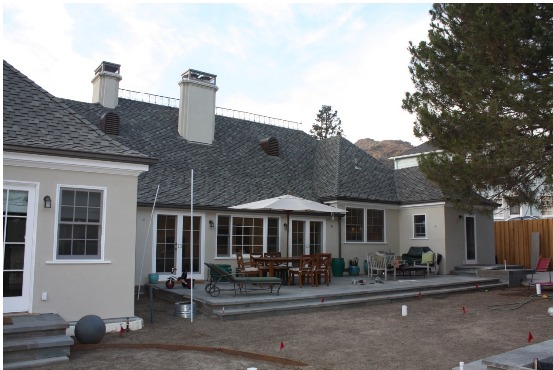
South elevation of residence: Master bedroom, sun room, kitchen, laundry. Original chimney forms, metal vents, original faux widow's walk; replaced roof, view northeast.
