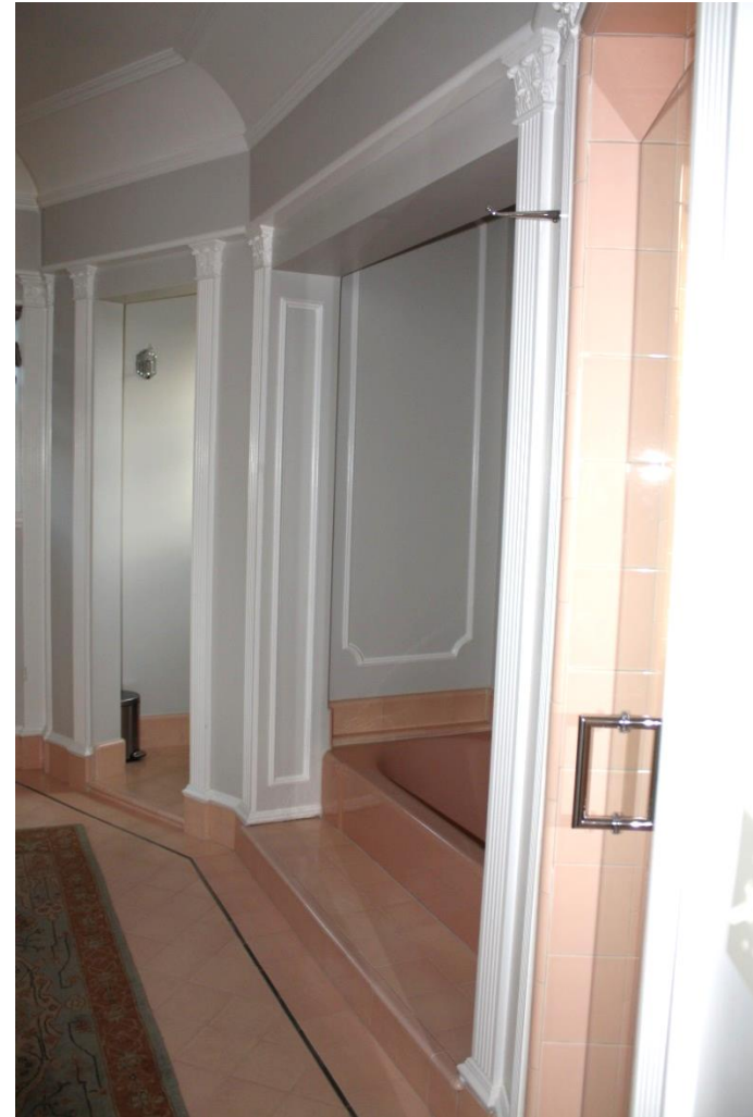
Original master bathroom: West wall water closet; step up to sunken tub inset in paneling outlines and fronted by stylized Corinthian piers; original handle of shower stall, diagonal tile floor, inset aluminum, square set tile border, view south.
