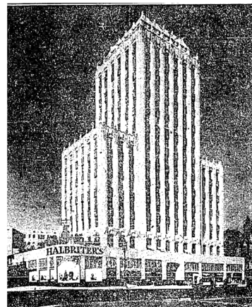
One More Big Branch Establishment of pioneer Los Angeles mercantile firm was added to the long list now located on Wilshire Boulevard with the opening yesterday of Halbriters', Inc., new store in the Wilshire Professional Building at St. Andrews Place.
