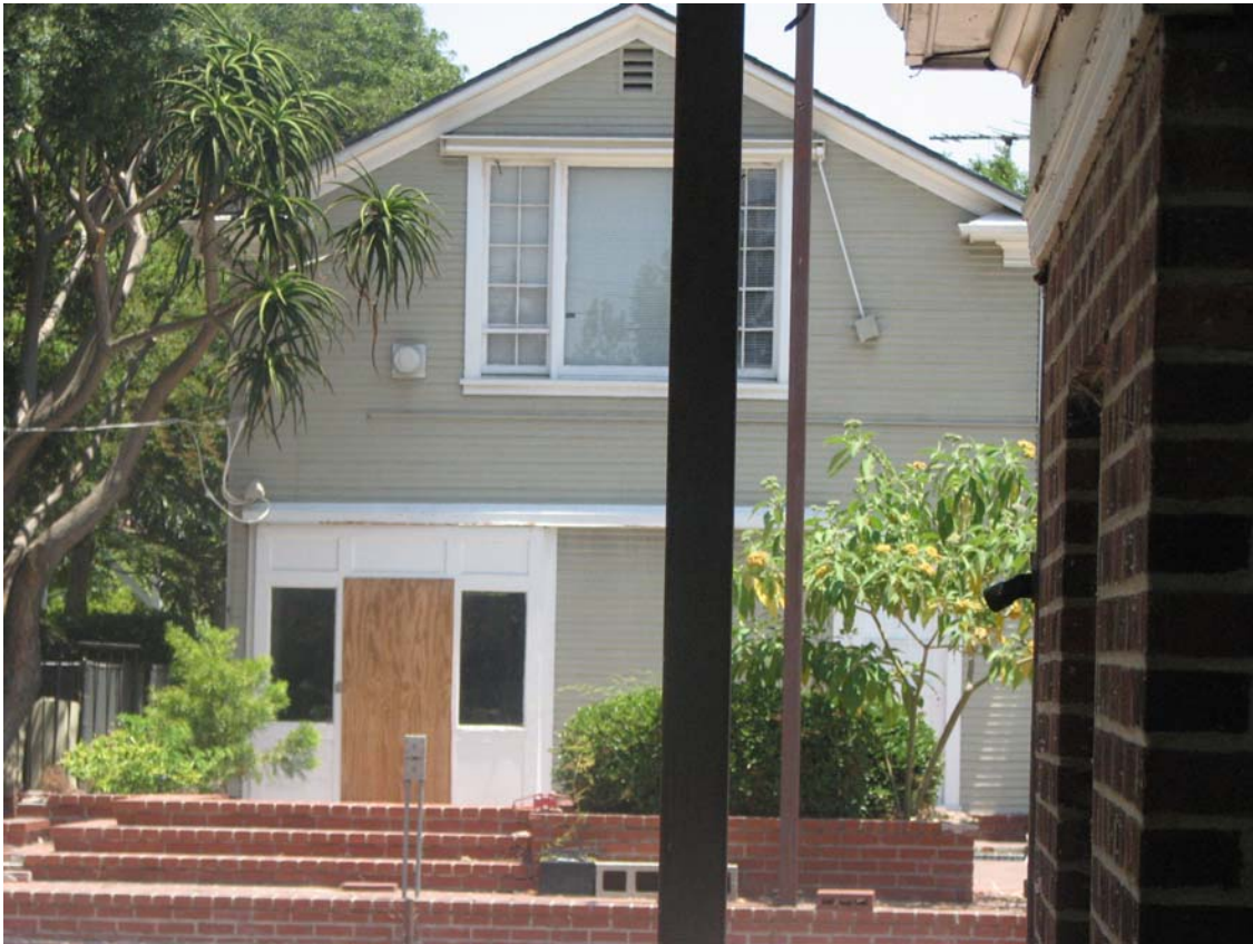
Heerman Estate, rear elevation, 525 S Van Ness Avenue (Photograph by Charles J. Fisher)
