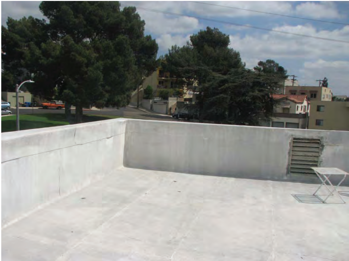
Restovich House, rooftop, 1001 Everett Street, September 19, 2014 (Photograph by Charles J Fisher)
