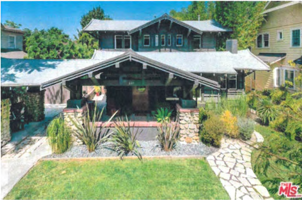
East façade at time of purchase.
