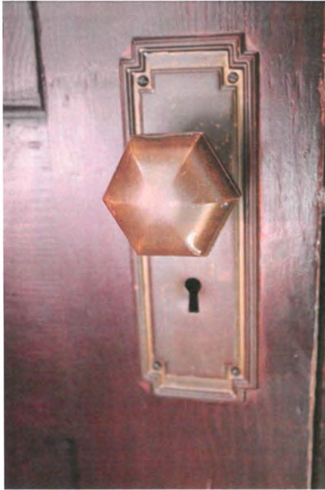
Detail: Original escutcheon & door knob used throughout.
