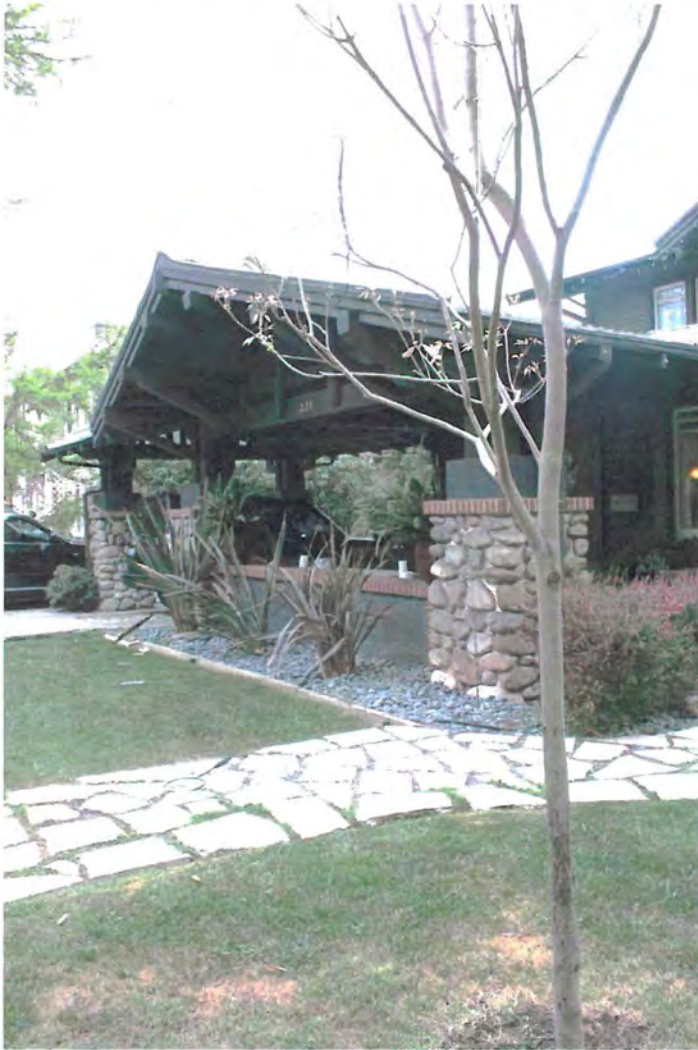
Porch of residence: View southwest.
