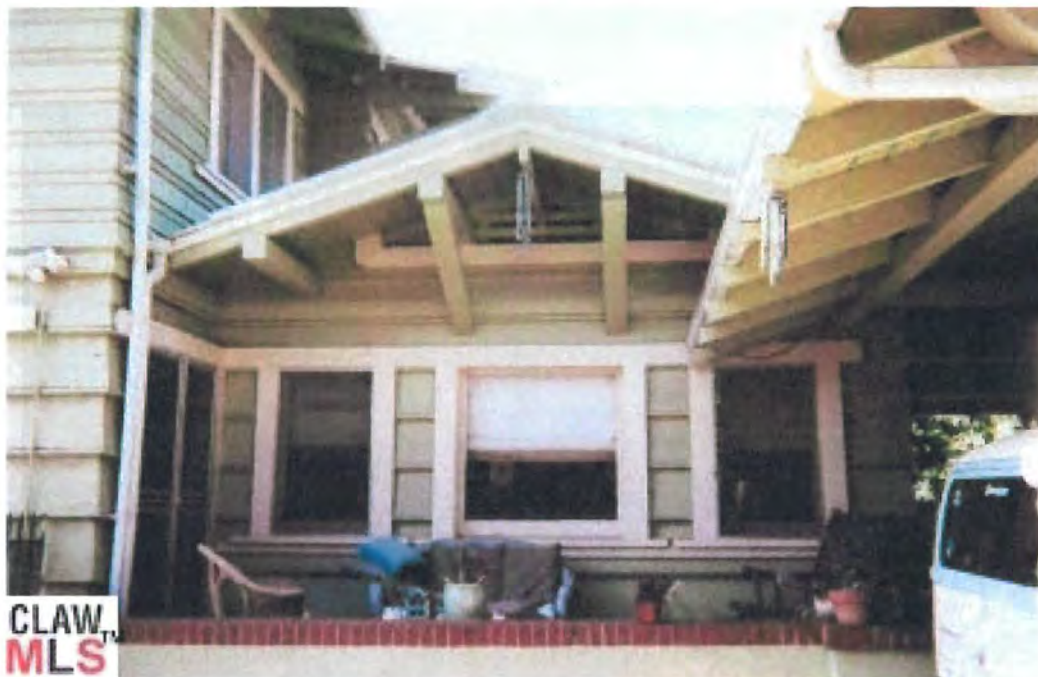
South porch with Oriental beam influence and eaves of porte-cochere, "before" photographs of previous owner's rehabilitation.
