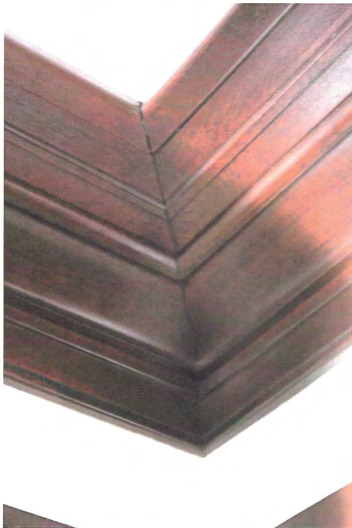
Detail: Corner of dining room ceiling molding.
