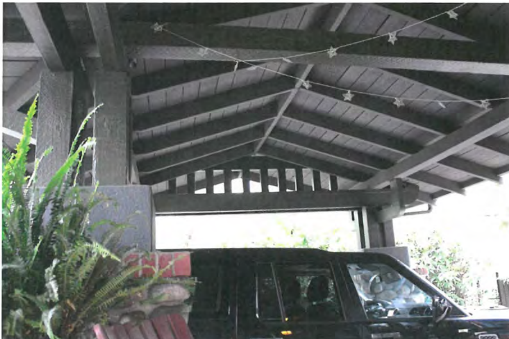
Gabled porte-cochere: Intersection of porch roof gable with porte-cochere gable above brick pier and beam upright support, view south.
