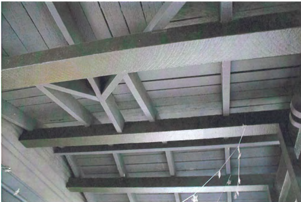
Detail: Beam work beneath porch roof.
