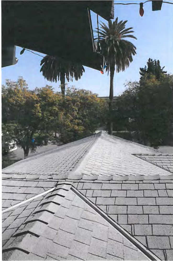
Detail: Craftsman Airplane bungalow roofs: View east from master bedroom, along first floor central ridge, beneath second floor deep eaves.
