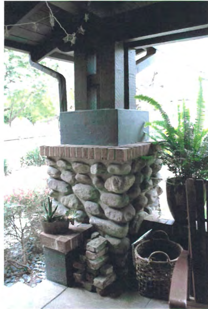
Pier at north end raised porch: Field stones set in concrete form base of pier, topped by cement square with four posts create vertical support for porch roof, the whole set in a low concrete wall w/ brick topper, view northeast.
