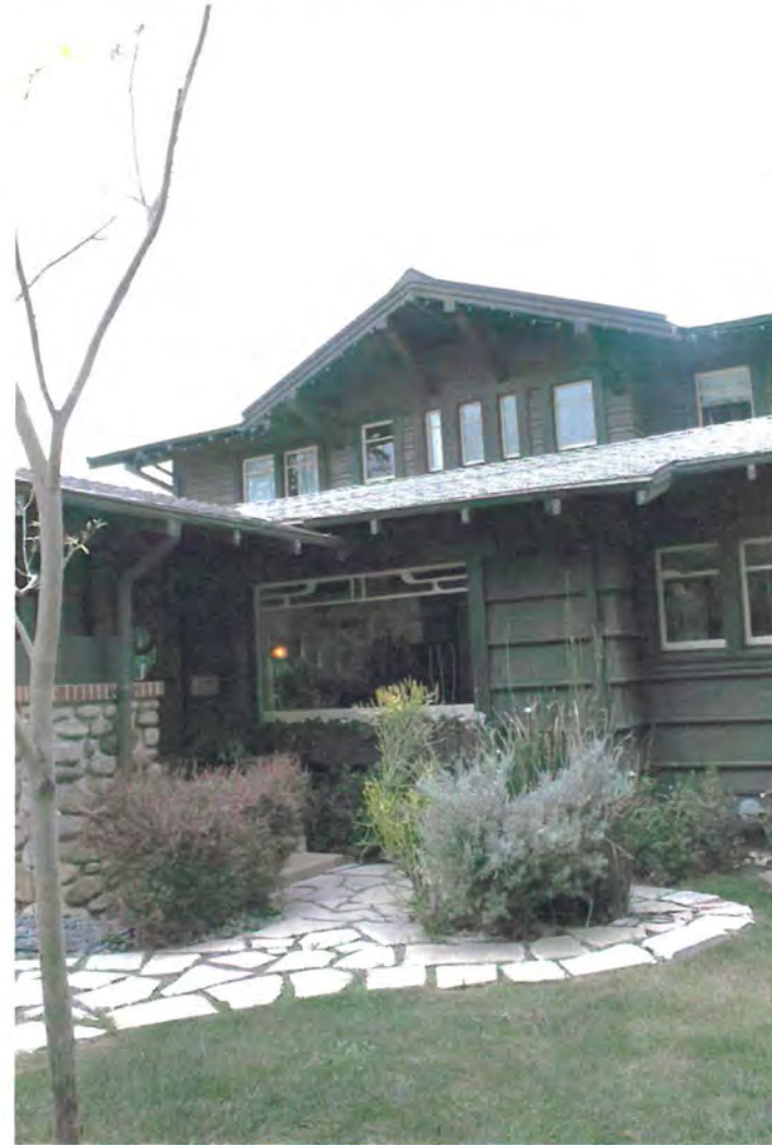
First and second story of residence with Oriental influence large single-pane window of living room: View southwest.
