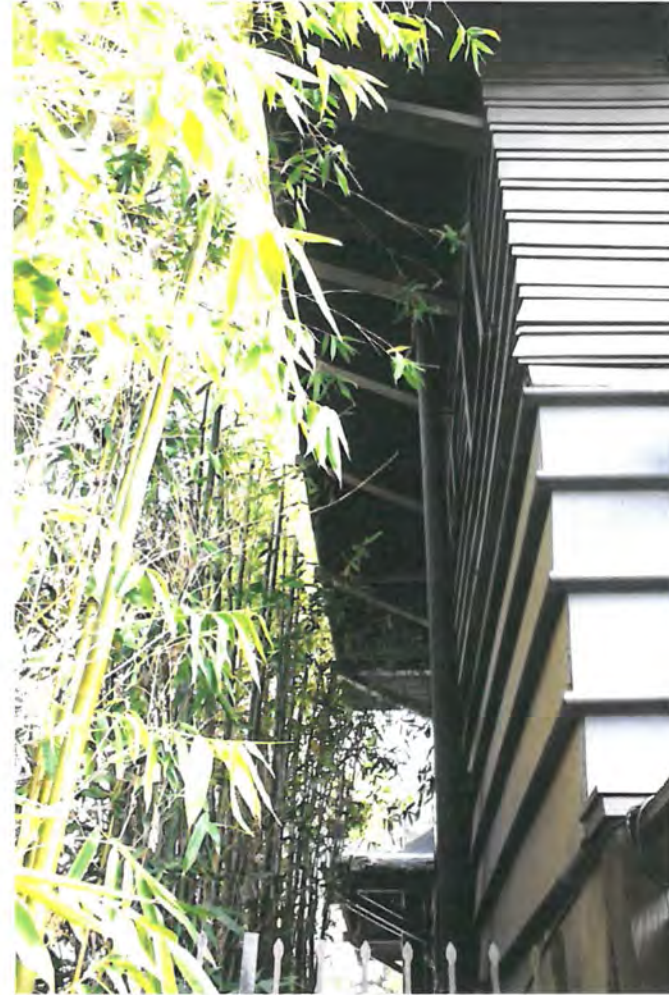
North elevation of residence: Brackets beneath deep eaves; differing types of siding clad first and second floor elevations. View east.
