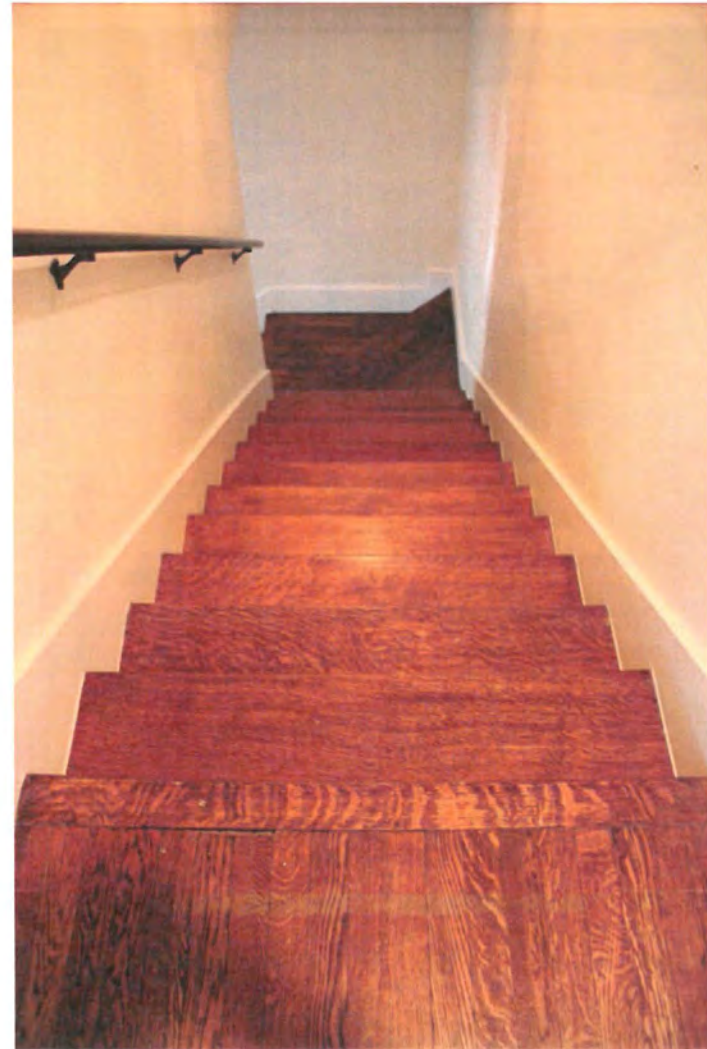
Stairs: Behind living room wall, view east from second floor.
