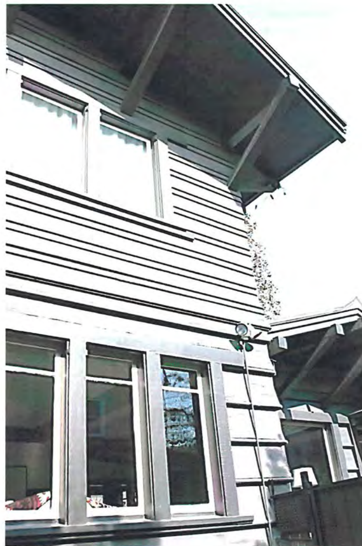
Detail: South elevation. Note variation in second and first story siding, view northeast.
