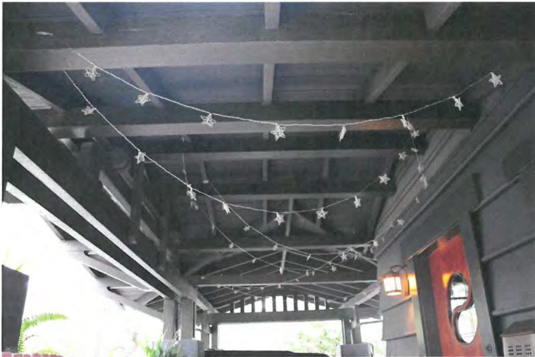
Porch: From beneath, to the south, past original entry door to intersection of gables of north/south porch, porte-cochere, east/west side porch, view south.
