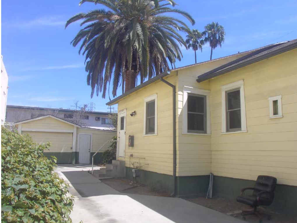
12. Rear elevation and garage. View: Northeast
