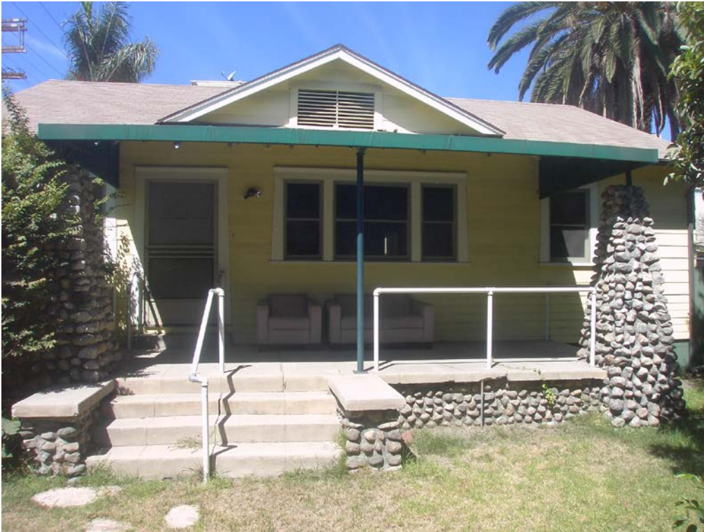
1. Front (East) elevation. View: West
