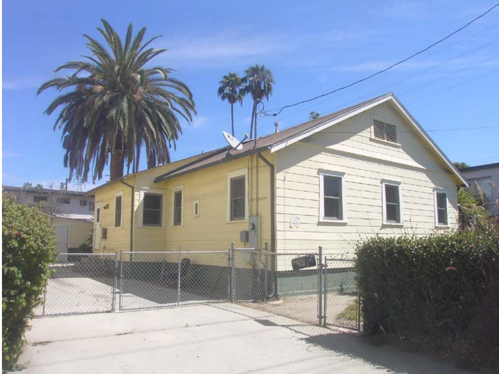
10. Rear and south elevations. View Northeast
