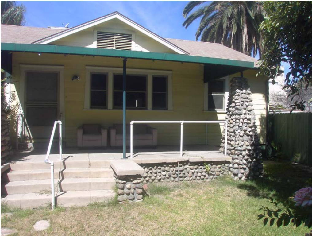
3. Front (East) elevation. View: West
