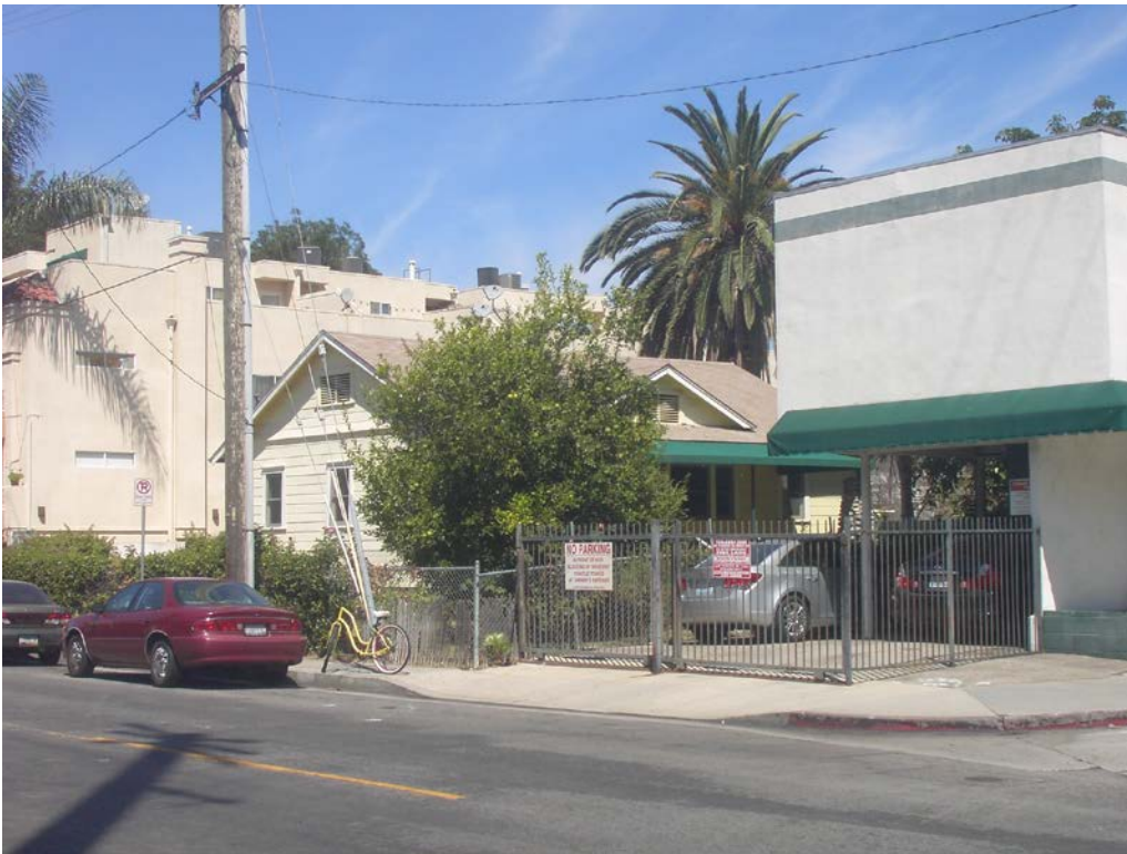
2. Front and south elevations. View: Northwest
