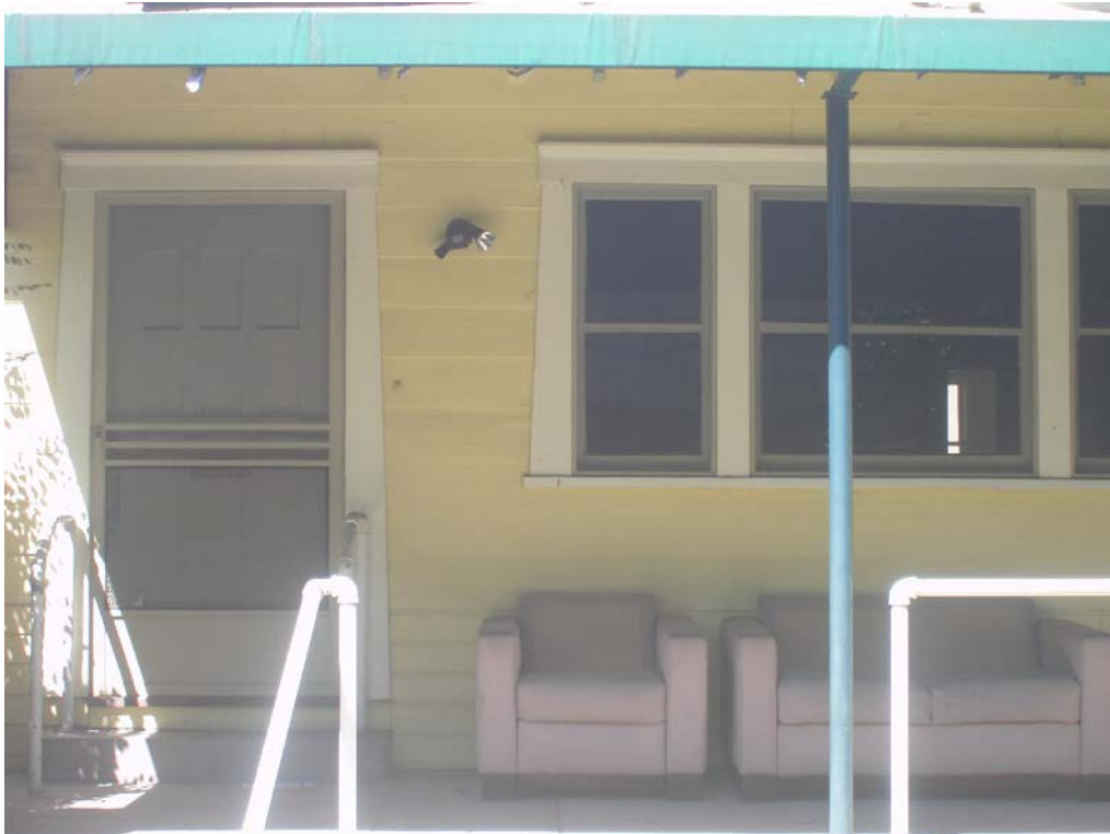
6. Front elevation, entrance and porch detail. View: West
