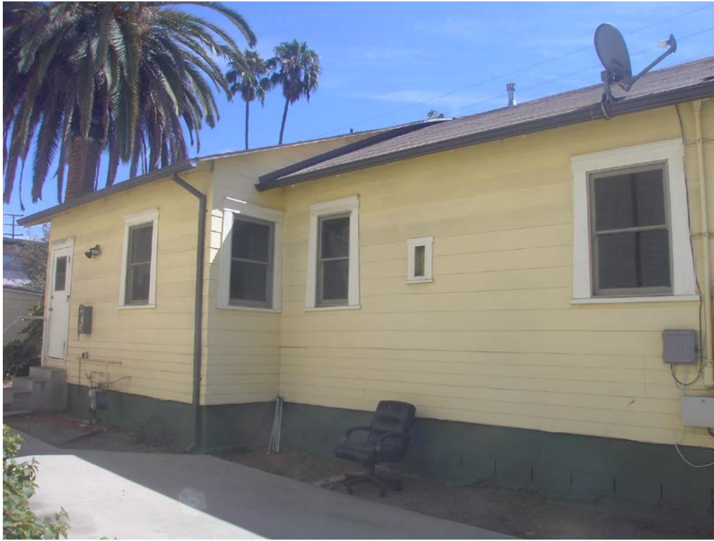
11. Rear and south elevations. View: Northeast
