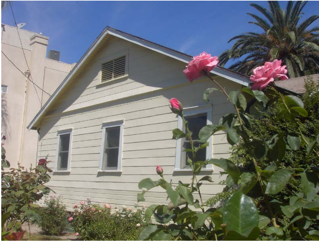
9. South elevation. View: Northwest
