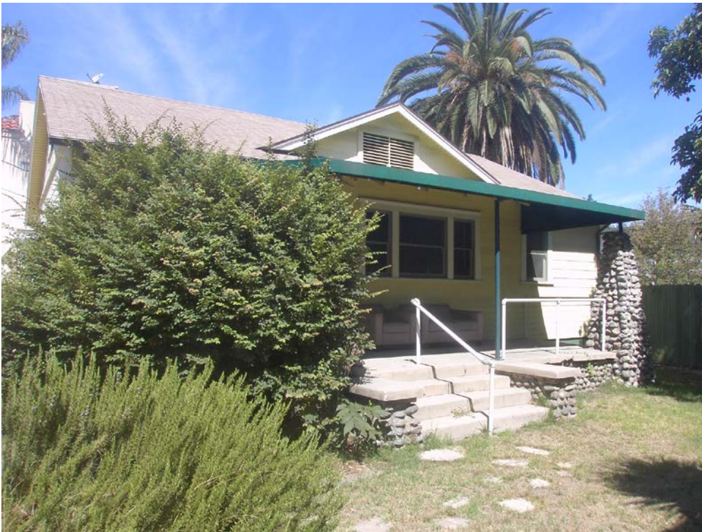
4. Front (East) elevation. View: Northwest
