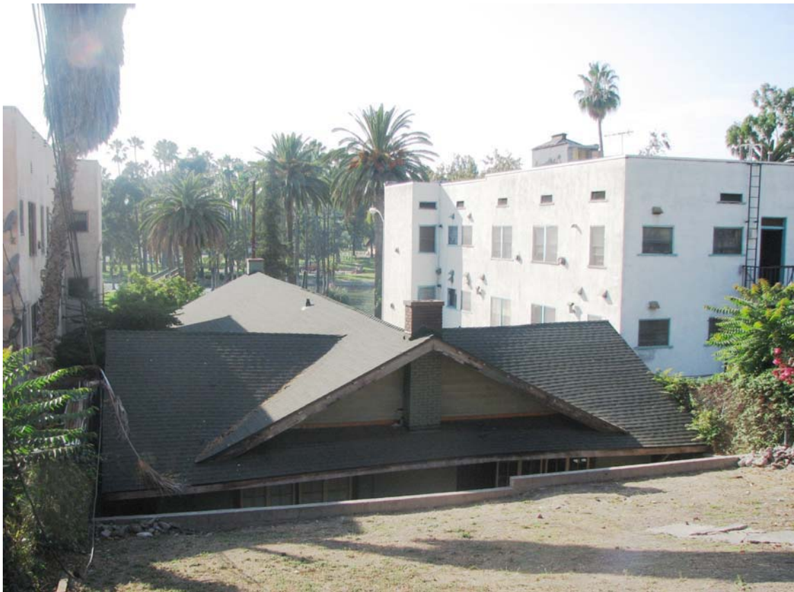
Original Echo Park Clubhouse, roof from rear, 1004 Echo Park Avenue (Photograph by Charles J. Fisher)
