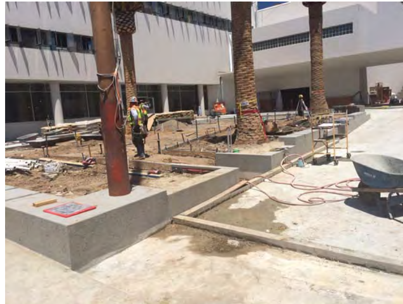
Detail of plaque after installation in courtyard (June 2015).
