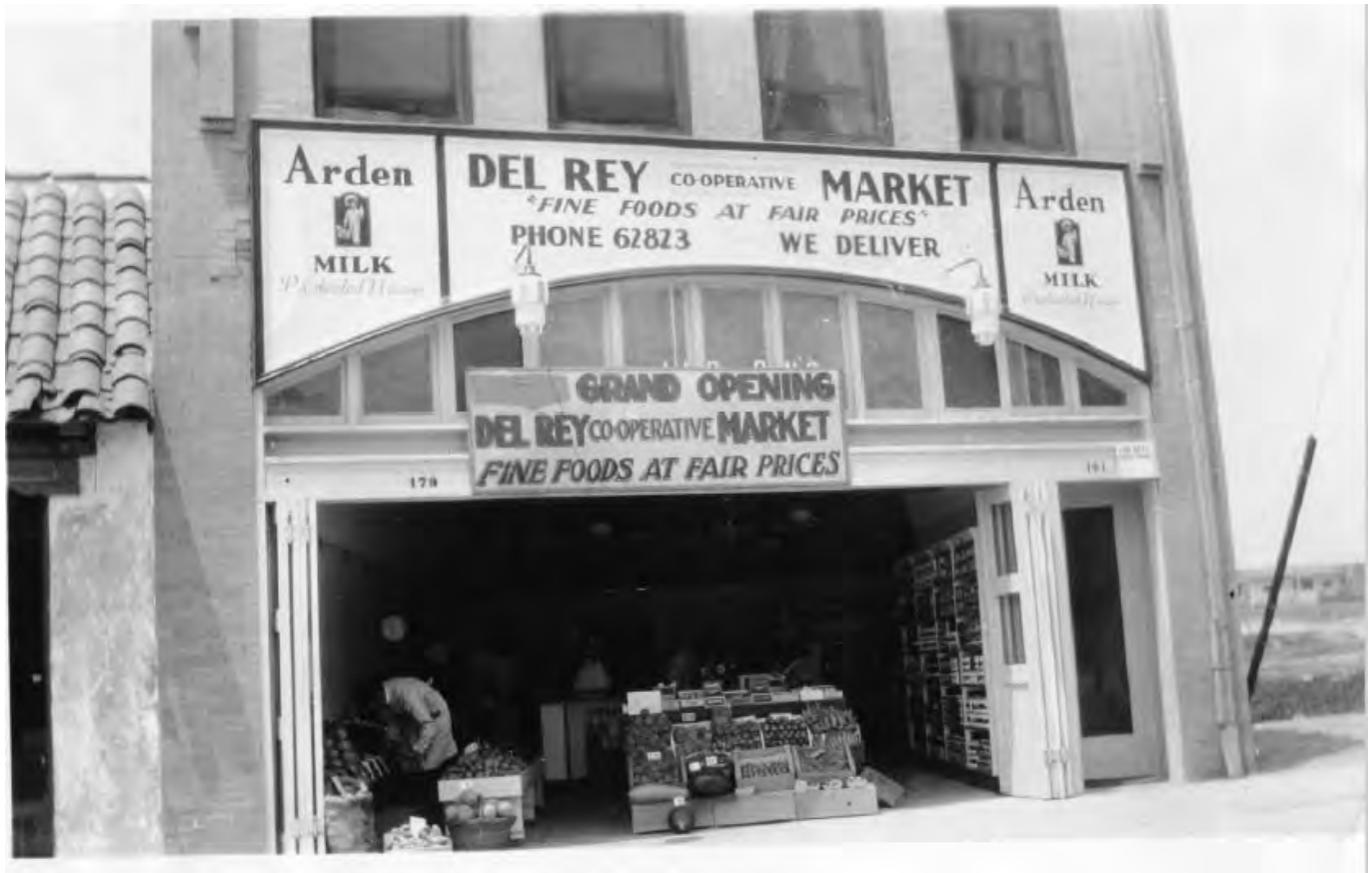
Figure 16. Del Rey Co-Operative Market circa early 1930s, showing market signage, two exterior light fixtures, and open wood storefront with folding doors (all removed)(Fowler, T.O. McCoy's Playa del Rey , 46)
