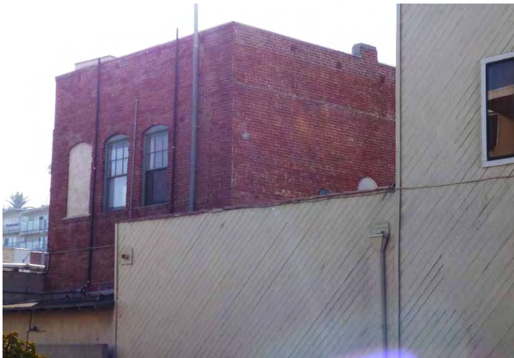
Figure 28. Rear (north) elevation, partially obstructed, view southeast (PCR 2015)
