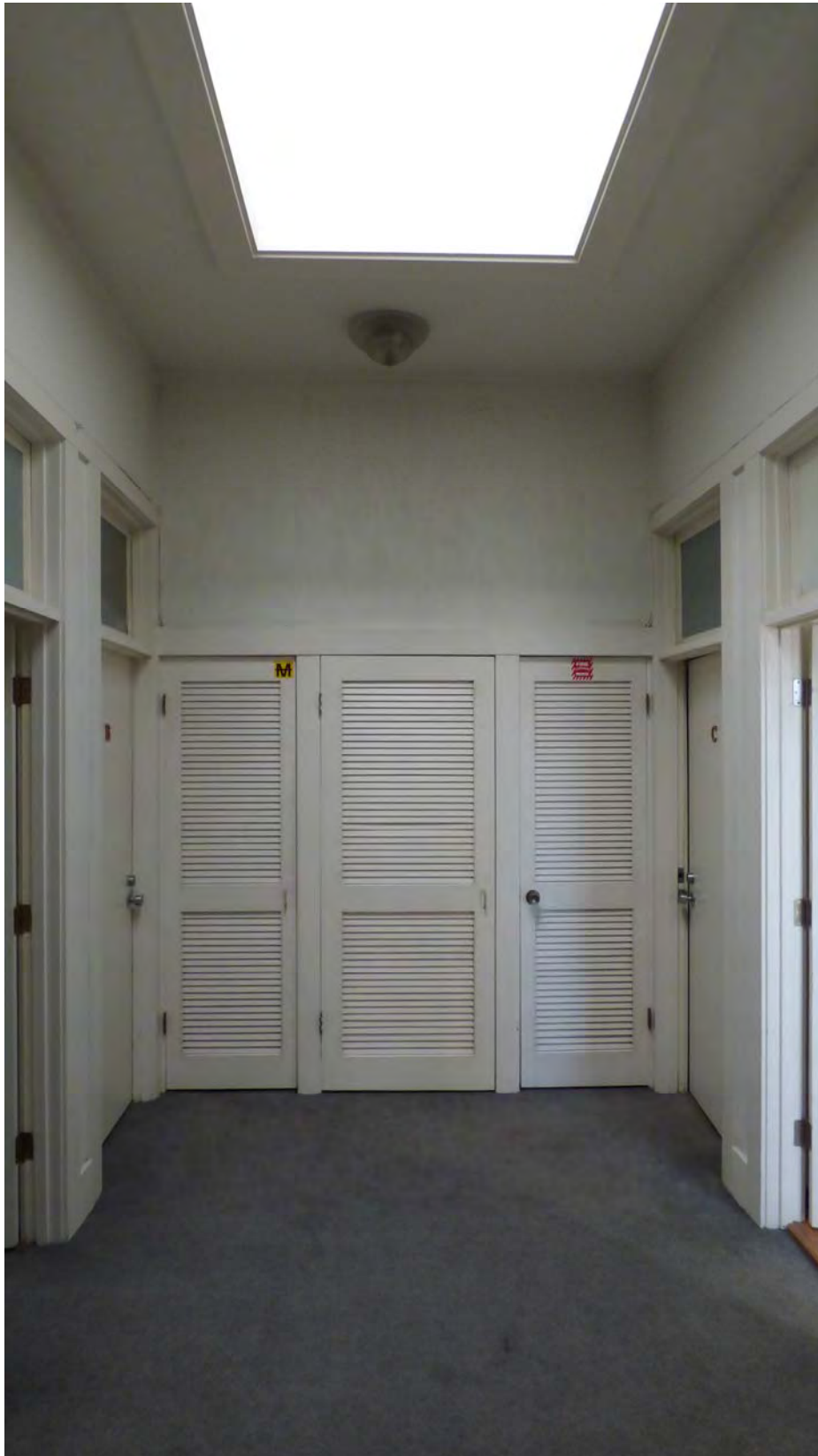
Figure 41. Second floor interior hallway, showing closet storage (center, alteration) with doors to individual units on either side (doors replaced), view east (PCR 2015)
