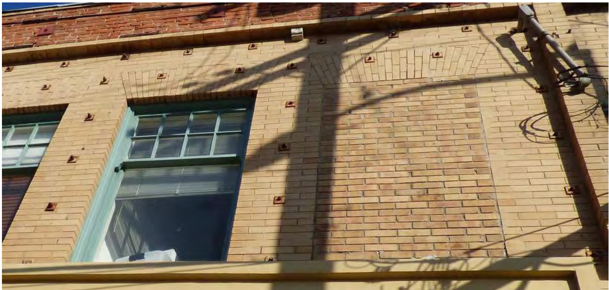
Figure 22. At left, an original wood frame double-hung sash window, and at right, an original window opening that has been infilled with brick (PCR 2015)
