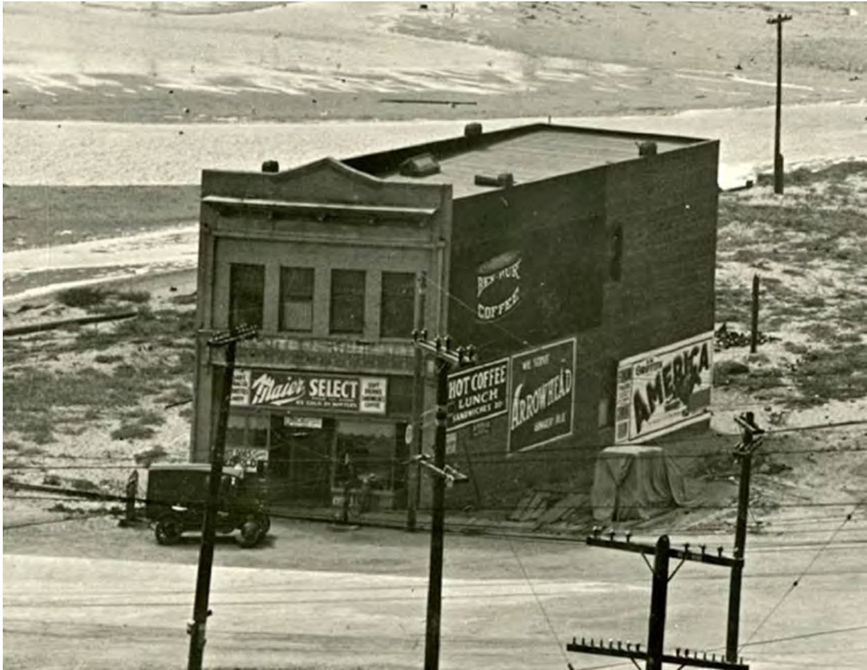
Figure 15. Subject property as it appeared circa 1920s, at which time it appears (based upon the signage) to have been used as a restaurant (McMahon, Historic-Cultural Monument Application, Playa del Rey Commerce Building, original provenance unknown)
