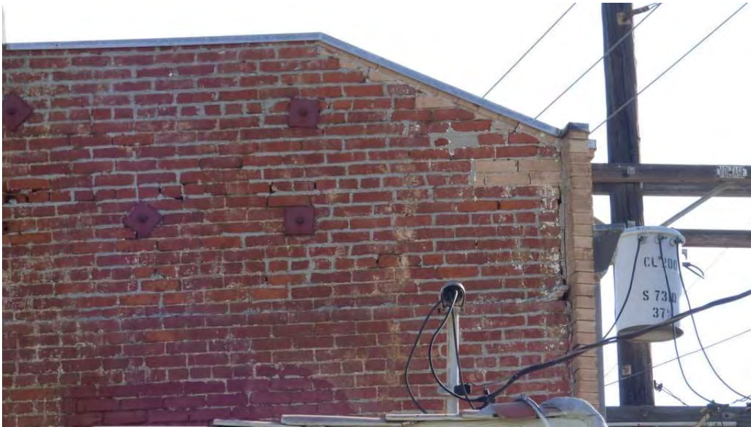
Figure 31. Detail of west elevation showing beveled corner (alteration) (PCR 2015)
