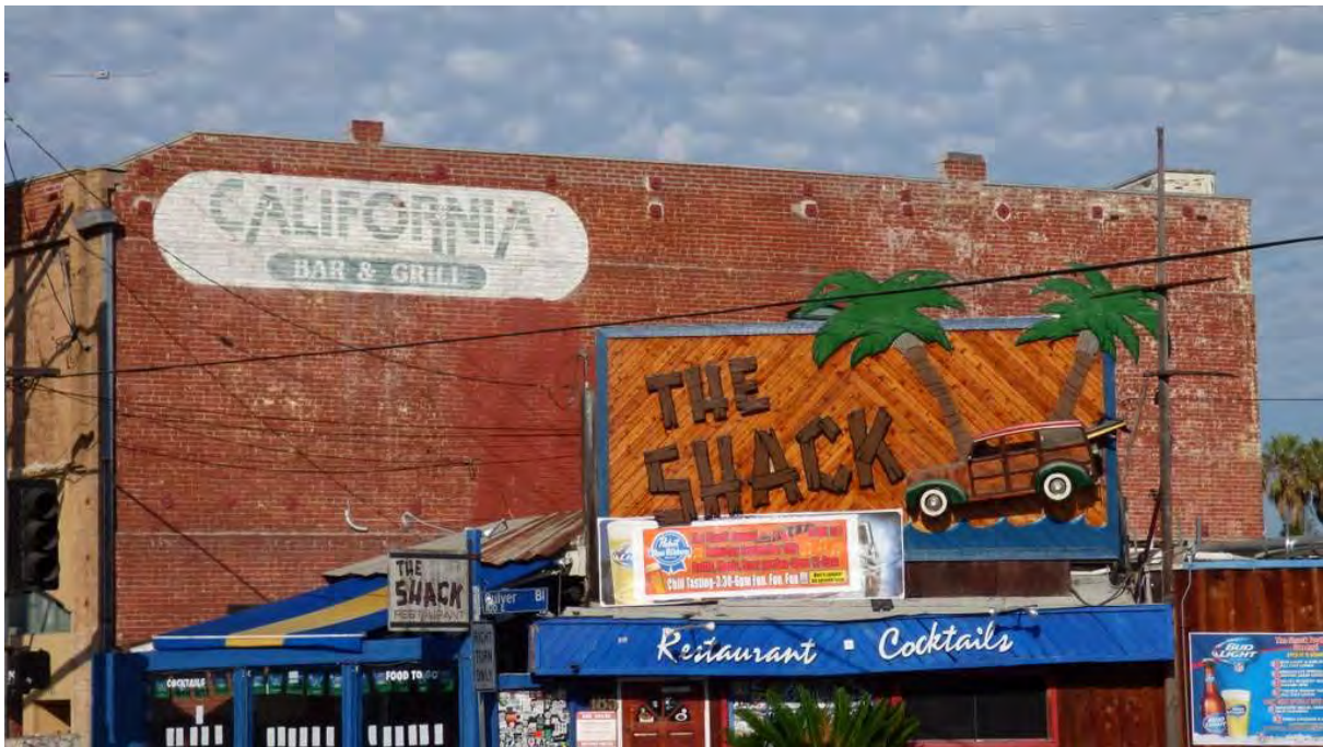
Figure 25. East elevation, view west (PCR 2015)
