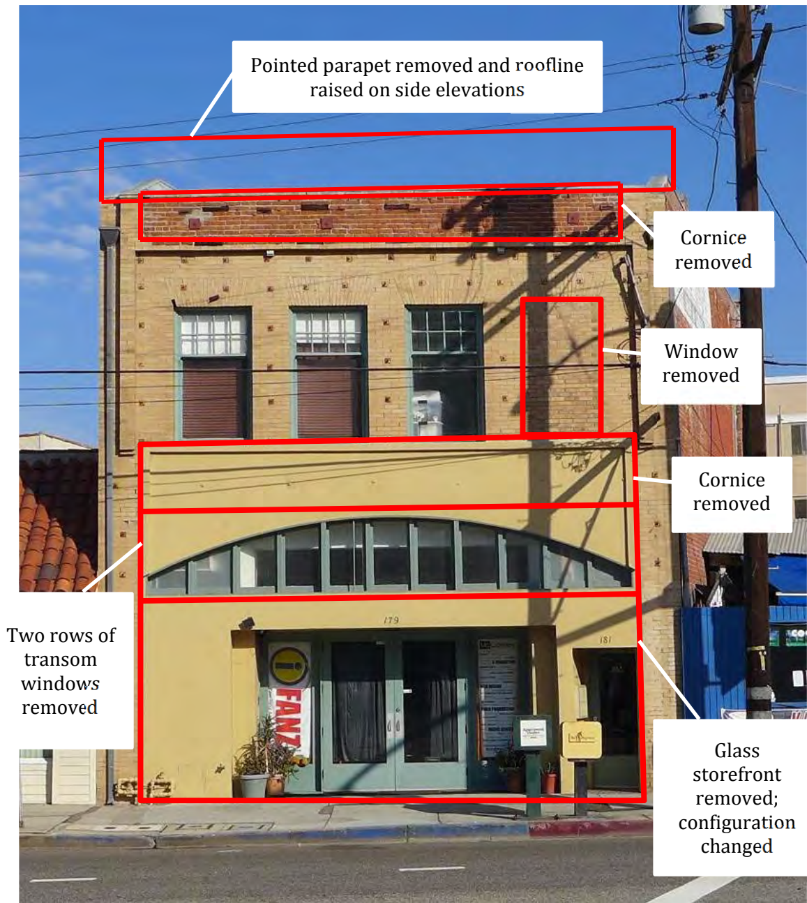
Figure 47. Alterations to historic appearance of the subject property from the primary period of significance 1904 to 1933 (PCR 2015)
