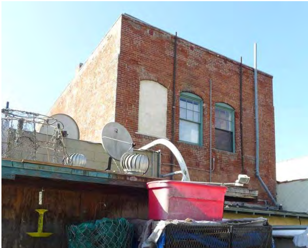
Figure 27. Rear (north) elevation, partially obstructed, view southwest(PCR 2015)
