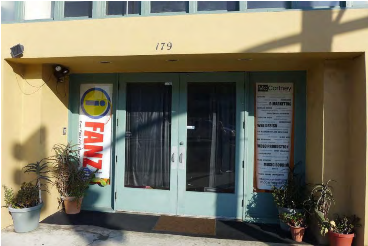
Figure 23. Recessed entry (alteration), with composite double-doors each with a large single-pane light, and two large side lights (alteration), view north (PCR 2015)
