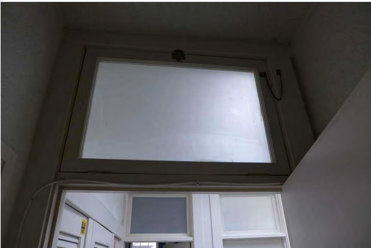
Figure 43. Transom above doorway, second floor (alteration, glass replaced) (PCR 2015)
