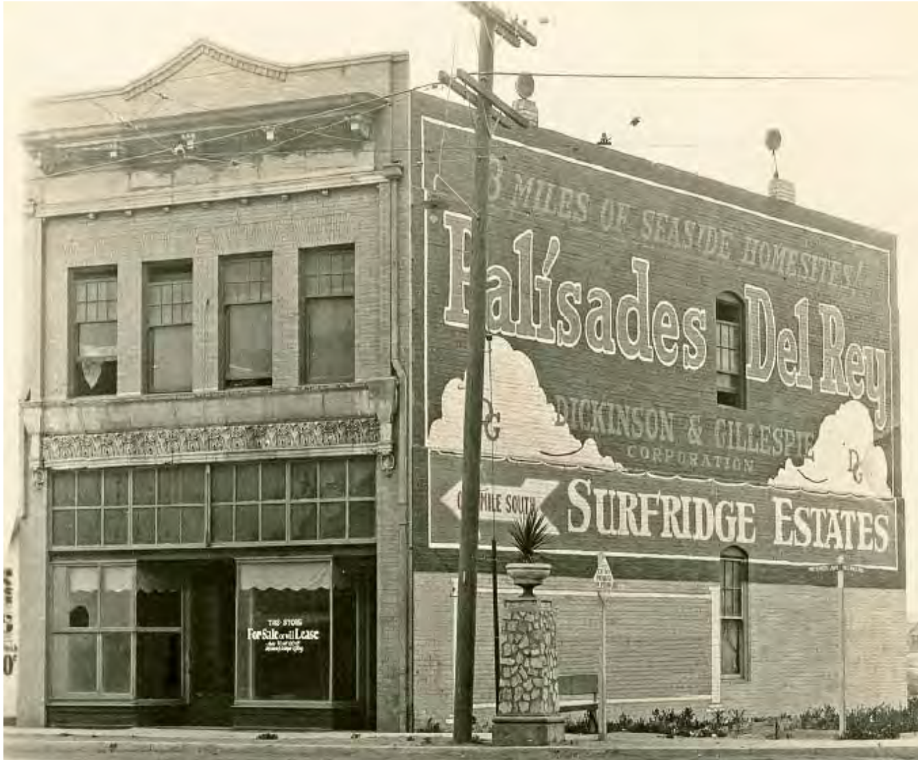
Figure 13. Original appearance of the subject property during the primary period of significance, showing pointed parapet, cornices, two rows of transom windows, and glass storefront (all removed) (McMahon, Historic-Cultural Monument Application, Playa del Rey Commerce Building, original provenance unknown)
