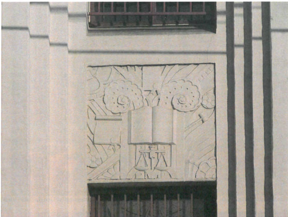
Redwine Building, panel above entrance, 1618 N. Las Palmas Avenue, Feb. 5, 2015 (photograph by Charles J. Fisher)
