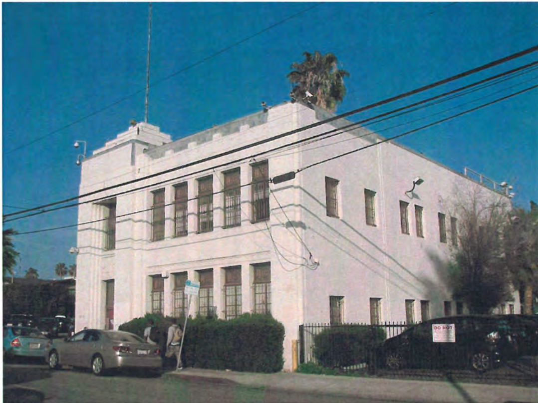
Redwine Building, 1618 N. Las Palmas Avenue, February 5, 2015 (photograph by Charles J. Fisher)
