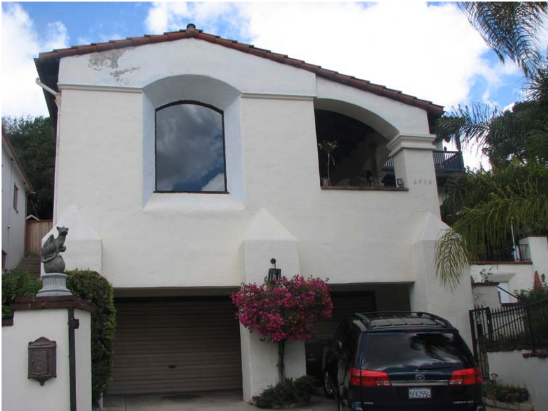
Durex Model Home, garage under living room and porch, 3410 Amesbury Road, April 11, 2012 (Photograph by Charles J. Fisher)
