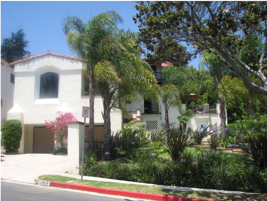
Durex Model Home, street view, 3410 Amesbury Road, June 29, 2011 (Photograph by Charles J. Fisher)
