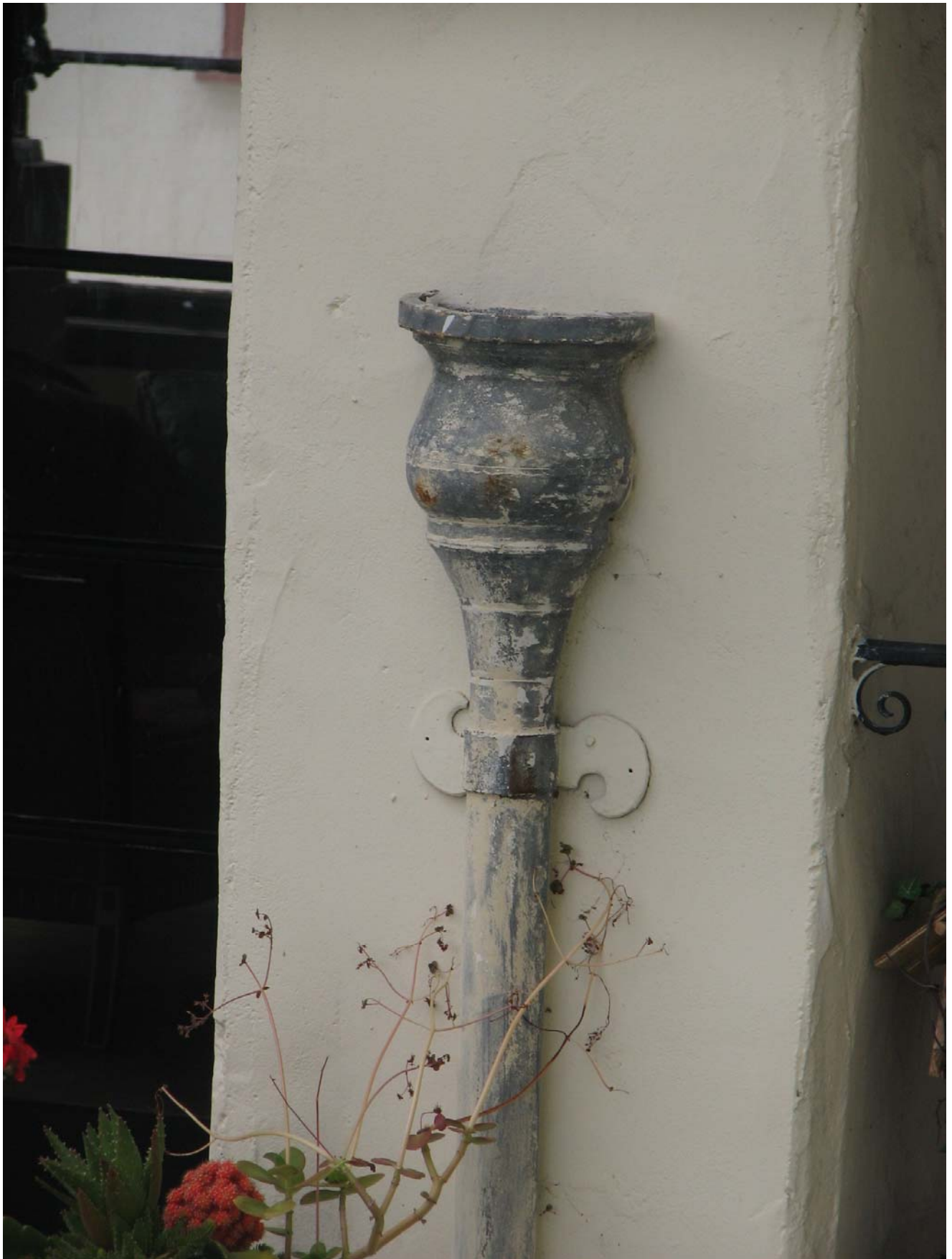
Durex Model Home, original copper downspout, 3410 Amesbury Road, April 11, 2012 (Photograph by Charles J. Fisher)
