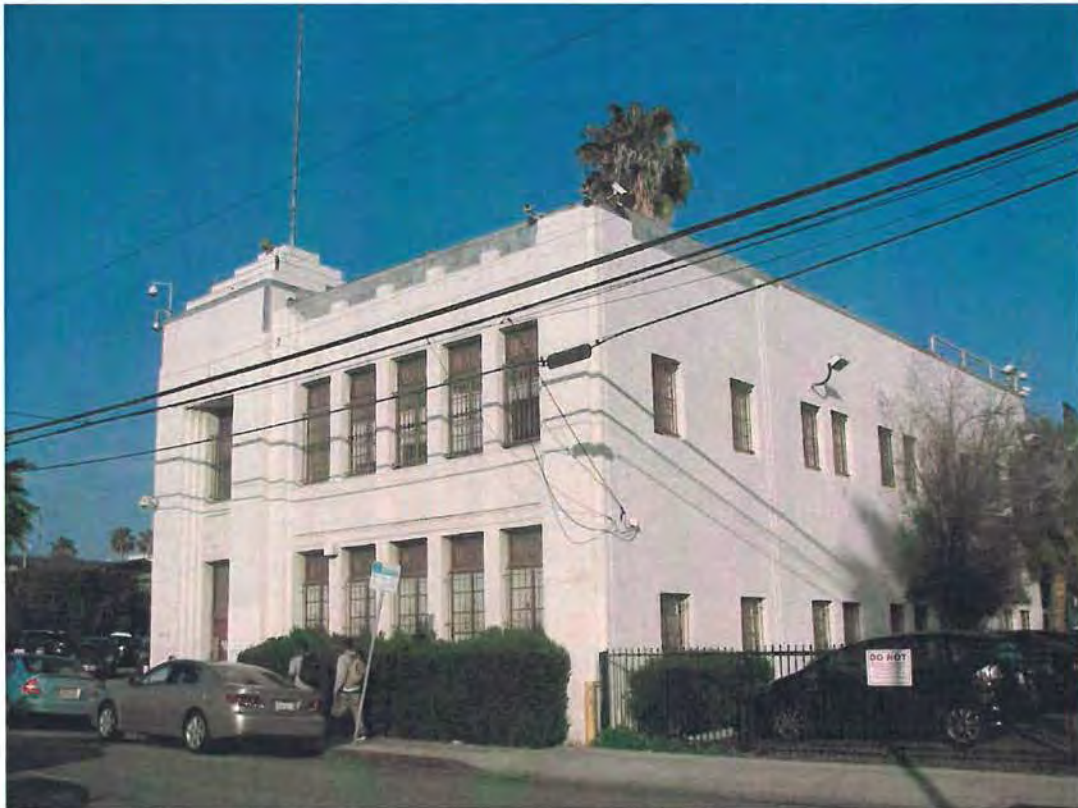
Redwine Building, 1618 N. Las Palmas Avenue, February 5, 2015 (photograph by Charles J. Fisher)
