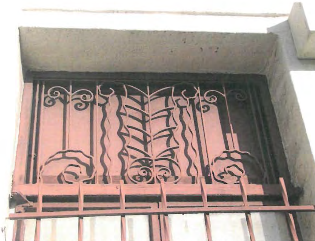
Redwine Building, window grille, 1618 N. Las Palmas Avenue, February 5, 2015 (photograph by Charles J. Fisher)
