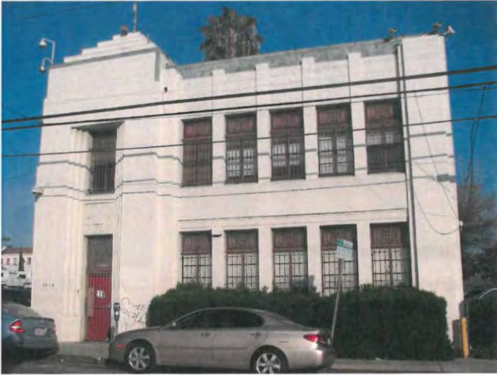
Redwine Building, 1618 N. Las Palmas Avenue, February 5, 2015 (photograph by Charles J. Fisher)
