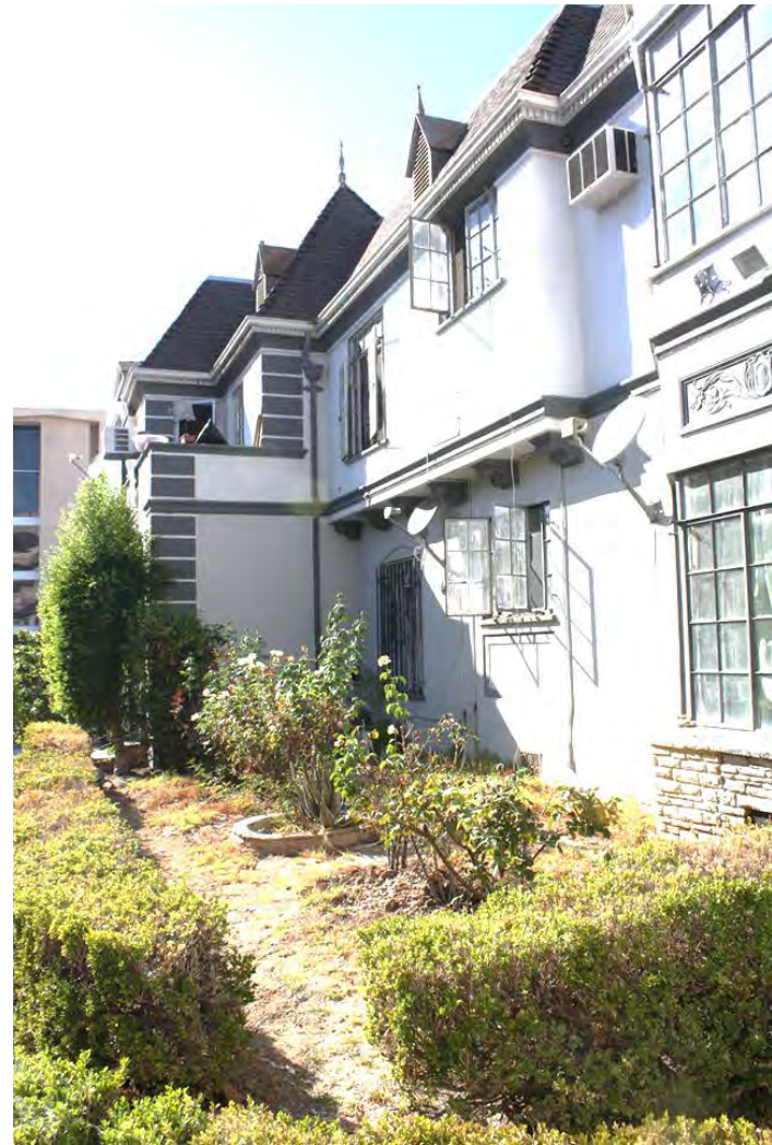
View along south façade of building: Balcony of upper west unit; quoining; steeply pitched roof; pinnacled gables; casement windows; French stone trim, window bay; banding; dentils; cantilevered 2 nd story & brackets; cast trim panels; view west.
