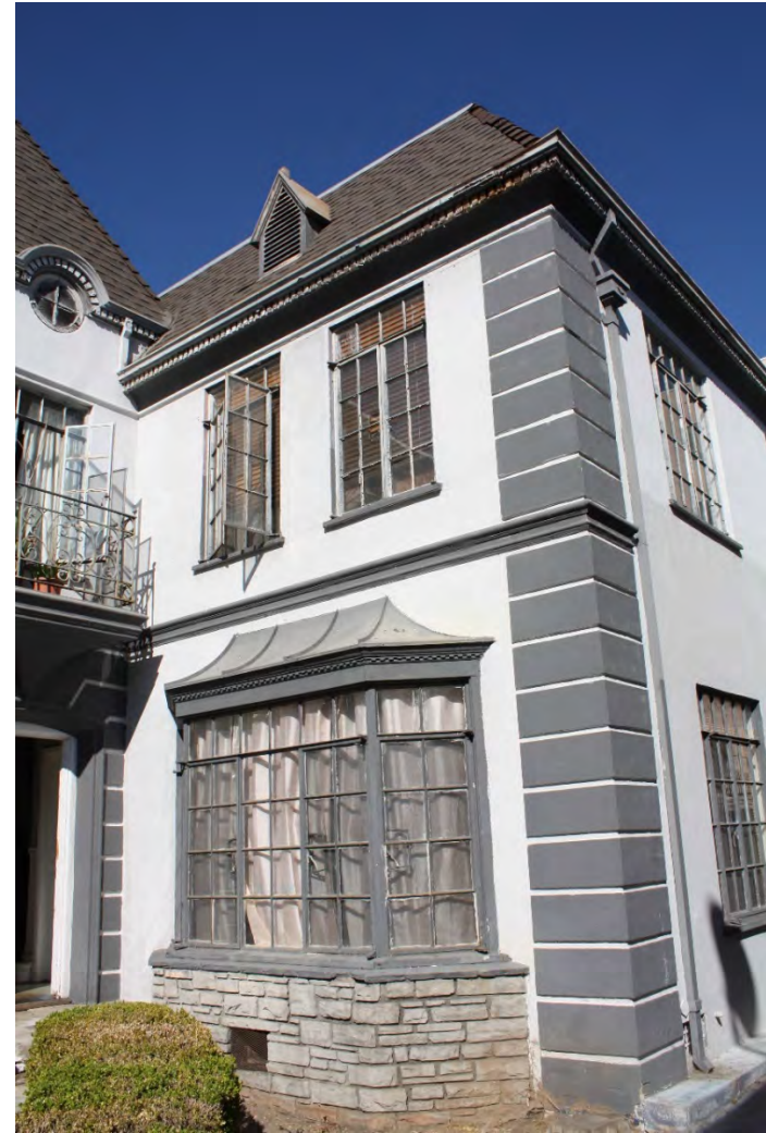
West elevation: French stone base of multi-pane casements and flared metal roofette: banding; two paired multi-pane casements with fixed multi-pane transom; step pitched roof/flat deck with gabled dormer vent, ; dentil trim; quoining at southwest corner, view northeast.
