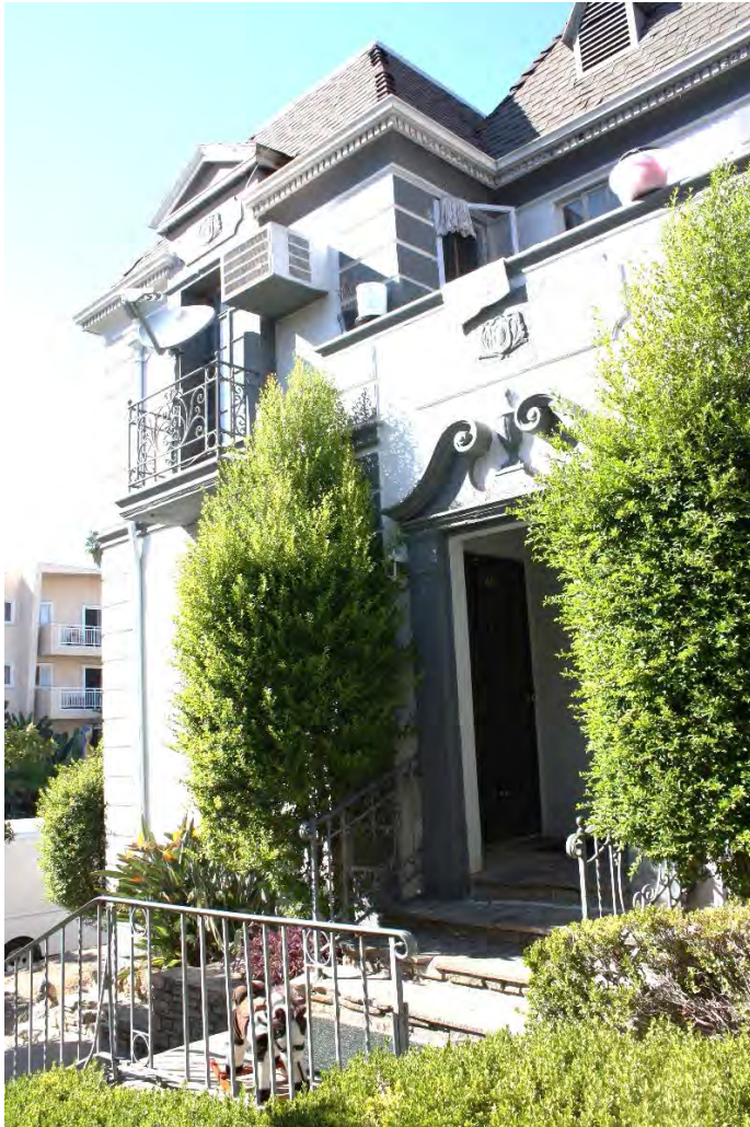
Raised entry to unit 412: Cantilevered balconette/wrought iron balustrade; pediment gable with stucco trim panel beneath; broken pediment with urn above entry; decorative panel on stucco balcony; original wrought iron banisters, view northwest.
