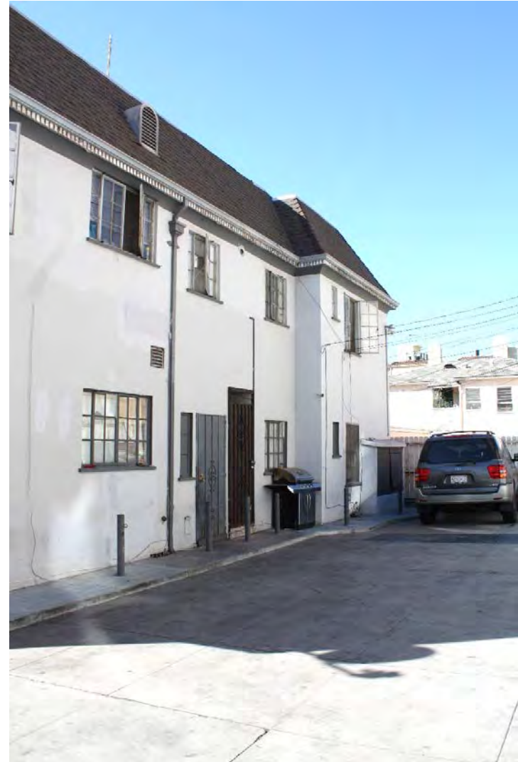
East elevation, continued: Steel casement windows; steep hipped roof with flat deck/arched top dormer vent; dentil trim at roofline; gutter/downspouts; return with higher roof, view north.
