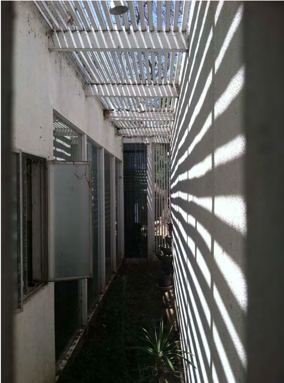
View of northern side yard featuring floor-to-ceiling glass, steel casement windows, landscaped area, screening wall, and wooden lattice sun screen. Photographed August 9, 2015.
