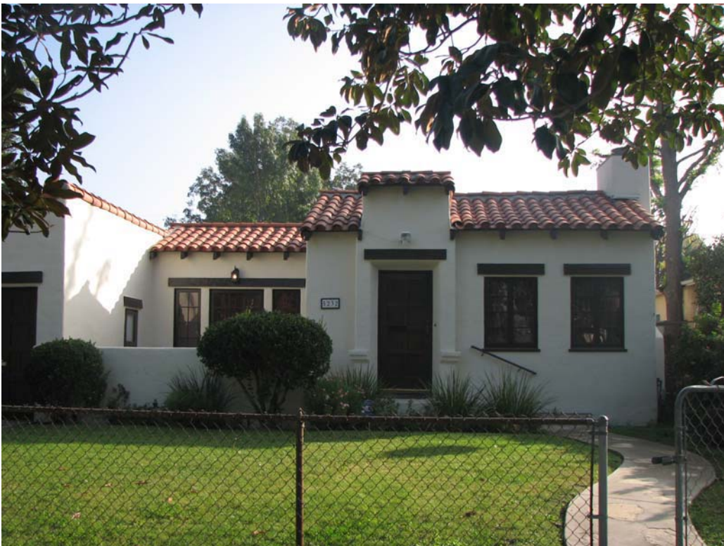
Sheridan House, 5232 N. Sylmar Avenue (Photograph by Charles J. Fisher)
