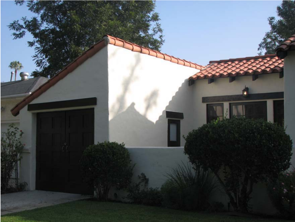
Sheridan House, garage and front patio, 5232 N. Sylmar Avenue (Photograph by Charles J. Fisher)
