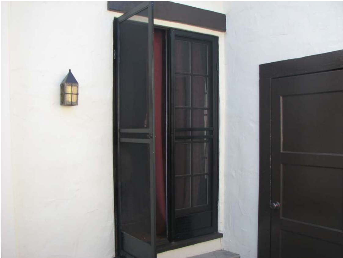
Sheridan House, French doors to side patio, 5232 N. Sylmar Avenue (Photograph by Charles J. Fisher)
