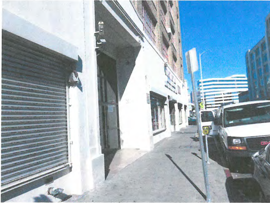
Original 1923 Entrance, and storefront modified in 1960 by furring out over original material.
