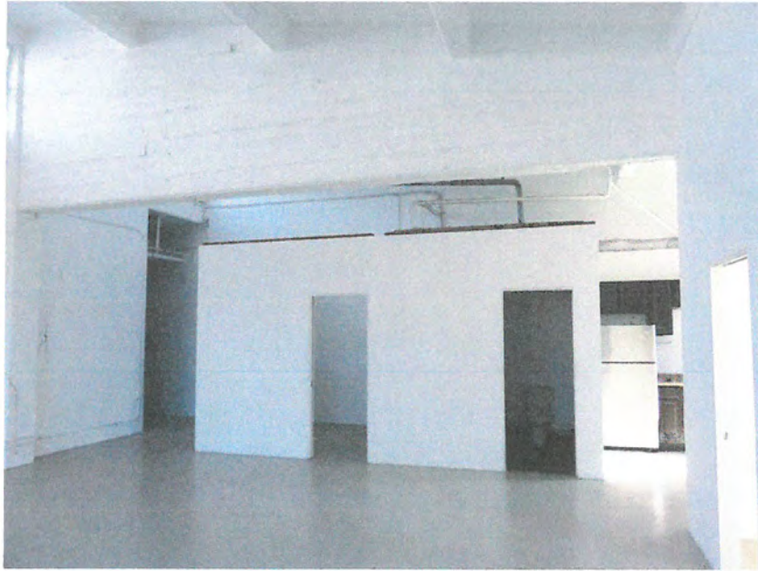
Interior conditions on the 6th Floor. Ceiling beams are exposed.
