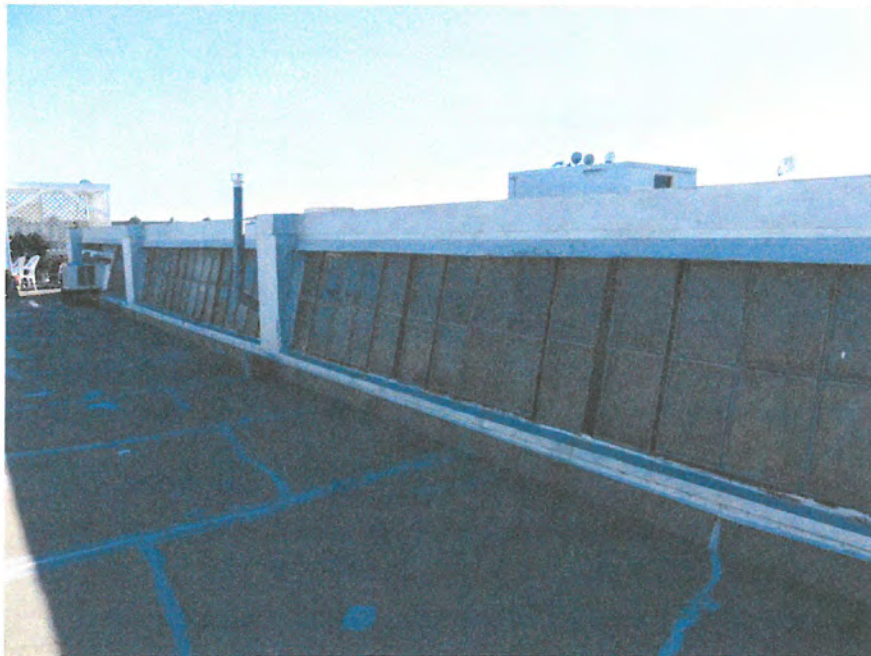
Monitor roofs have original steel sash.
