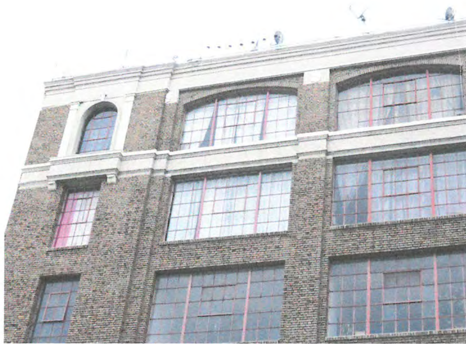
Upper story, modest neoclassic detailing adds stylistic identity to a manufacturing building, typical of the early work of W. Douglas Lee.
