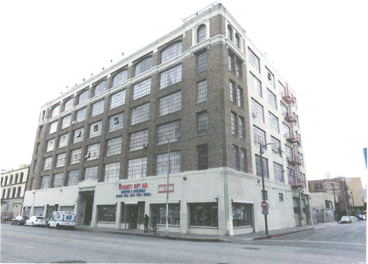
Catalina Swimwear Building, Primary façade (east) and secondary (north) elevation. The building is highlighted and characterized by Neoclassic detailing on the sixth floor. The first story of the façade is furred out, obscuring the original terra cotta pilasters which survive behind the stucco.
