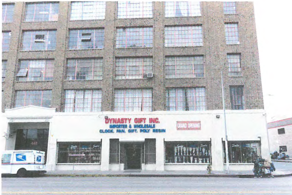
Former storefront openings conform to window placement on upper façade. Original pediment remains over recessed central entrance.
