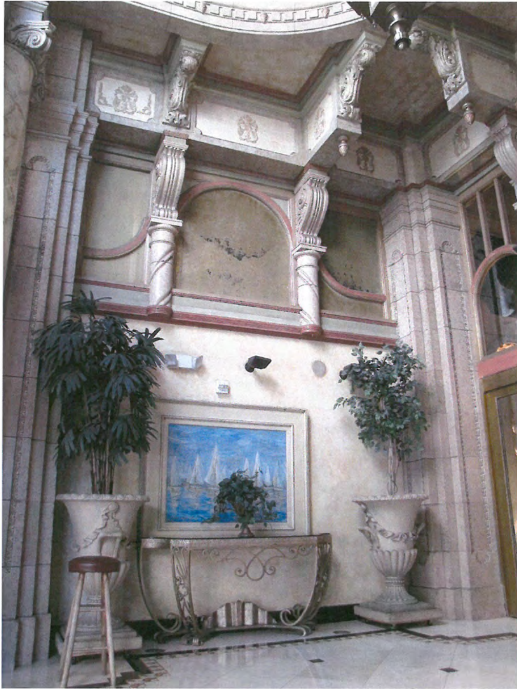
Figure 17: View NE of the terra cotta detailing inside the loggia.
