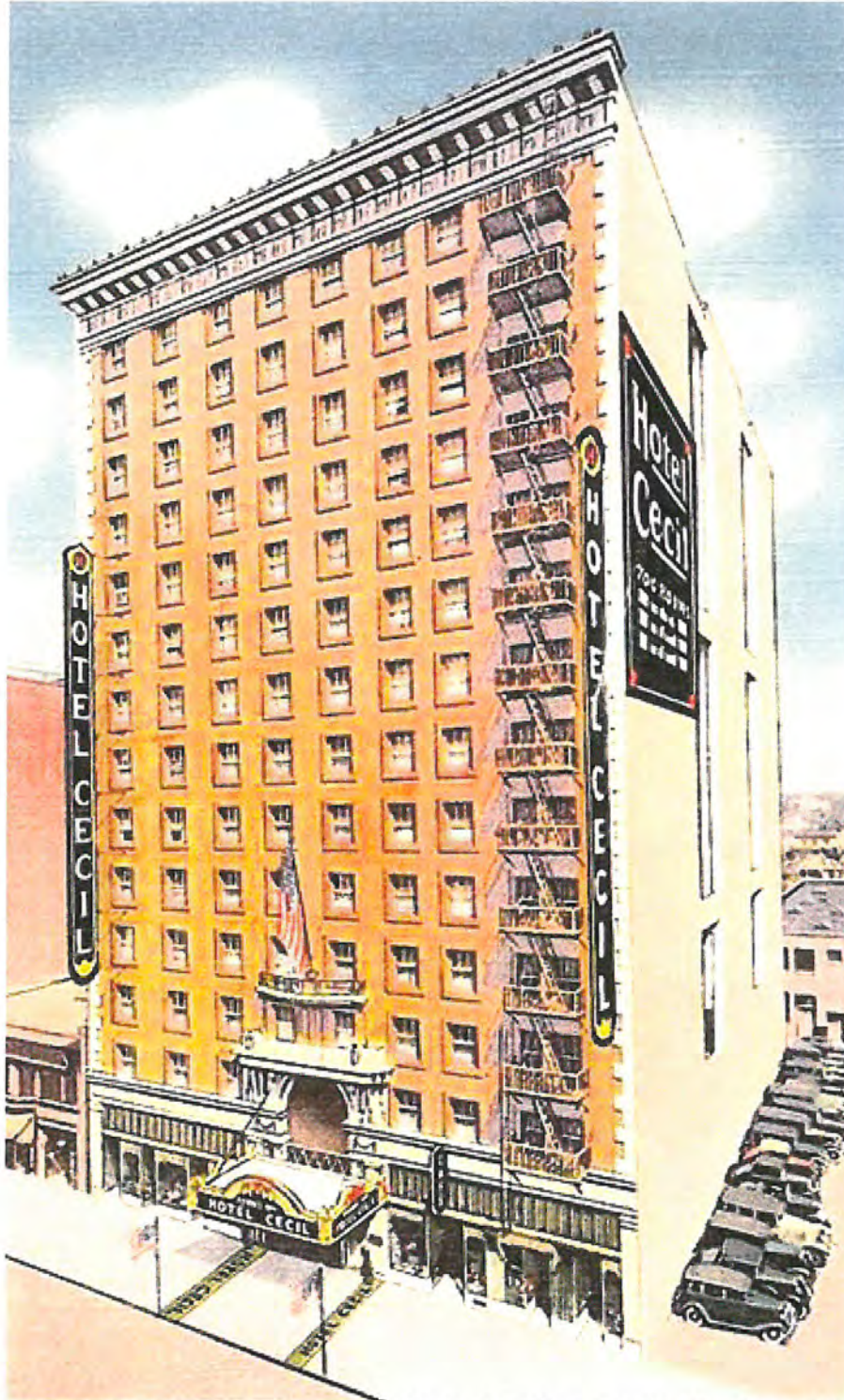
Figure 6: Undated color postcard showing west (S Main Street) and south elevations of the Hotel Cecil. The prominent blade signs were not indicated on L.L. Smith's original plans, although City of Los Angeles Building Permit #46860 indicates they were installed at the time of construction in 1924.
