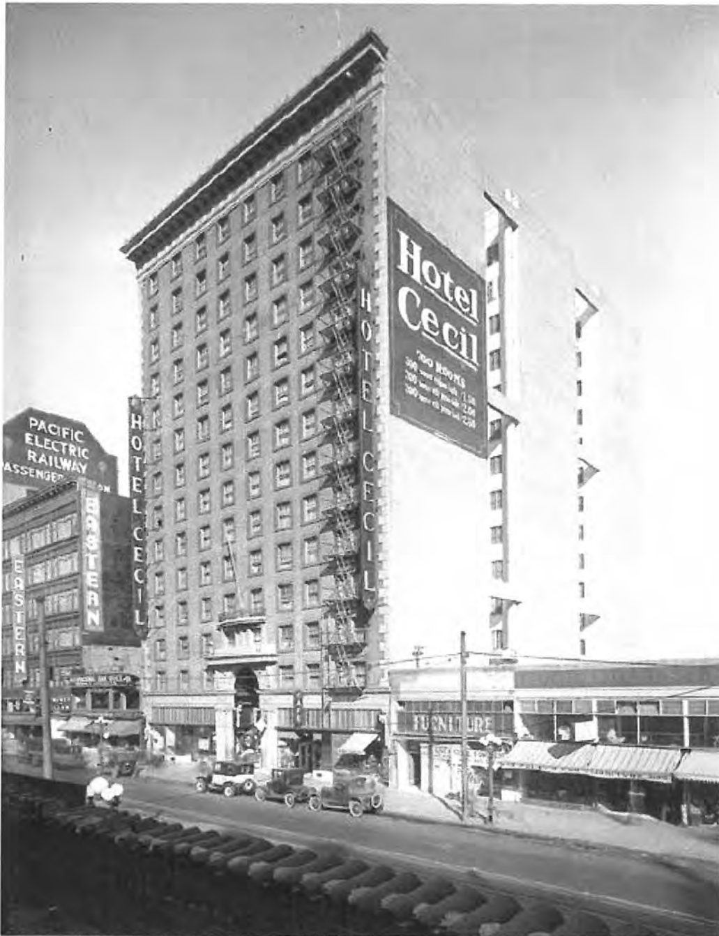
Figure 8: Undated black and white photograph showing the front (S Main St) and south elevations of Hotel Cecil. The advertisement painted on the south elevation of the building indicates Hotel Cecil as having 700 rooms, a fact that is discredited by early occupancy permits and the historic architectural drawings.
