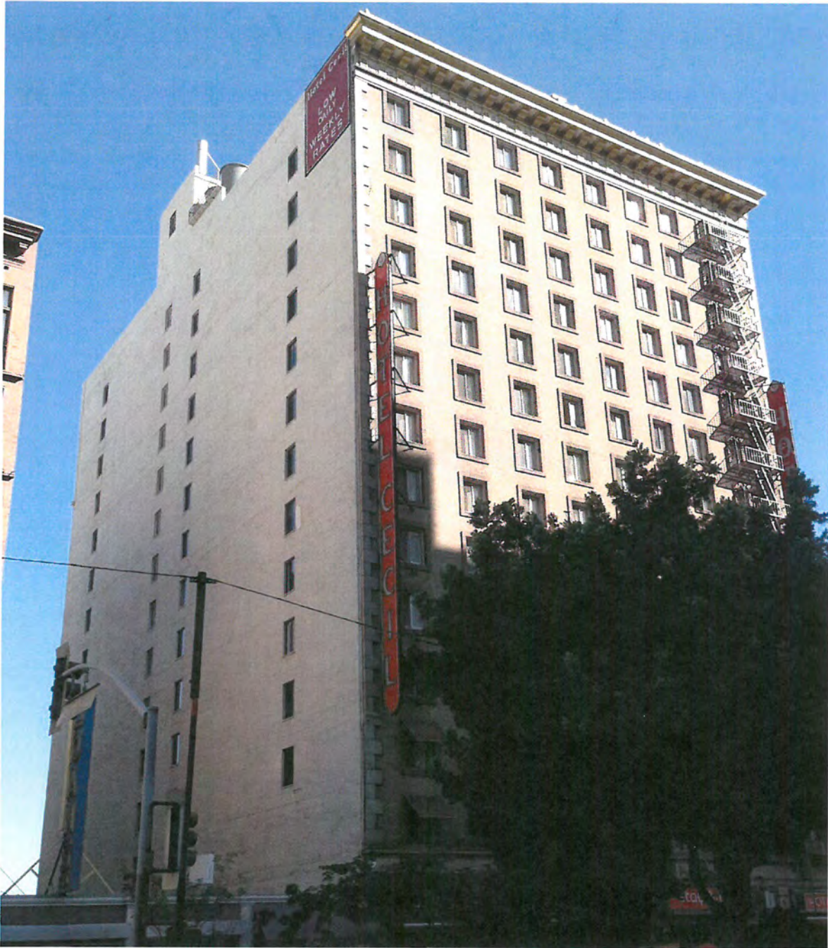
Figure 15: The north and partially-obscured west elevations of Hotel Cecil.
