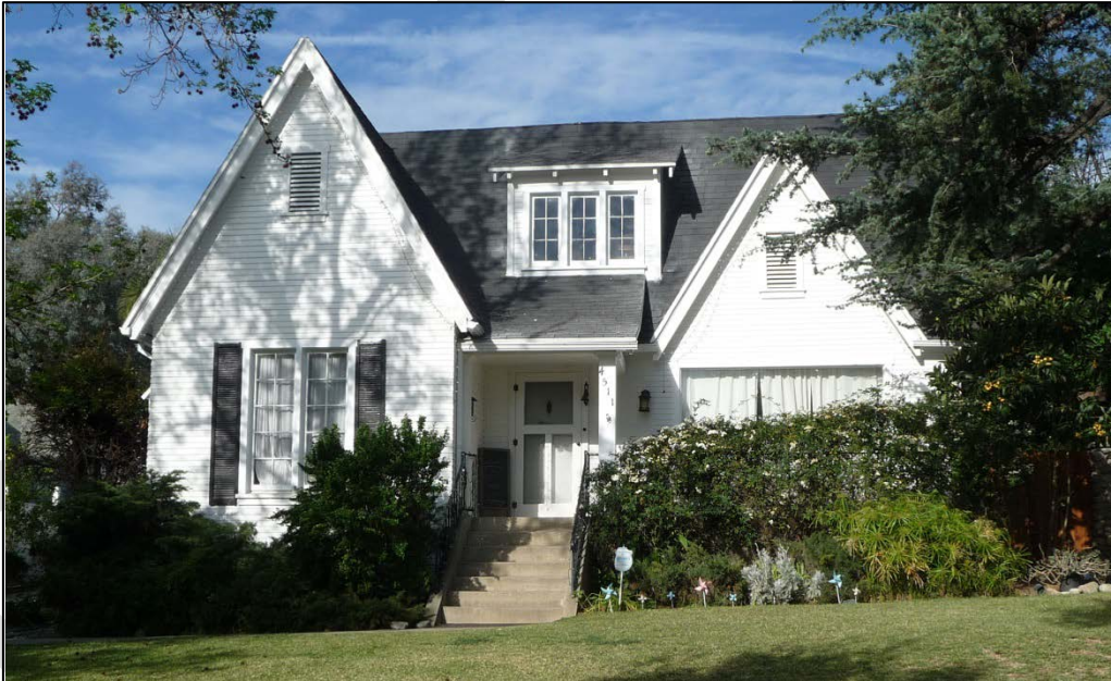
Example of the English Tudor Revival style. 4511 N Berkshire Ave.
