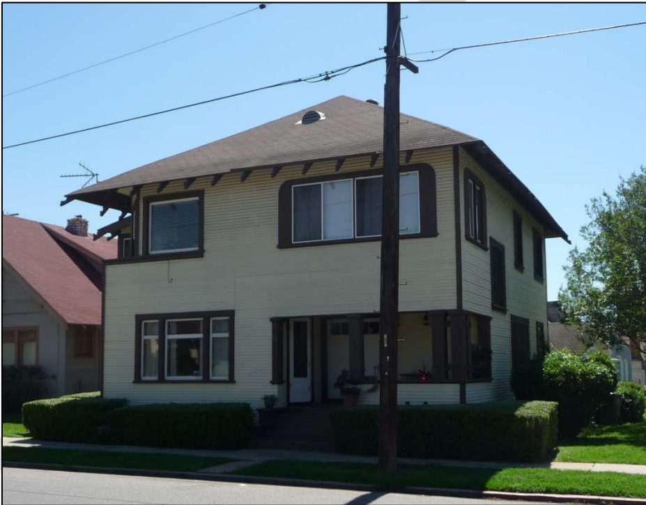
Example of the American Foursquare style. 5704 E Kendall Ave.
