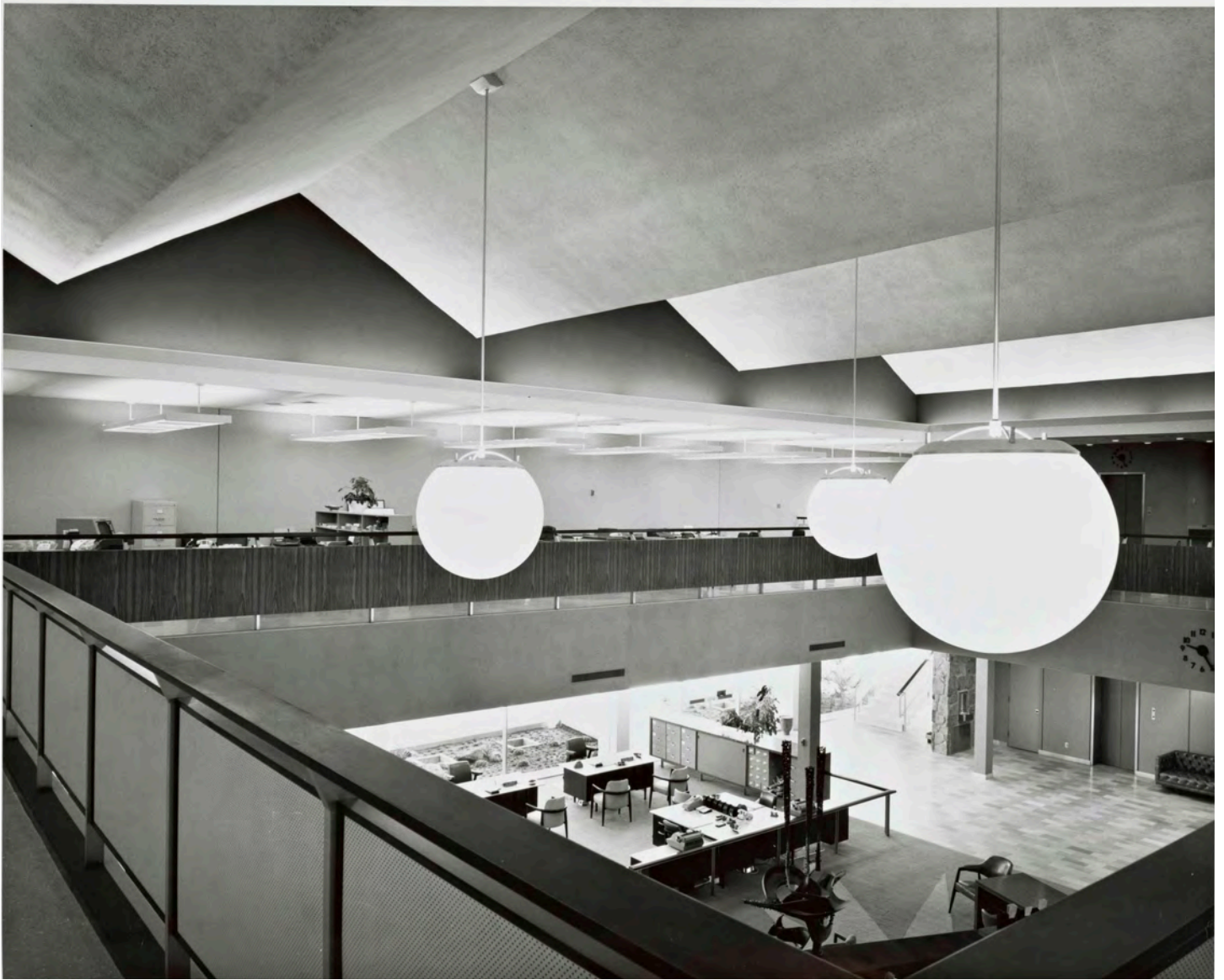
Interior Balcony With Folded Plate Roof and Ground Floor Offices (1960) Photo Julius Shulman. J. Paul Getty Trust. Getty Research Institute, Los Angeles (2004.R.10)
