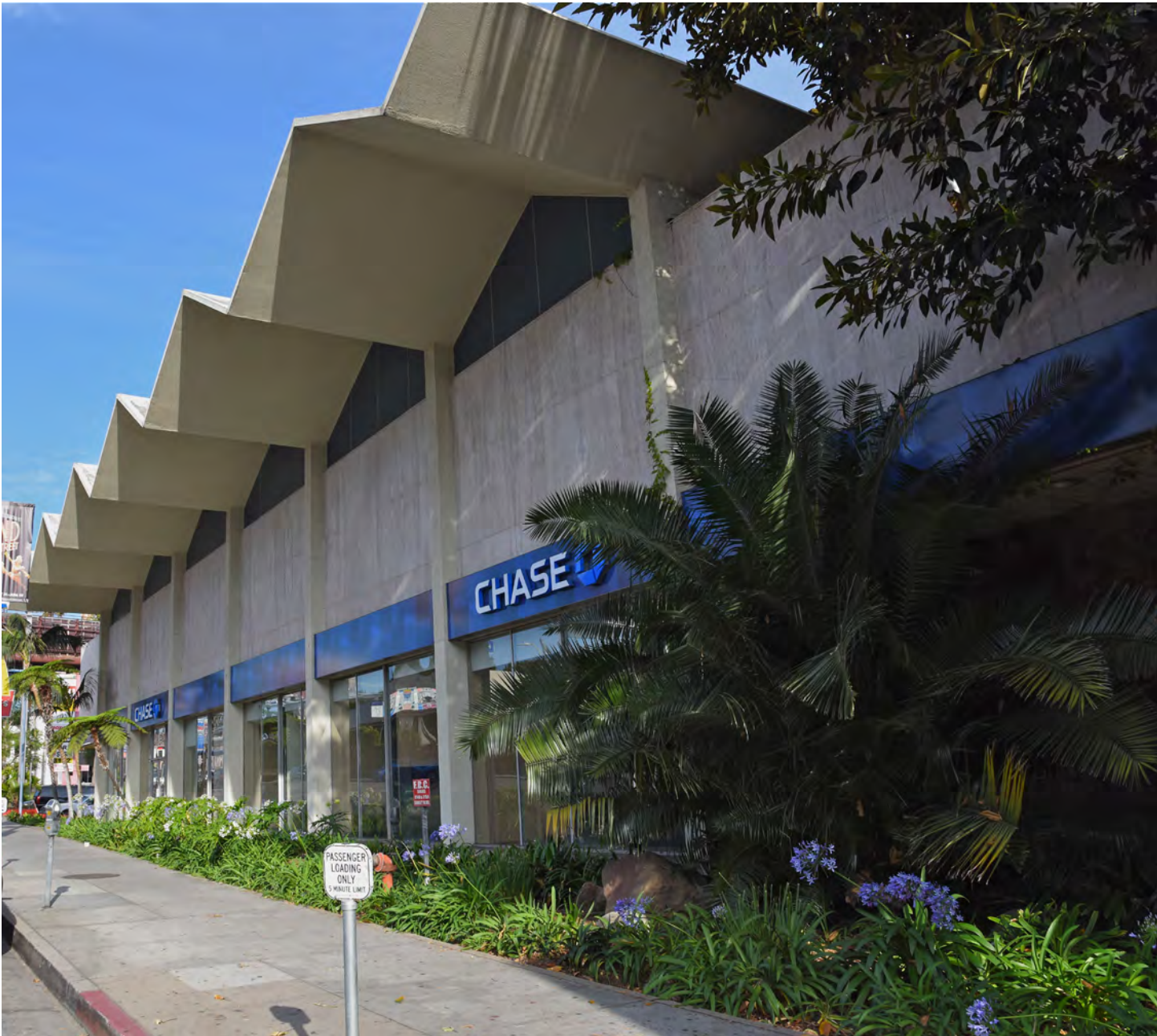
North elevation, view southeast. (2016) Photo Keith Nakata
