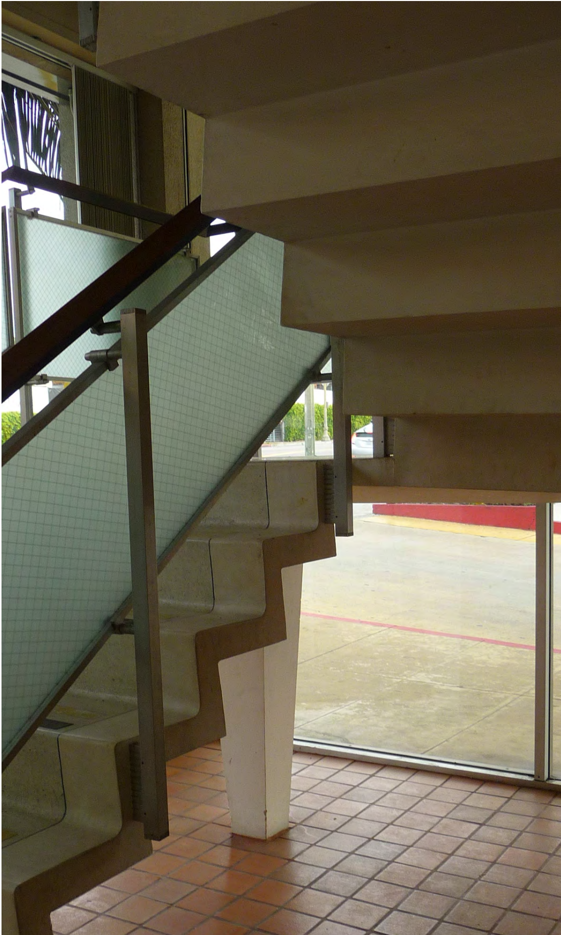
Northeastern Corner Floating Staircase Encased in Glass First Floor, looking northeast (2016) Adrian Fine
