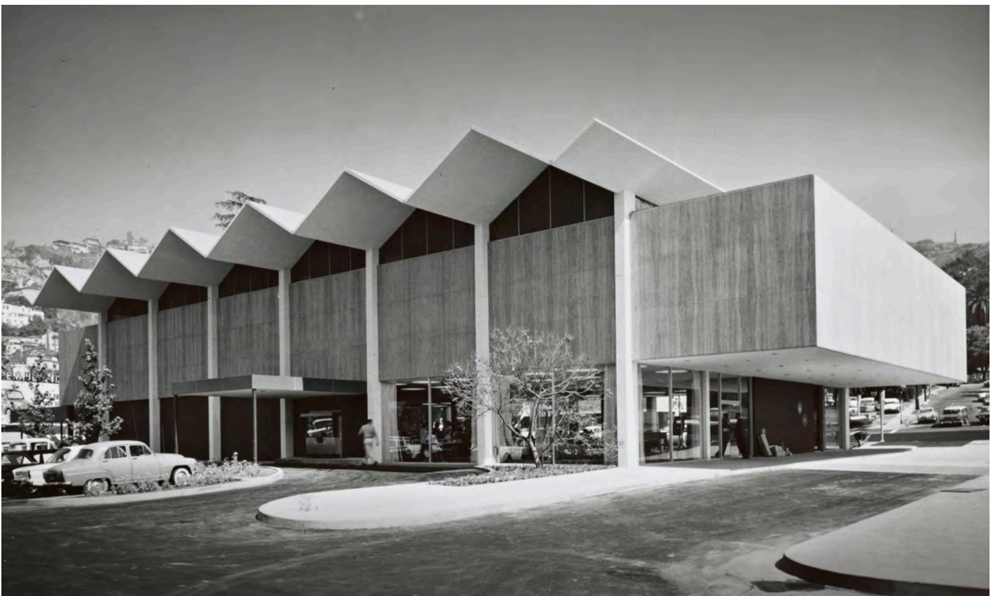
South and East Elevations, looking northwest (1960) Photo Julius Shulman. J. Paul Getty Trust. Getty Research Institute, Los Angeles (2004.R.10)
