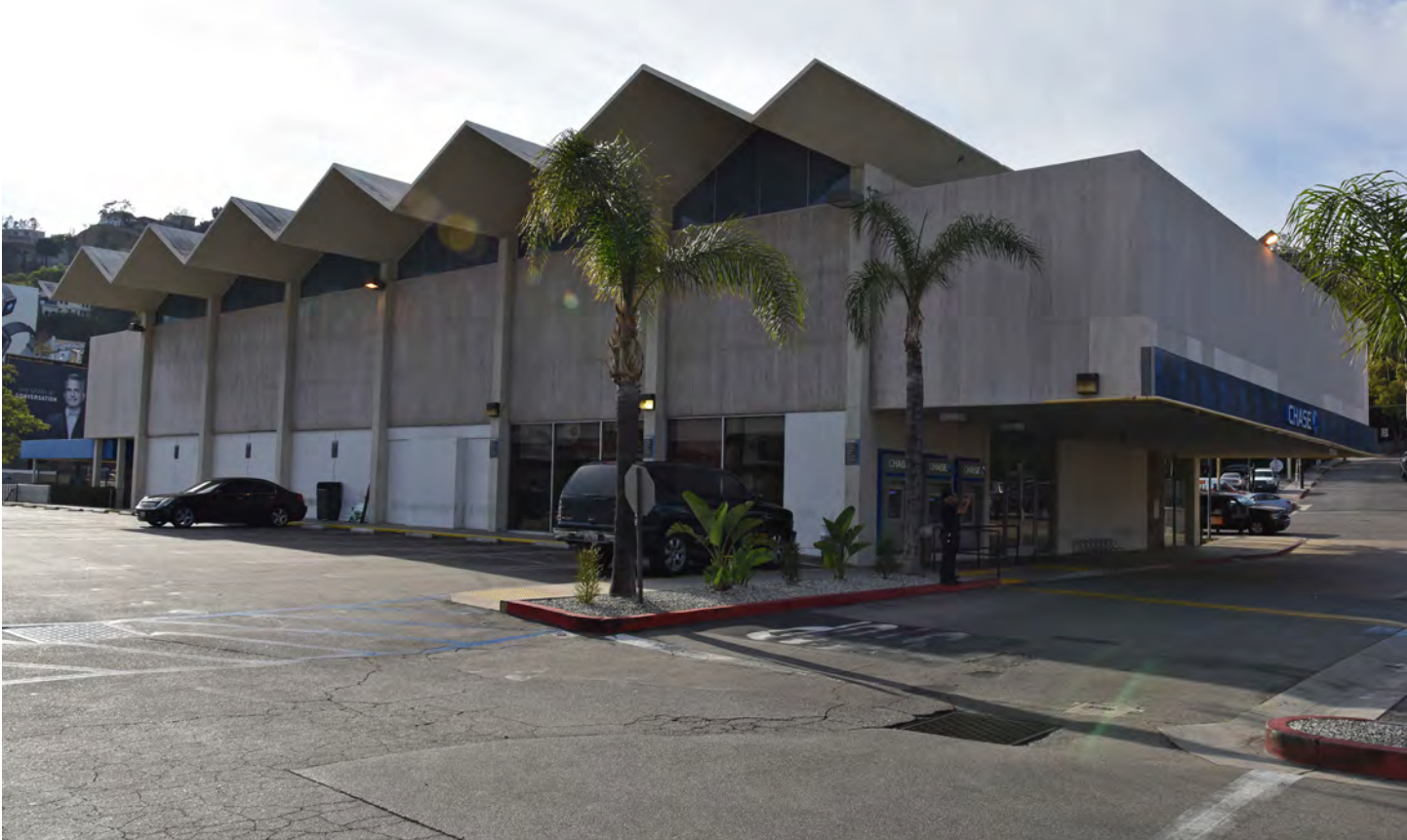
South and east elevation, view northwest. (2016) Photo Keith Nakata
