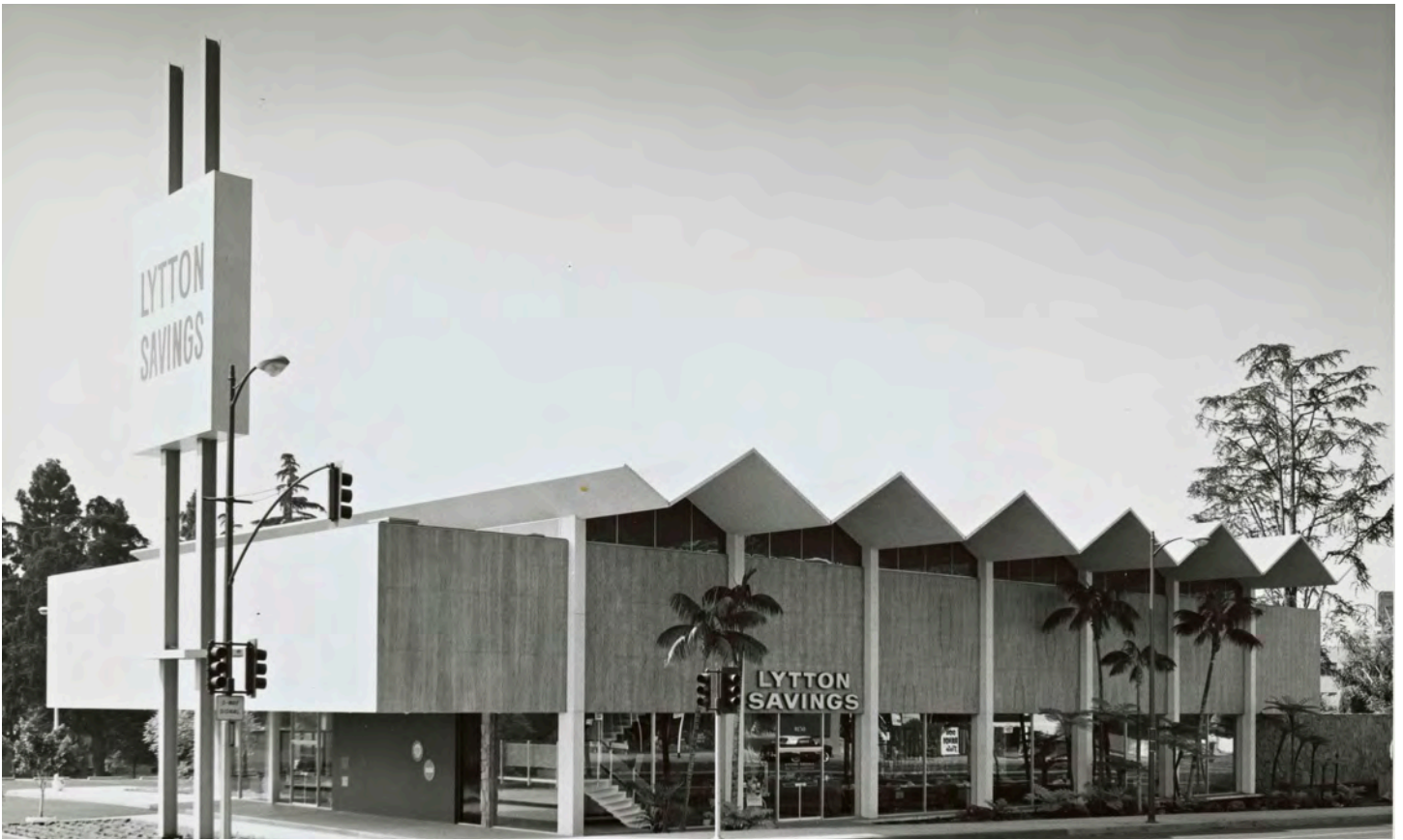
North Elevation view southeast (1960) Photo Julius Shulman. J. Paul Getty Trust. Getty Research Institute, Los Angeles (2004.R.10)
