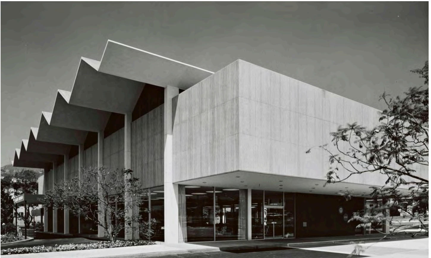
South and East Elevations, looking northwest (1960) Photo Julius Shulman. J. Paul Getty Trust. Getty Research Institute, Los Angeles (2004.R.10)
