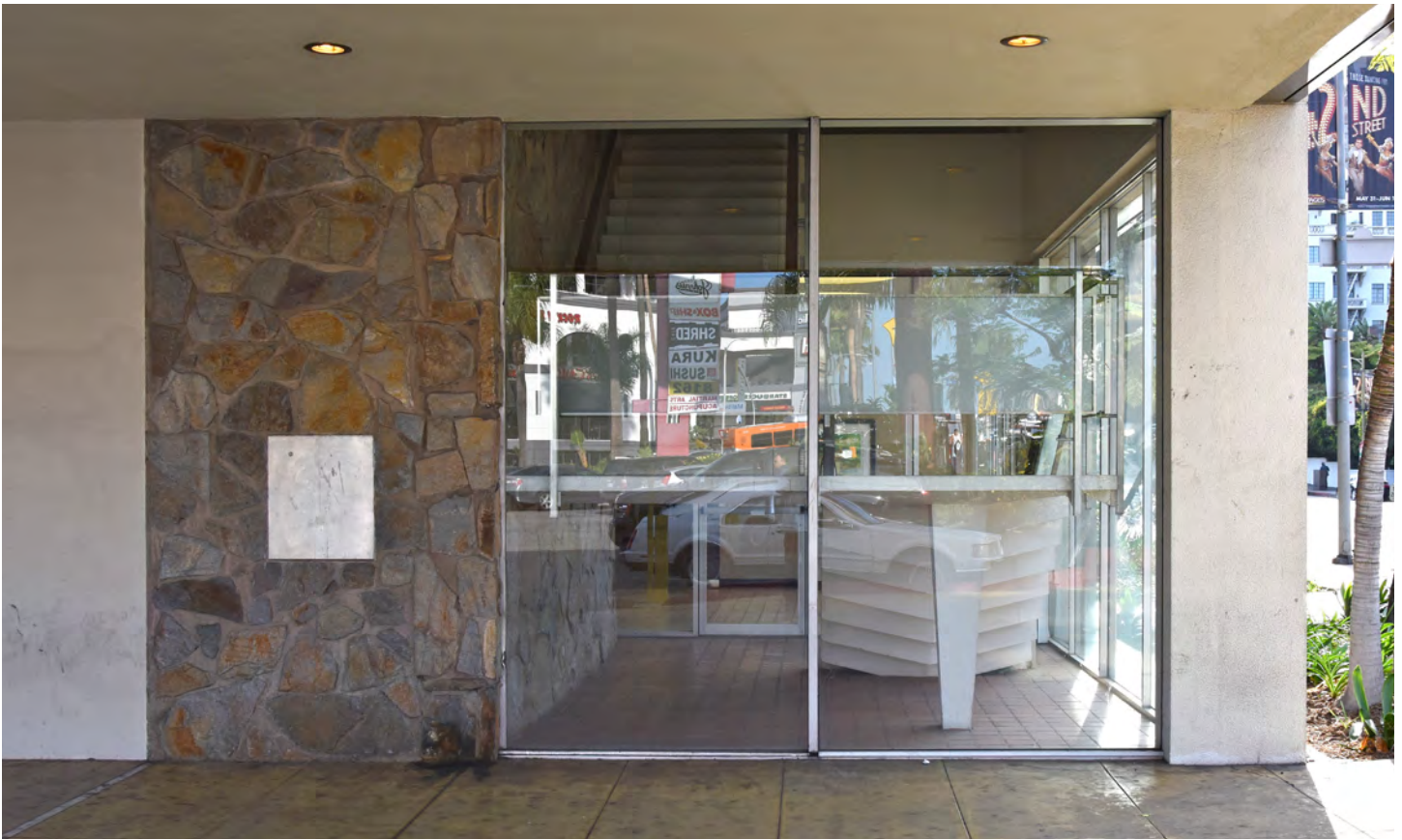
Northeastern Corner Stairwell view west (2016) Keith Nakata
