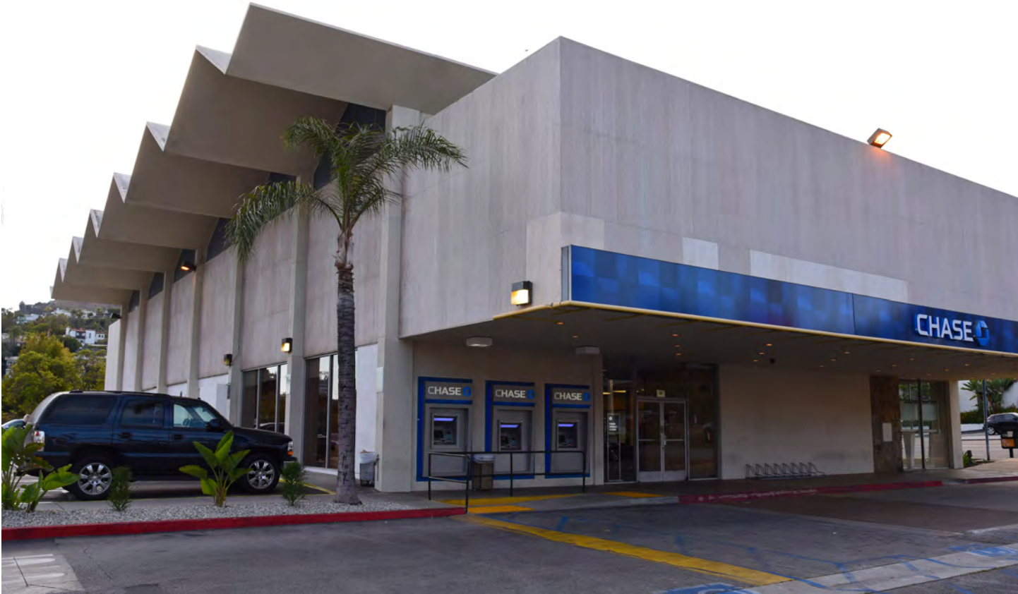
South and east elevation, view northwest. (2016) Photo Keith Nakata
