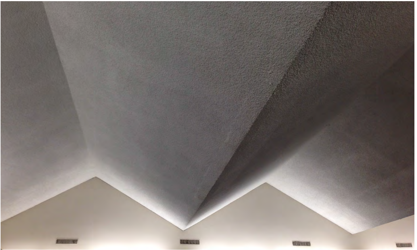
Interior View of Folded Plate Roof Design (2016) Adrian Fine
