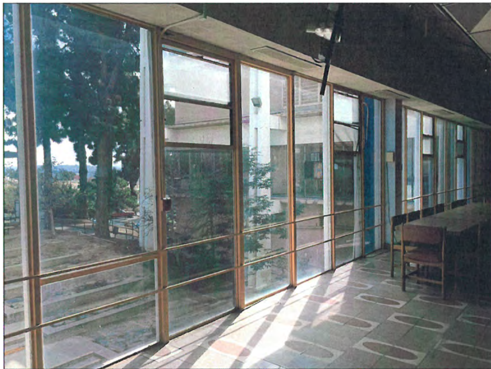
Figure 28: Building 2, interior, second floor windows, view southeast (Snow, 2016)
