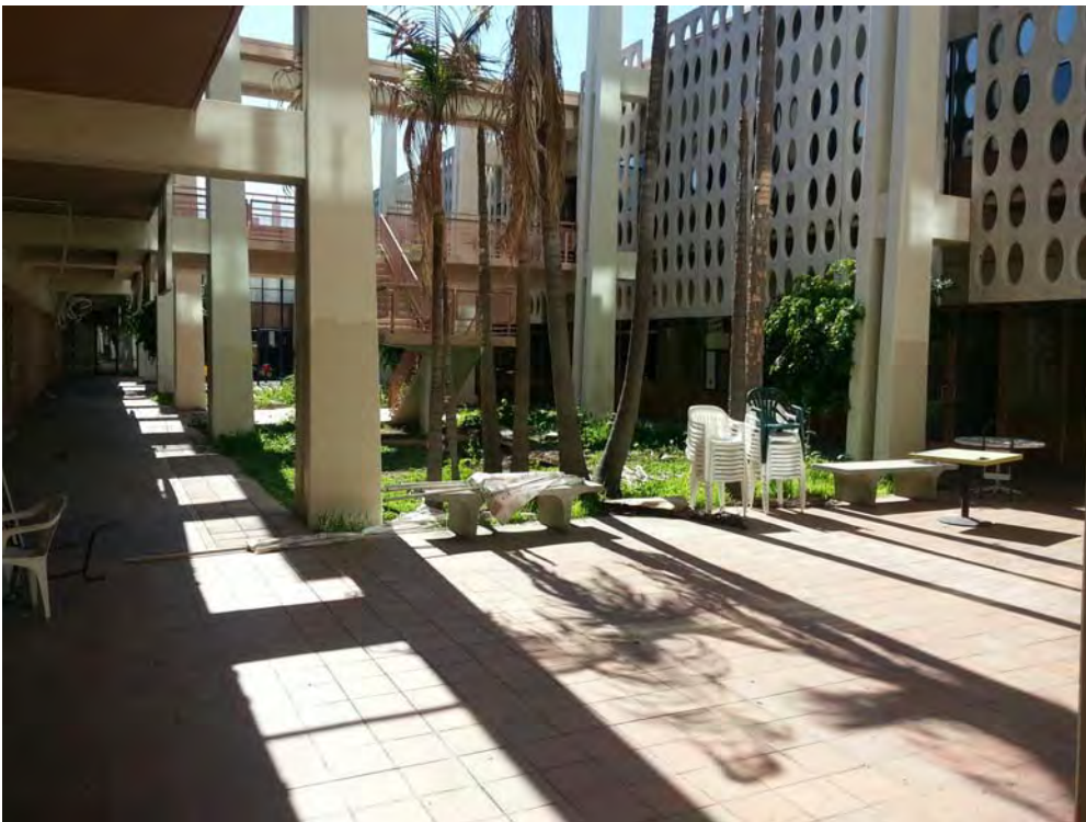
60. Courtyard looking southeast
