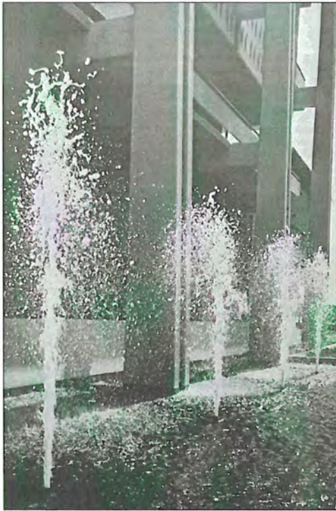
Historic Photograph 30: Building 3a, west elevation, view southeast (1964, MWD Annual Report)
