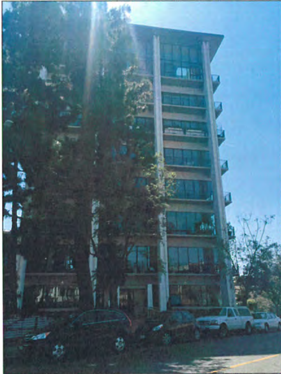
Figure 51: Building 4, east elevation, view west (Snow, 2016)
