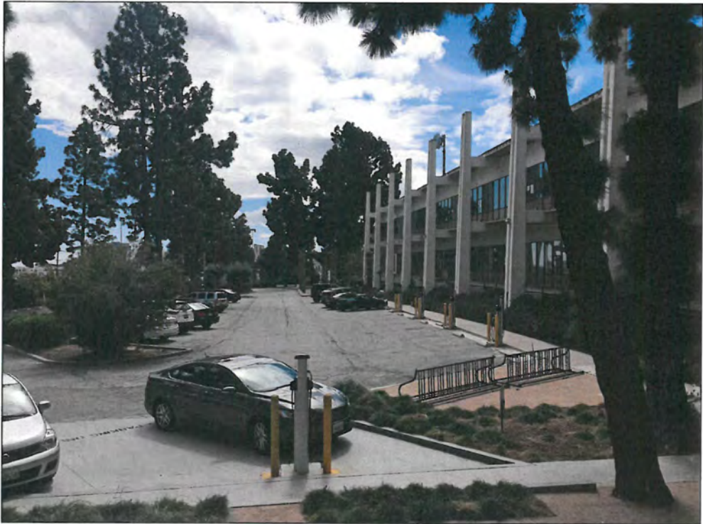
Figure 30: Building 3b, east elevation, view south (Snow, 2016)
