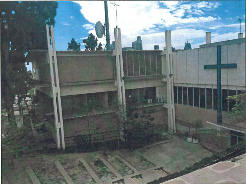
Figure 23: Building 2, east elevation, view southwest from Building 3 (Snow, 2016)
