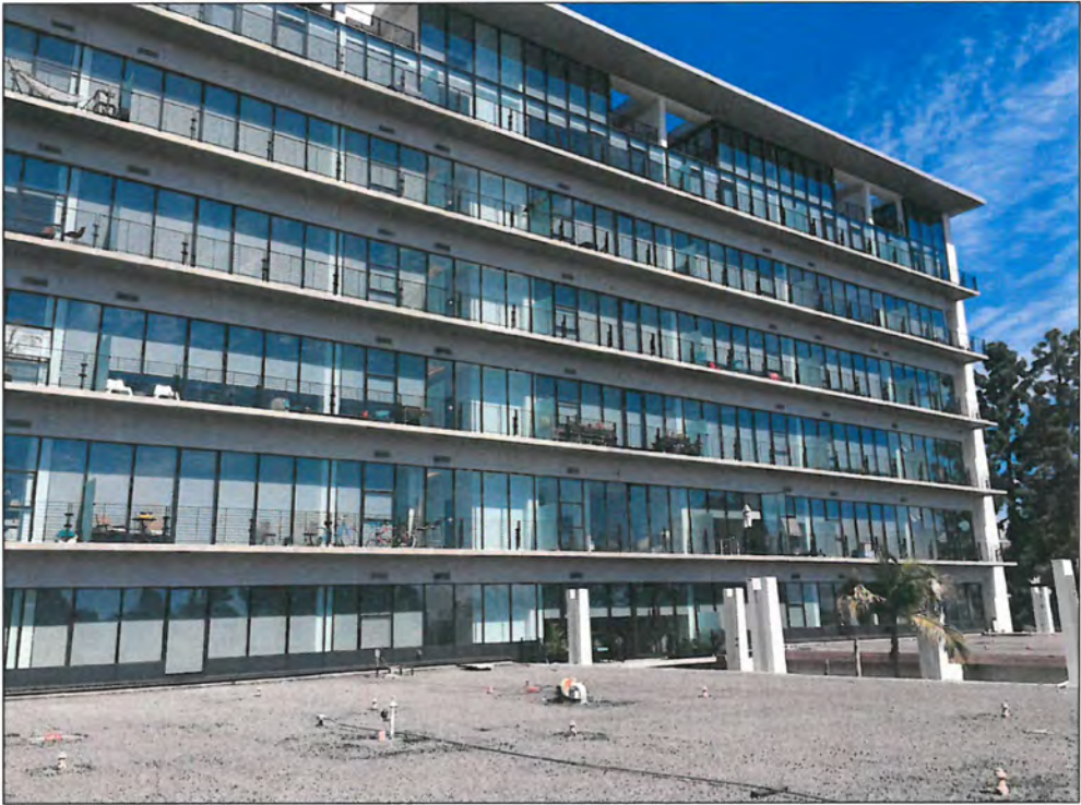
Figure 50: Building 4, south elevation, view northeast from roof of Building 3 (Snow, 2016)
