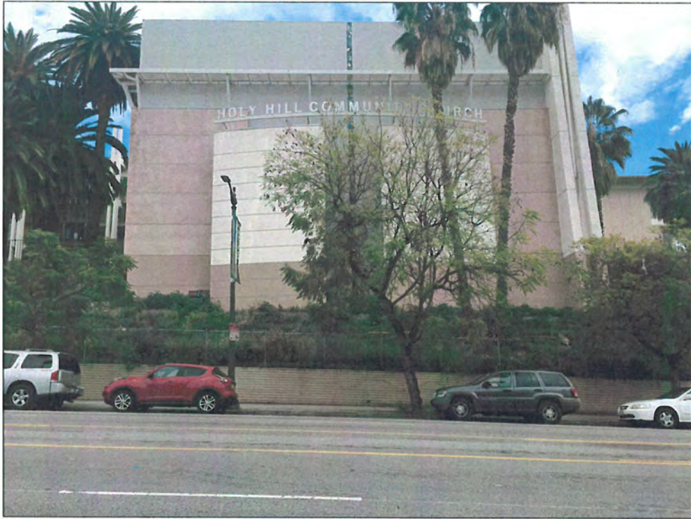
Figure 55: Building 5, west elevation, view east (Snow, 2016)
