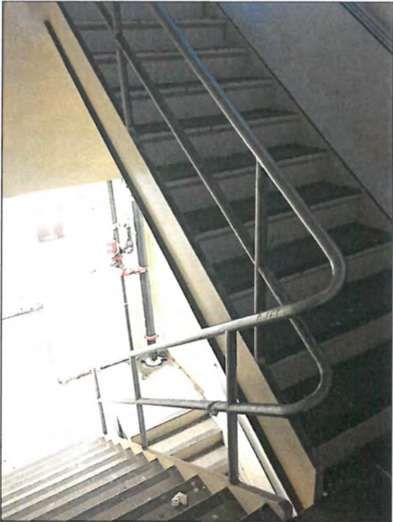
Figure 45: Building 3a and 3b, interior, typical stair (Snow, 2016)
