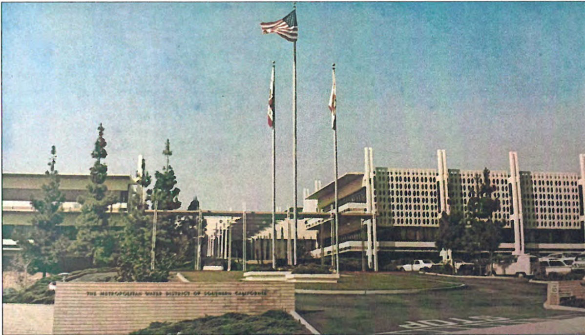
Historic Photograph 35: Building 1 (left), Building 2 (center) and Building 3b (right), east elevation, view west (1966, MWD Annual Report)
