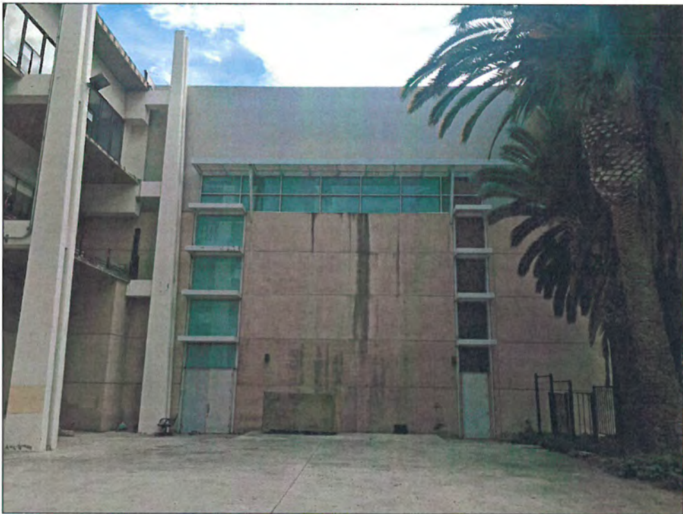
Figure 56: Building 5, north elevation, view south (Snow, 2016)
