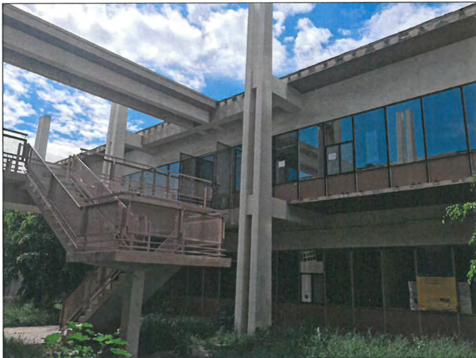
Figure 38: Building 3a and 3b, interior courtyard, view southeast (Snow, 2016)
