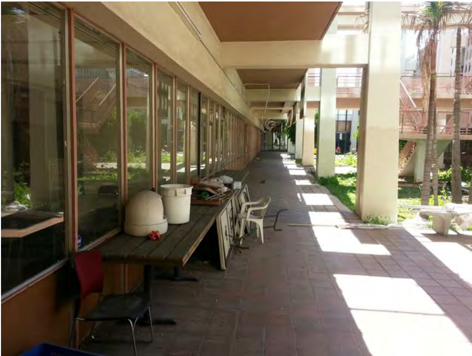
58. View of courtyard looking east
