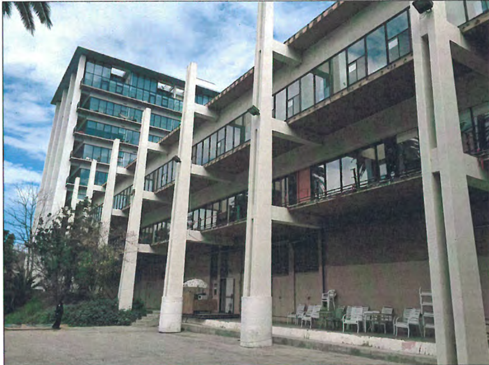
Figure 32: Building 3a, west elevation, view northeast (Snow, 2016)
