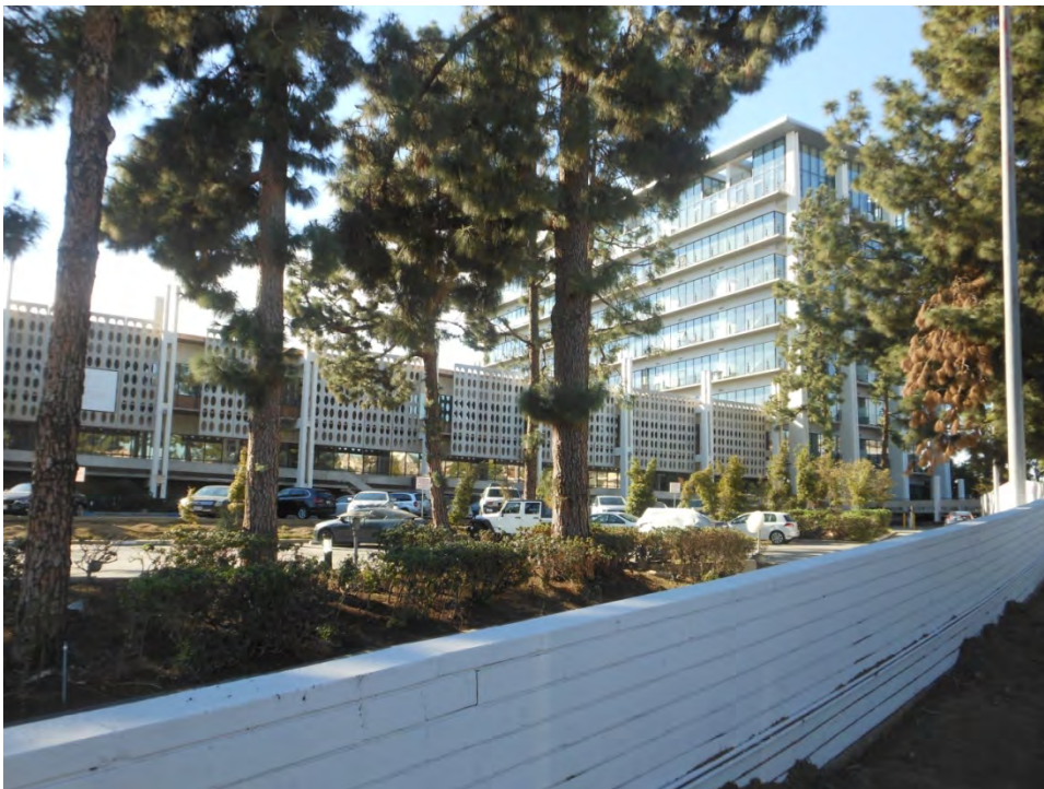
35. Metropolitan Water District Headquarters Campus, Original Building Alpine wing north elevation
