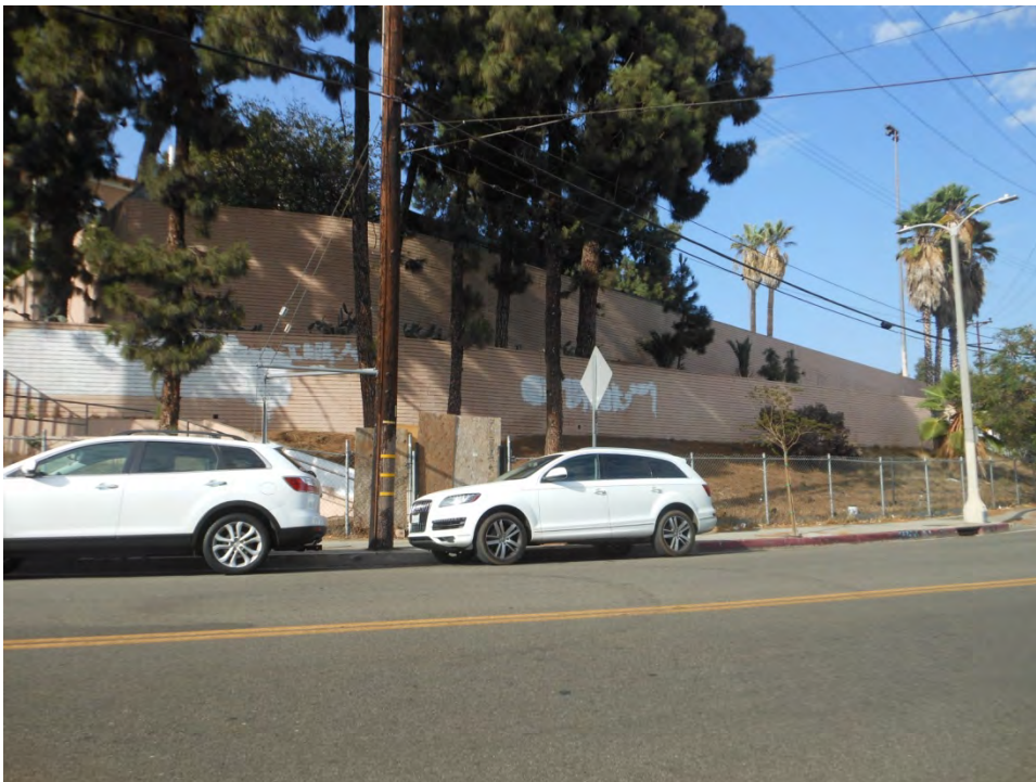
27. Retaining wall, Beaudry Avenue
