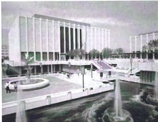
Overall view of LACMA at opening where the simple massing and strong vertical expression of structure is the primary feature.
