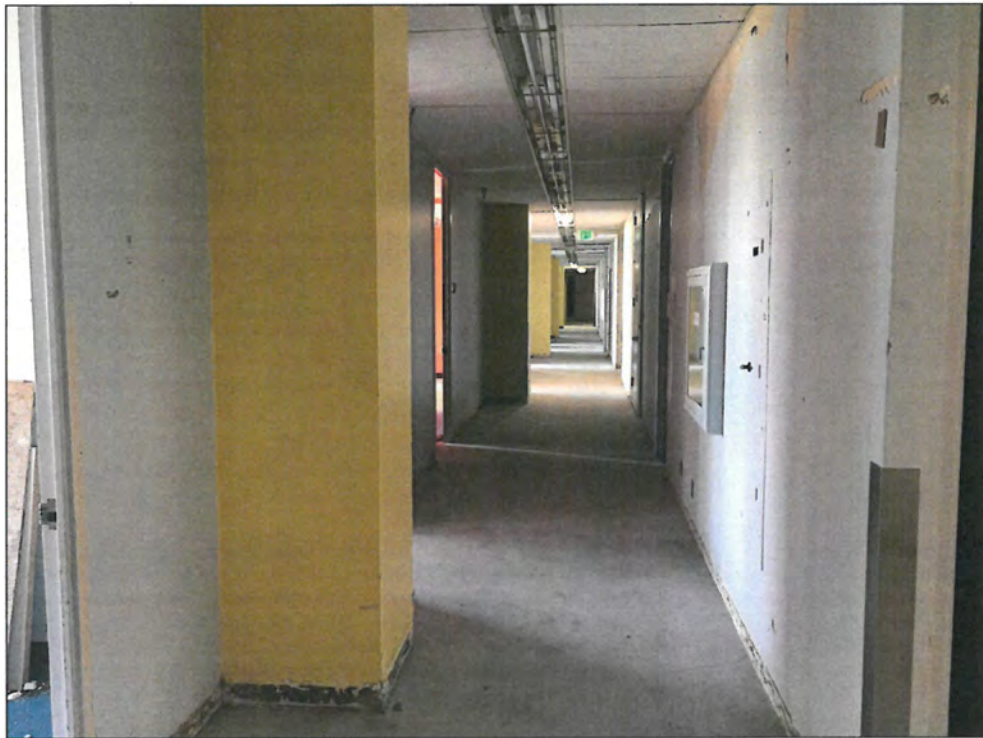
Figure 42: Building 3a and 3b, interior, typical corridor (Snow, 2016)
