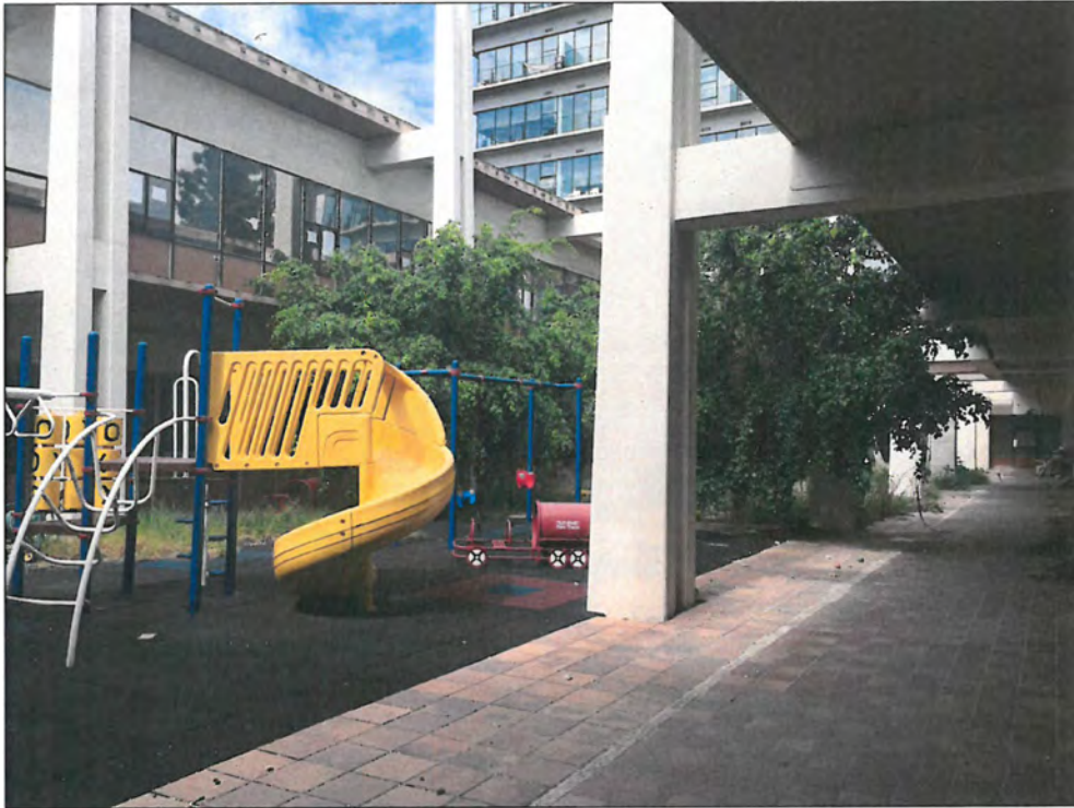
Figure 37: Building 3a and 3b, interior courtyard, view northwest (Snow, 2016)
