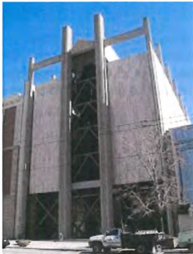
Prudential Building in Salt Lake City (demolished) had similar vertical pylons creating the overall design with infill of various kinds.
