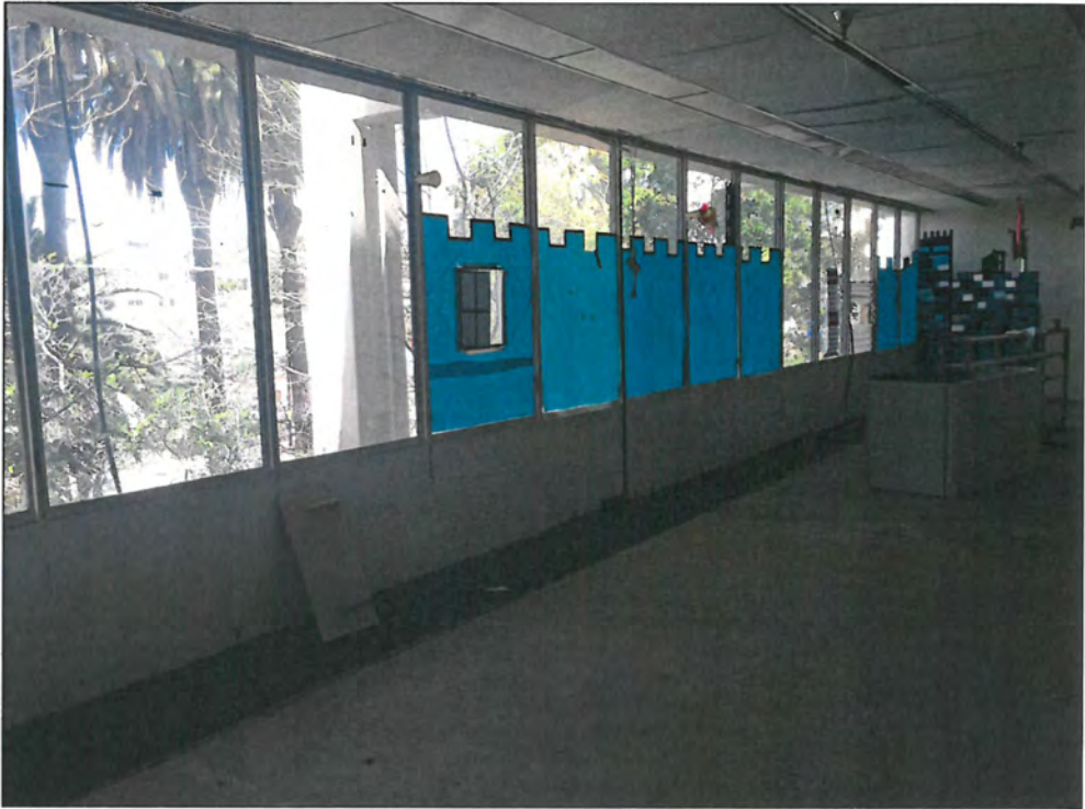
Figure 46: Building 3a and 3b, interior, typical office (Snow, 2016)
