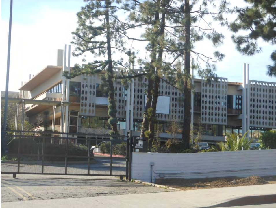
34. Metropolitan Water District Headquarters Campus, and Original Building Alpine wing east and north elevations
