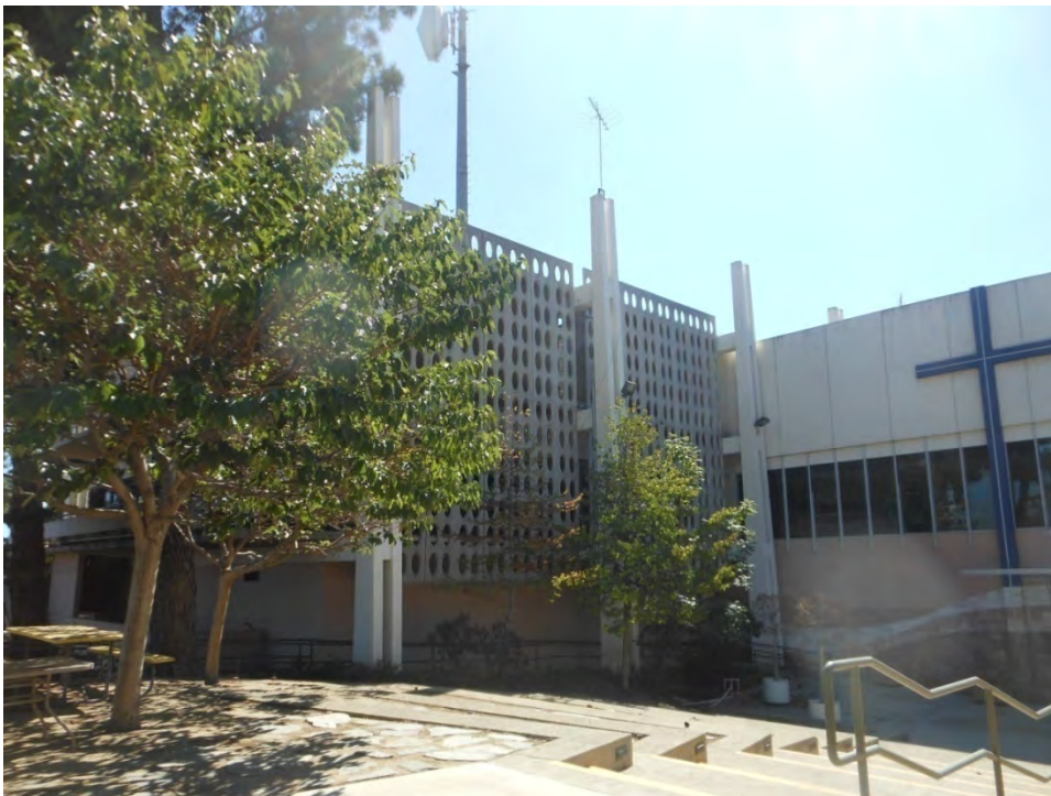
31. Metropolitan Water District Headquarters Campus, Original Beaudry Building, west elevation and Sanctuary Addition, north elevation
