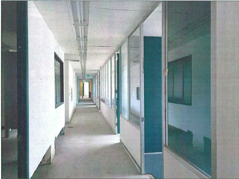
Figure 43: Building 3a and 3b, interior, typical corridor (Snow, 2016)
