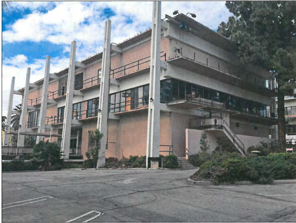
Figure 13: Building 1, south (left) and east (right) elevation, view northwest (Snow, 2016)
