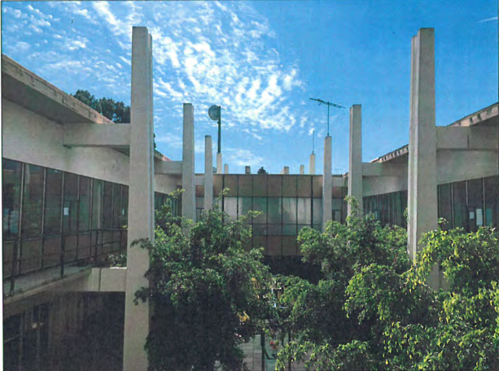
Figure 35: Building 3a and 3b, interior courtyard, view south (Snow, 2016)
