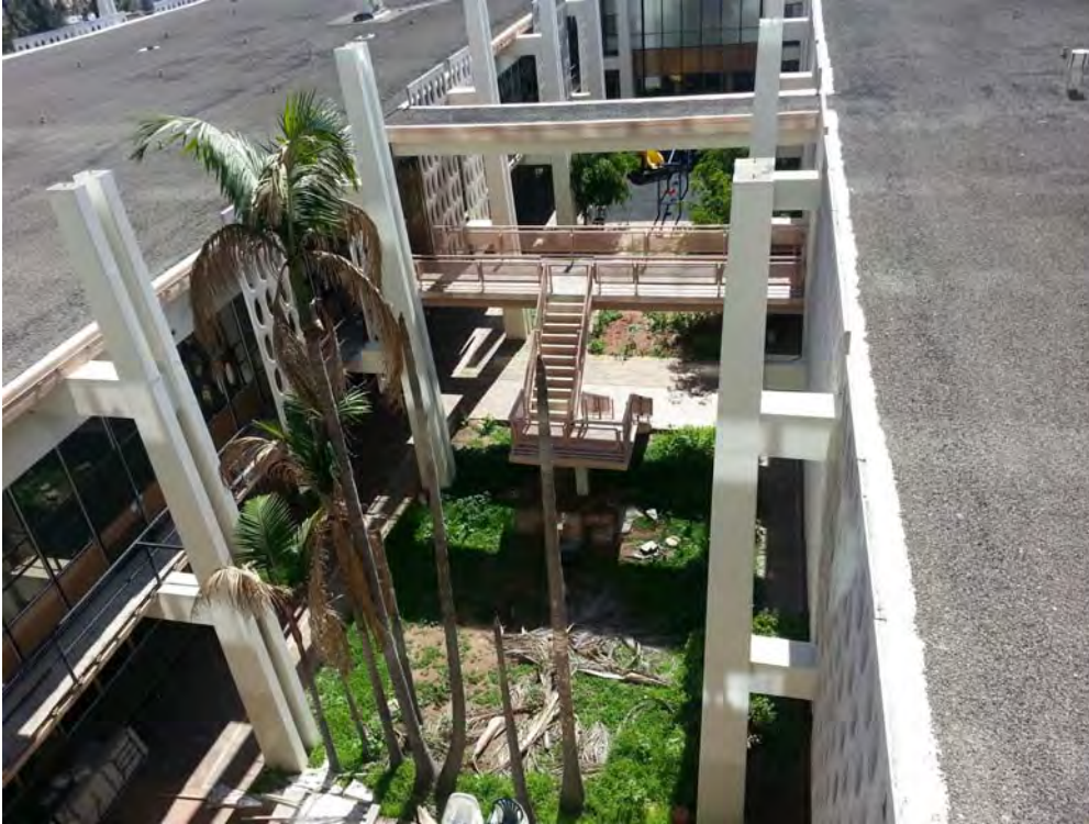
59. View of courtyard from Tower
