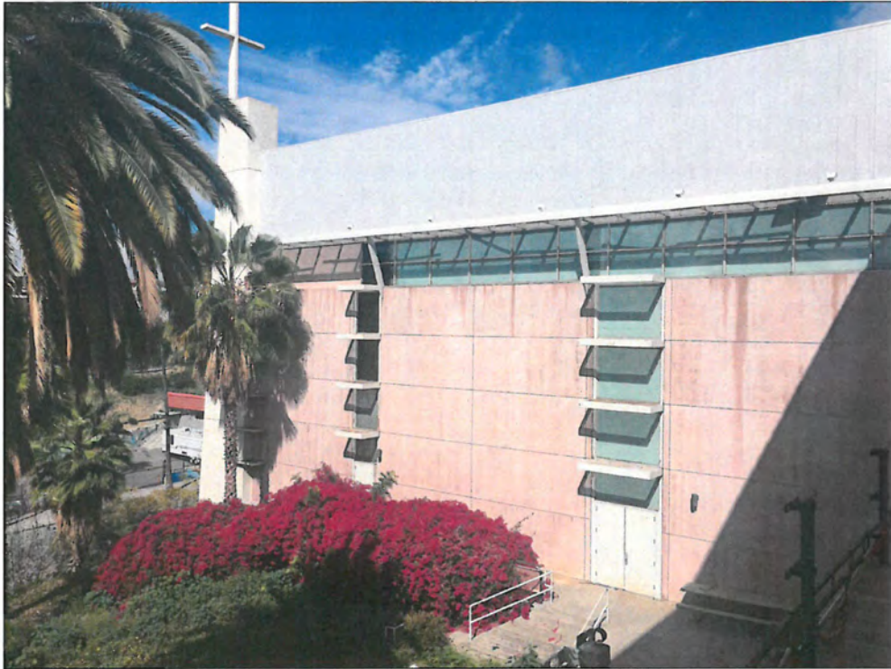
Figure 57: Building 5, south elevation, view northwest (Snow, 2016)
