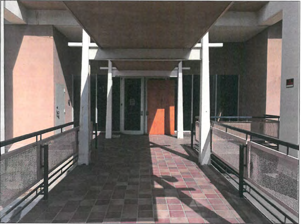
Figure 10 Building 1, south elevation, main entrance, view north (Snow, 2016)
