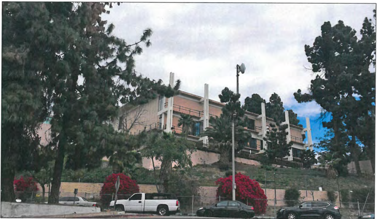
Figure 5: Subject property from North Beaudry Avenue, view north (Snow, 2016)
