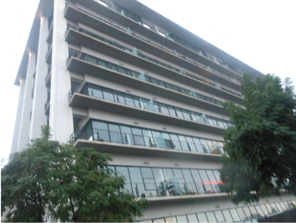
38. Metropolitan Water District Headquarters Campus, High Rise Building, west elevation
