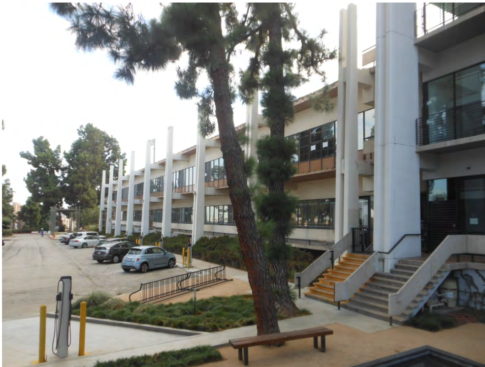
49. Metropolitan Water District Headquarters Campus, Original Alpine Building, north elevation and High Rise Building, north elevation (September 2015)
