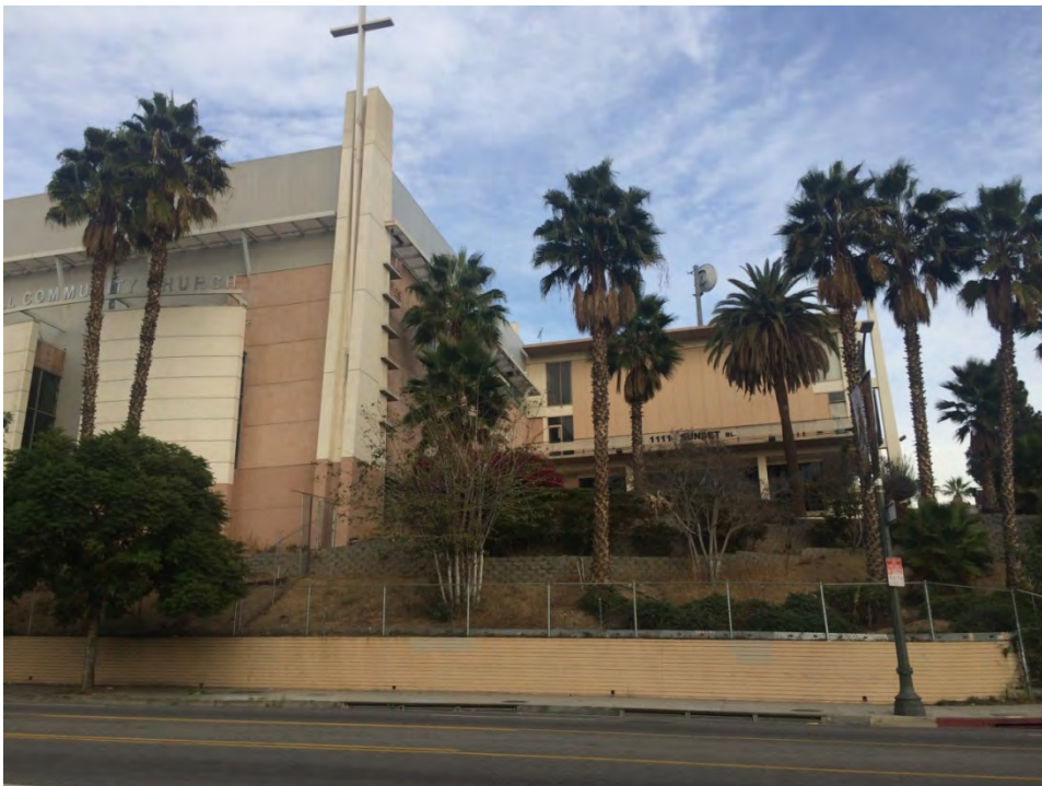
43. Metropolitan Water District Headquarters Campus, Original Building Sunset wing and Sanctuary Addition, south elevations
