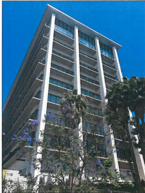
Figure 54: Building 4, west elevation, view southeast (Snow, 2016)
