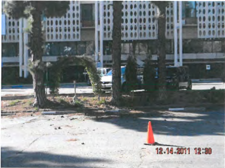
East Elevation – All original Pereira sunscreens and guard rails in first level in place
