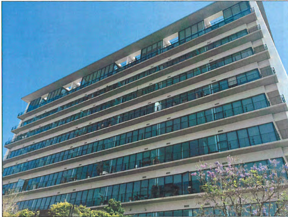
Figure 53: Building 4, north elevation, view southeast (Snow, 2016)
