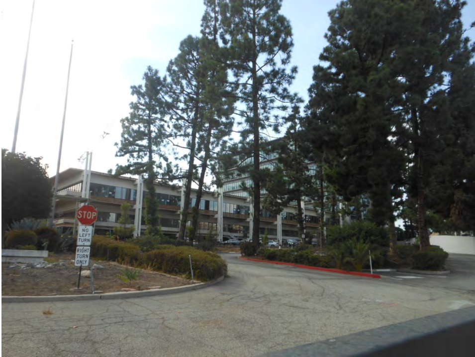
48. Metropolitan Water District Headquarters Campus, original Alpine Building, north elevation (September 2015)
