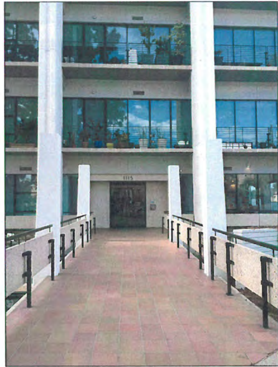
Figure 52: Building 4, east elevation, main entry, view west (Snow, 2016)
