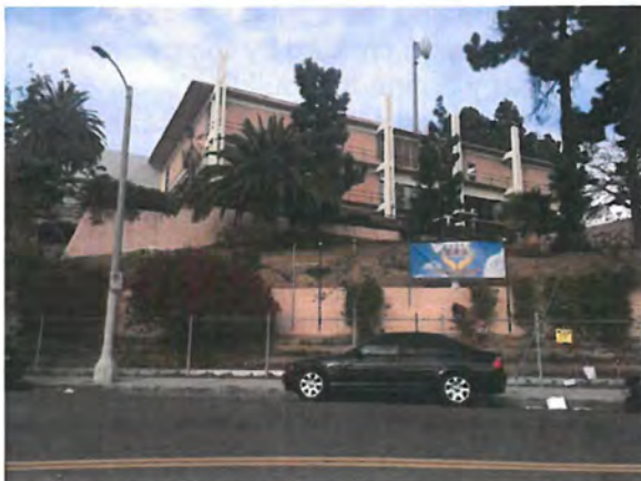
The building without decorative screens is still clearly a design by William Pereira.
