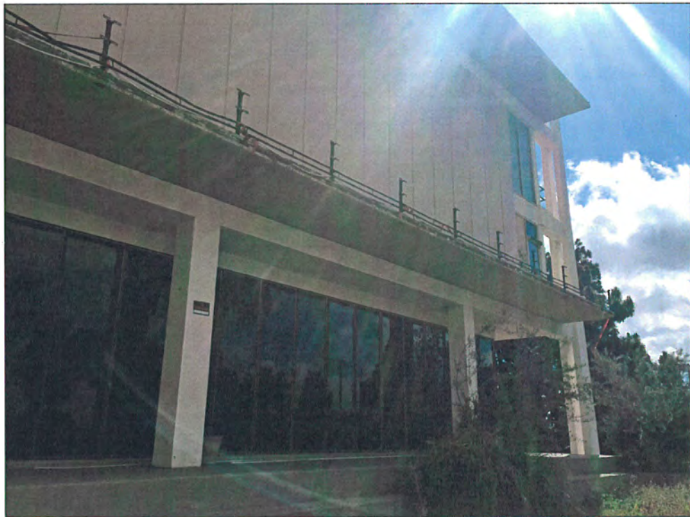
Figure 12: Building 1, west elevation, view southeast (Snow, 2016)
