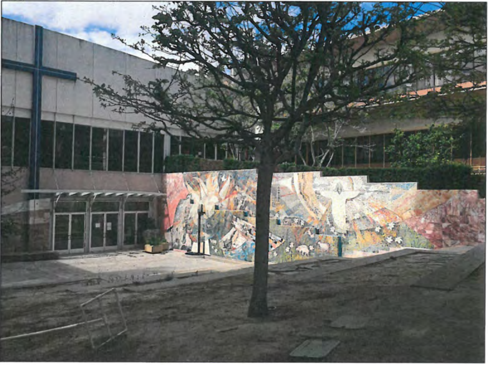
Figure 22: Building 2, east elevation, view northwest (Snow, 2016)
