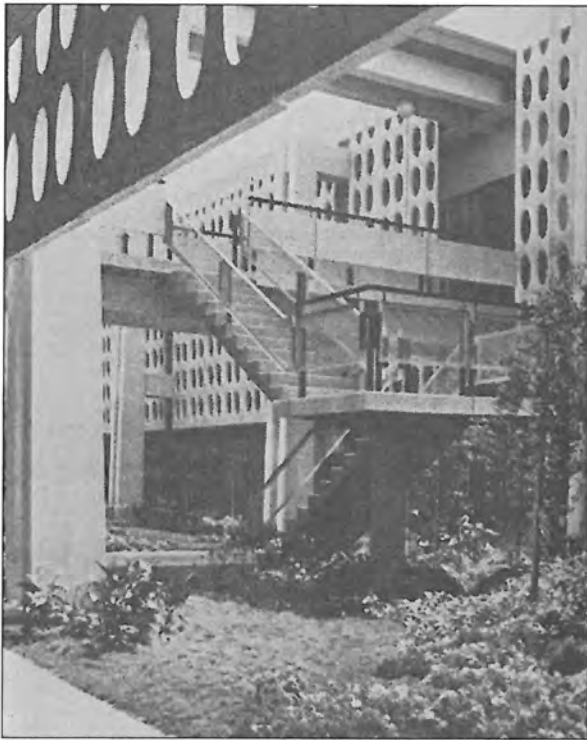
Historic Photograph 24: Building 3a and 3b, interior courtyard, compare with Figure 38 (1963, MWD Annual Report) 1111 Sunset Boulevard, Los Angeles, CA
