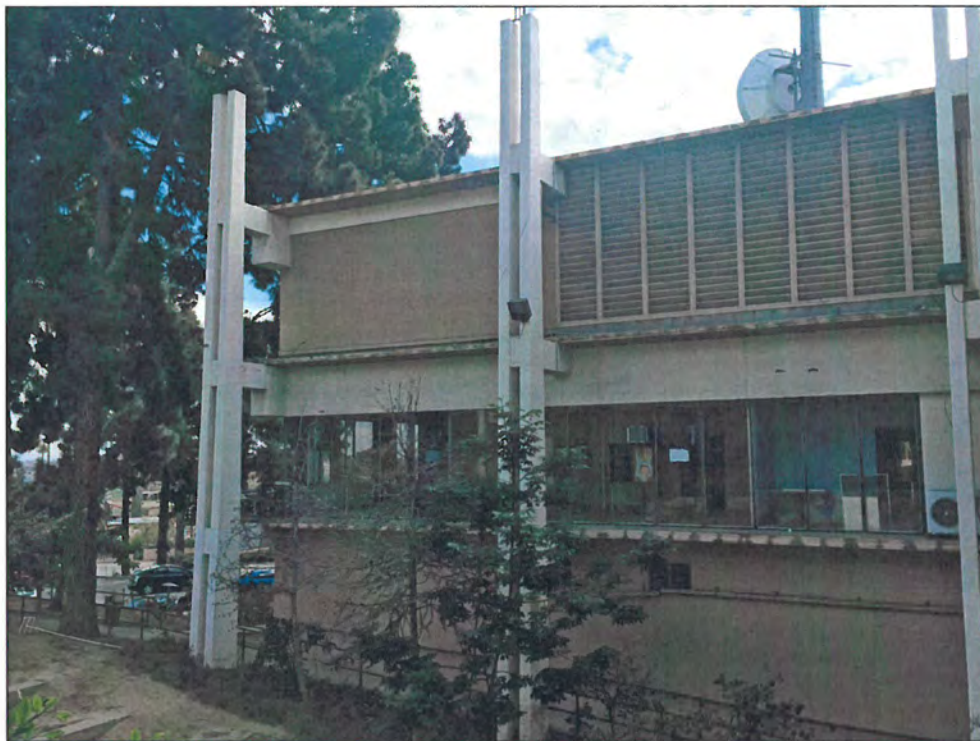
Figure 16: Building 1, north elevation, view southeast (Snow, 2016)
