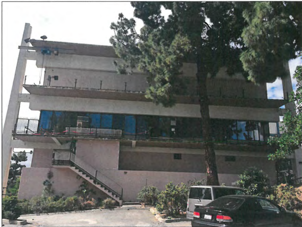
Figure 14: Building 1, east elevation, view west (Snow, 2016)
