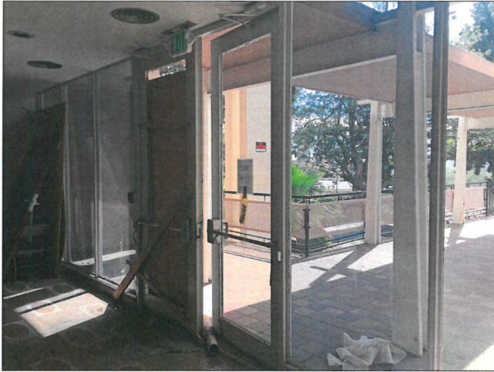
Figure 17: Building 1, interior, main entrance at south elevation, view southeast (Snow, 2016)
