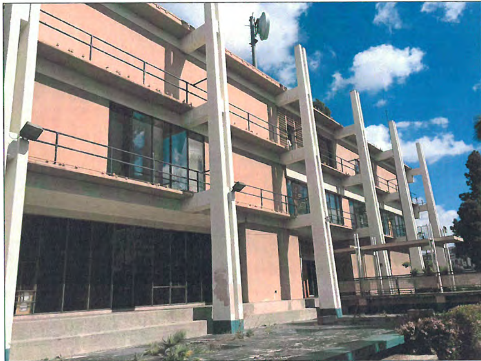
Figure 8: Building 1, south elevation, view northeast (Snow, 2016)
