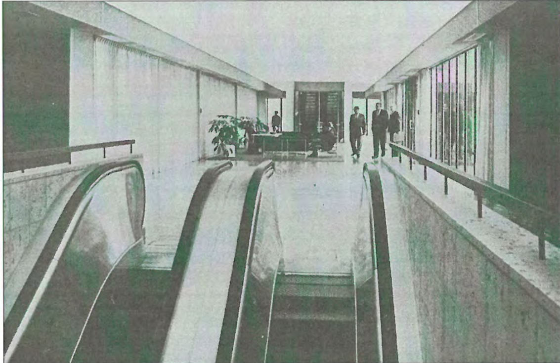
Historic Photograph 27: Building 2, interior, view north (1963, MWD Annual Report, caption reads, "View of the lobby with the escalators to the cafeteria in the foreground.")
