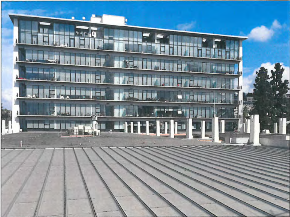
Figure 49: Building 4, south elevation, view north from roof of Building 3 (Snow, 2016)
