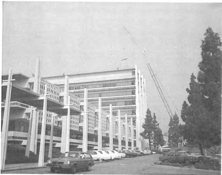
Figure 7: Annex completing construction, south elevation, view northwest, note ribbon windows, rather than floor to ceiling windows (MWD Archives, 1973)
