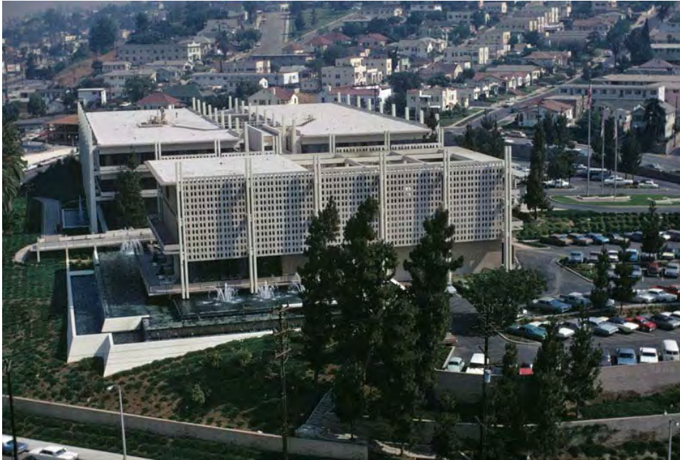
11. Metropolitan Water District Headquarters Campus, Original Beaudry Building and Original Building Sunset wing, looking east, c. 1962
