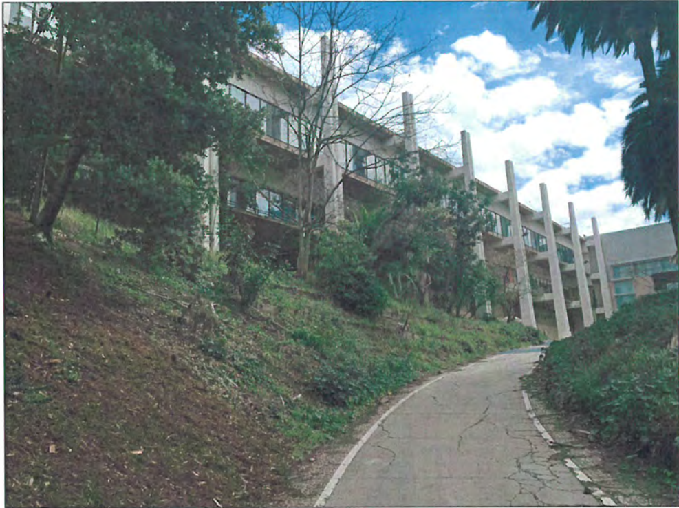
Figure 31: Building 3a, west elevation, view southeast (Snow, 2016)
