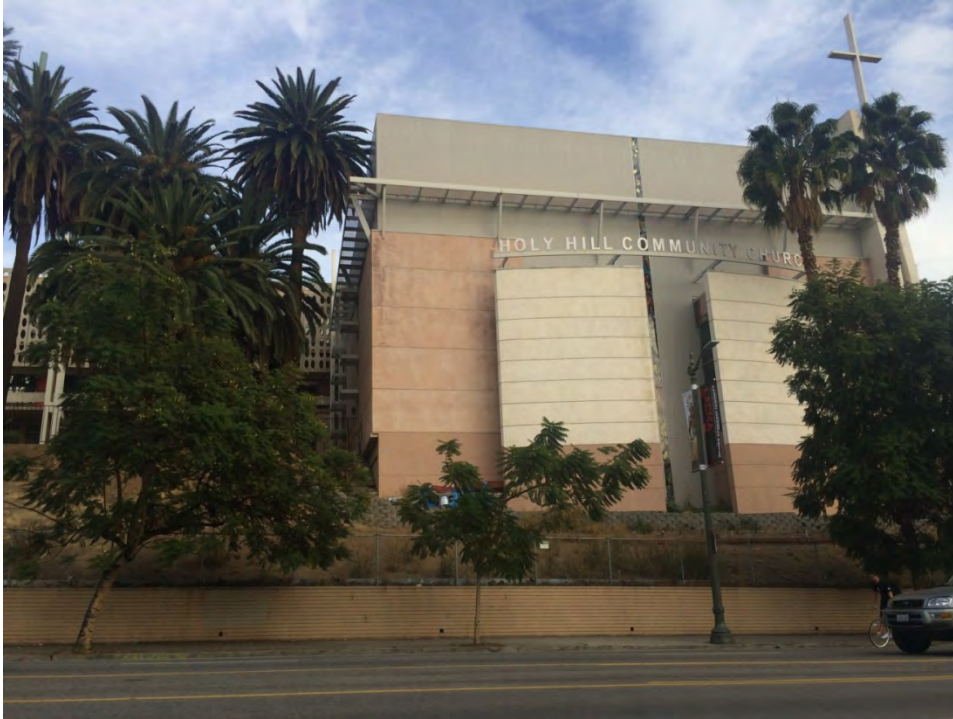
42. Metropolitan Water District Headquarters Campus, Original Building Sunset wing, mid-section of south elevation
