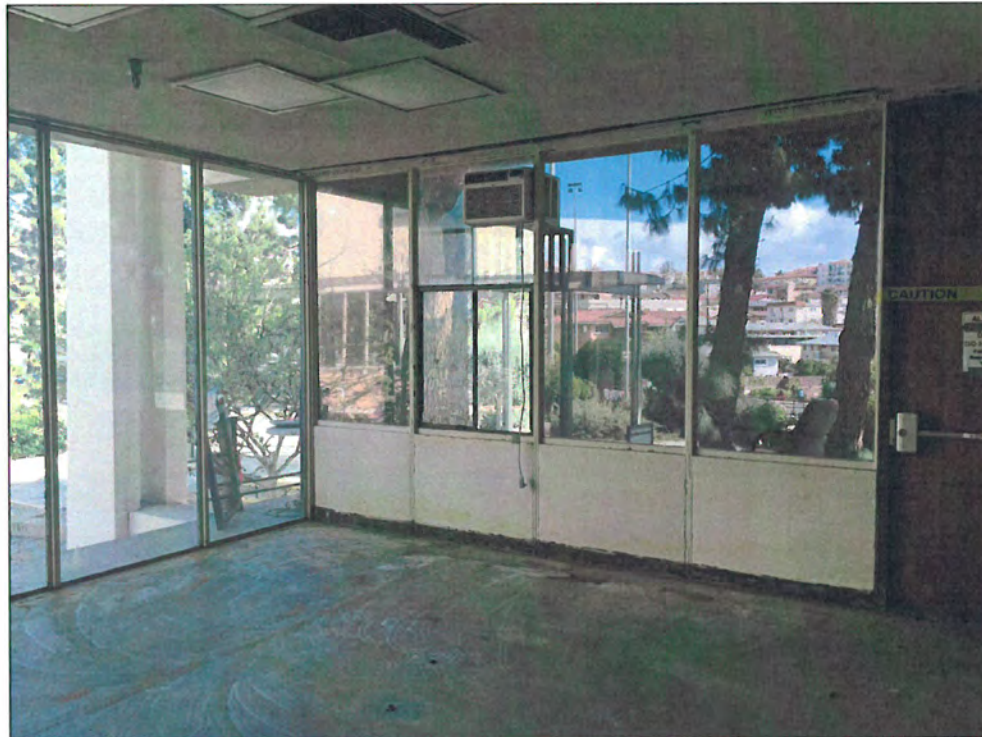
Figure 20: Building 1, interior, typical second floor office space, view southeast (Snow, 2016)
