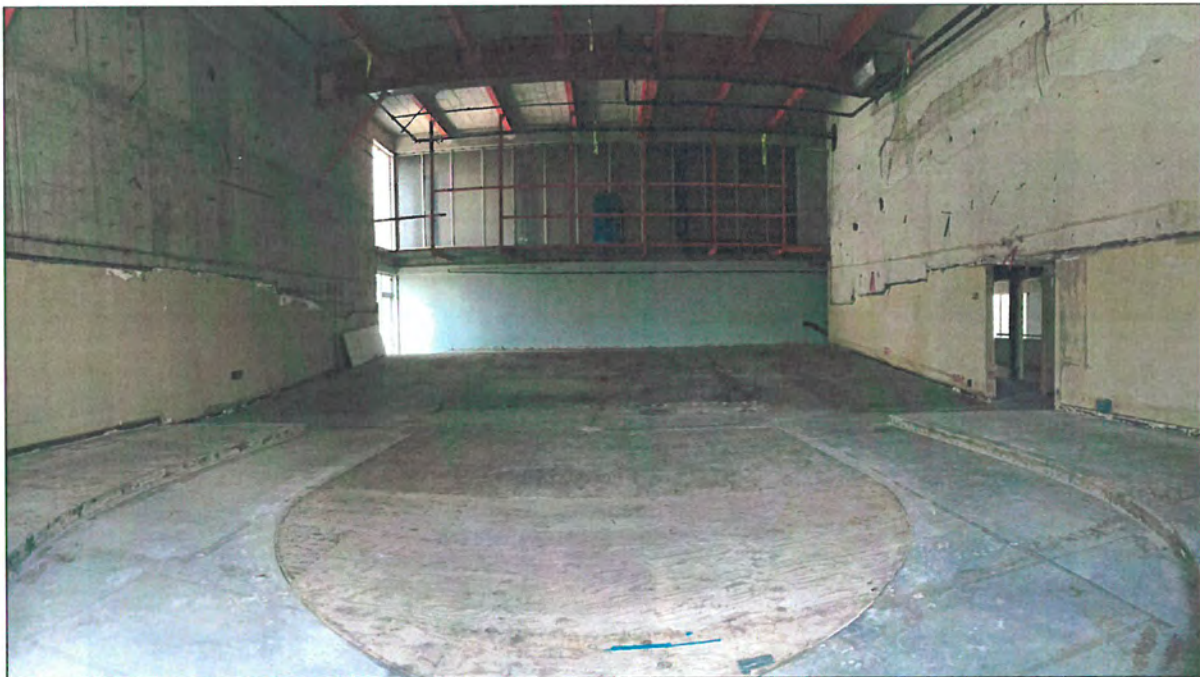
Figure 19: Building 1, interior, board room, compare with Historic Photograph 14, view north (Snow, 2016)
