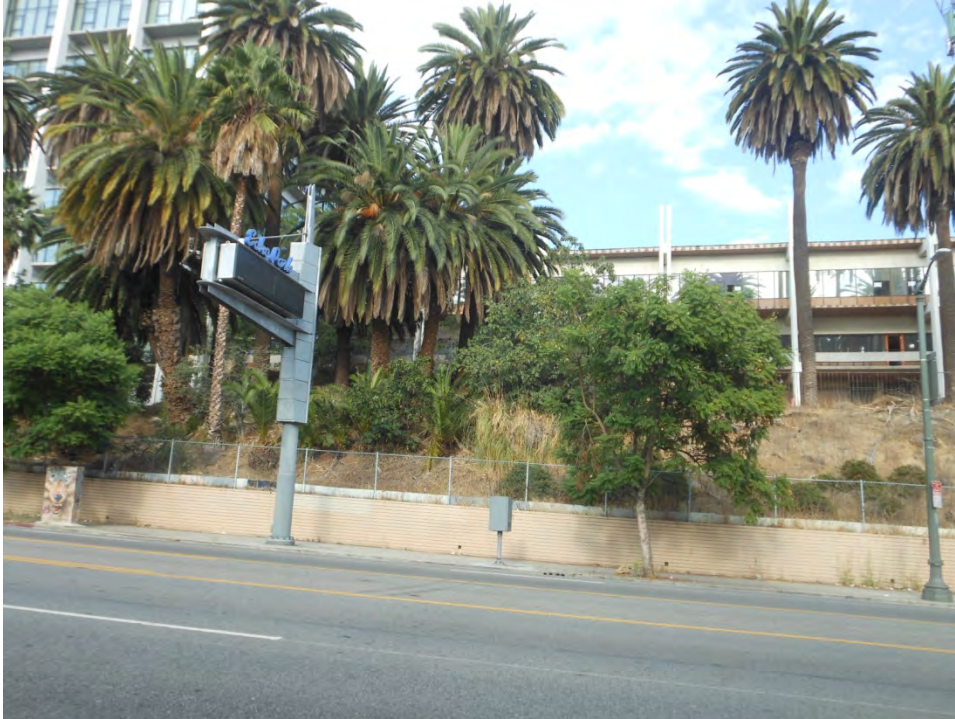
52. Metropolitan Water District Headquarters Campus, Original Sunset Building, south elevation (September 2015)
