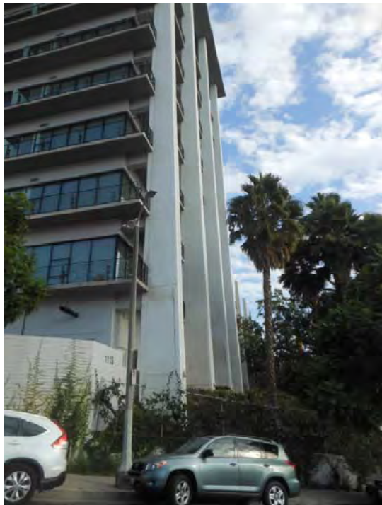
51. Metropolitan Water District Headquarters Campus, High Rise Building, west and south elevations (September 2015)
