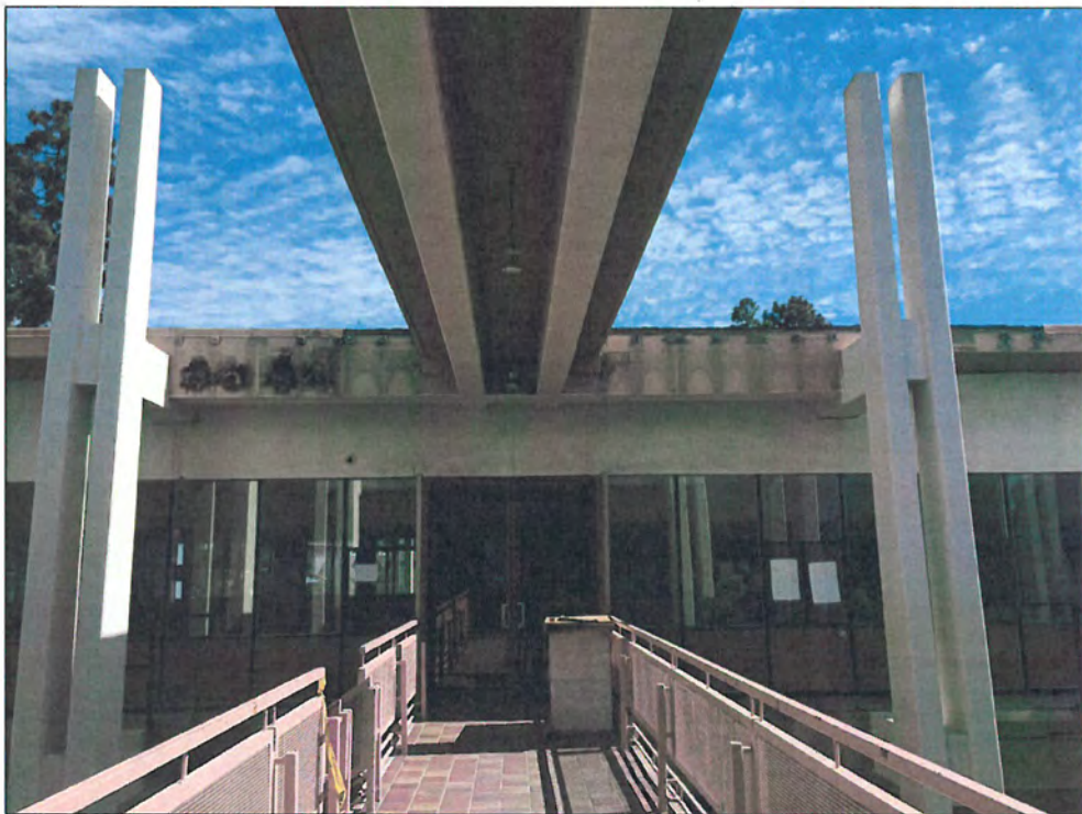
Figure 40: Building 3a and 3b, bridge between two wings spanning courtyard, view east (Snow, 2016)
