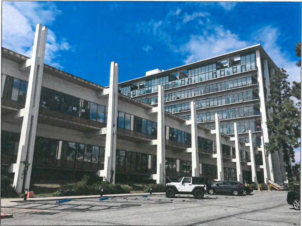
Figure 29: Building 3b, east elevation, view northwest (Snow, 2016)
