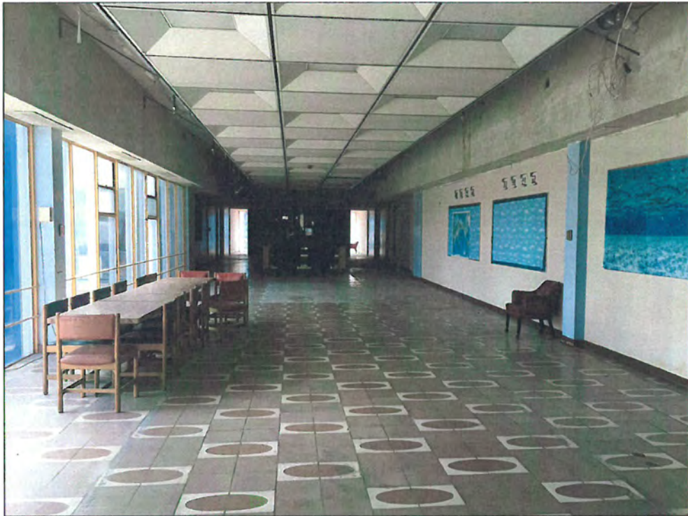
Figure 27: Building 2, interior, second floor corridor, view south (Snow, 2016)
