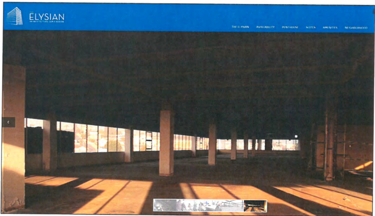
Figure 9: Annex prior to renovation, note two-part window systems with a solid lower panel, ( http://theelysian.la/ , c. 2012)
