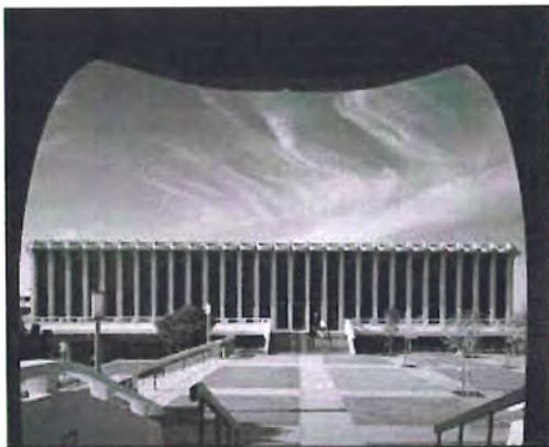
Building at UC Irvine with simple strong vertical expression of structure.
