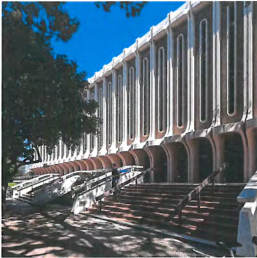
Building at UC Irvine with prominent vertical structural expression of pylons.
