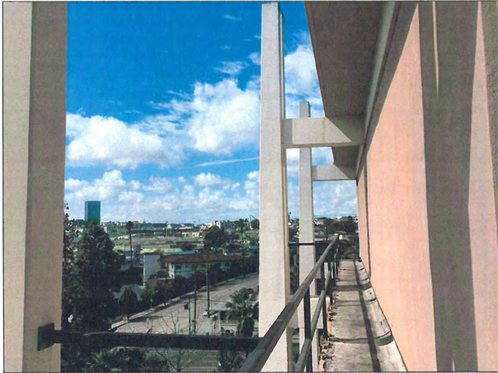
Figure 11: Building 1, south elevation, balcony at second floor view west (Snow, 2016)
