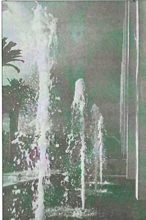
Historic Photograph 22: Building 3a west elevation, view north (1963, MWD Annual Report, caption reads, "Fountains at the new Headquarters Building symbolize the all important function of The Metropolitan Water District...to provide ample supplemental water for more than 8,500,000 people.") 1111 Sunset Boulevard, Los Angeles, CA
