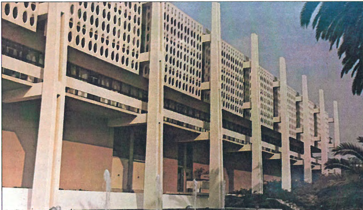
Historic Photograph 36: Building 3a, west elevation, view southeast (1966, MWD Annual Report)
