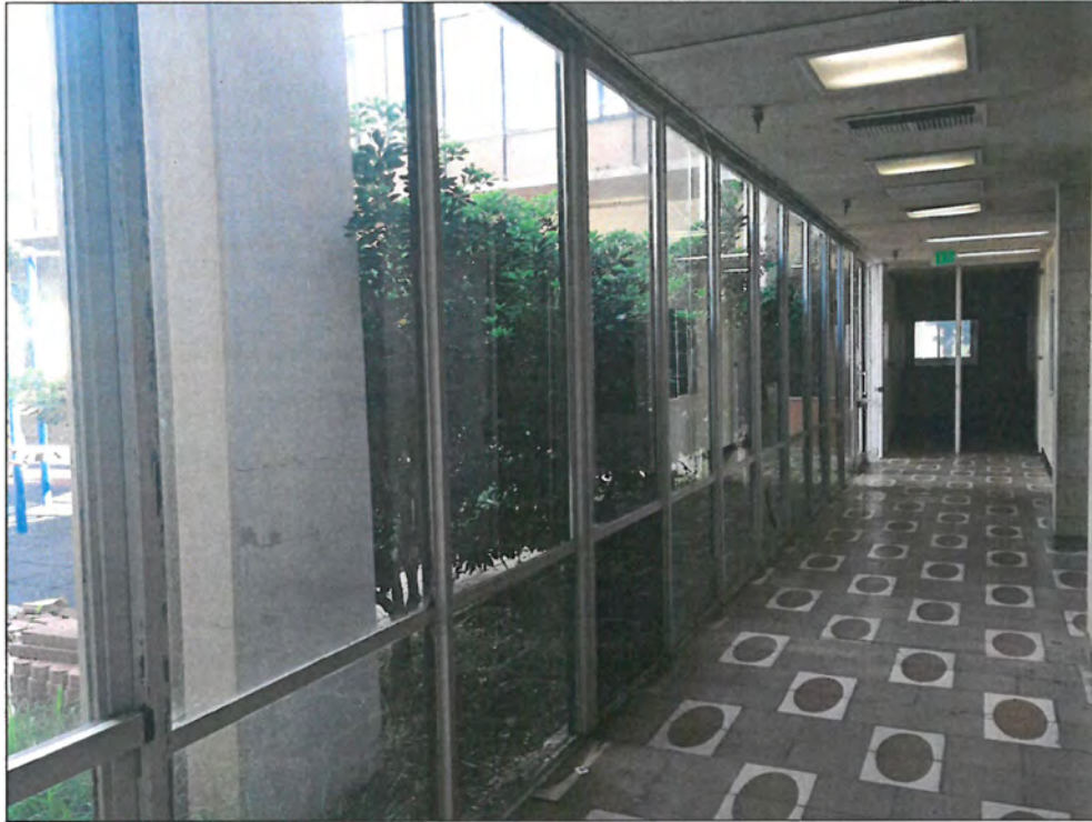
Figure 41: Building 3a and 3b, interior, corridor along south elevation, view east (Snow, 2016)
