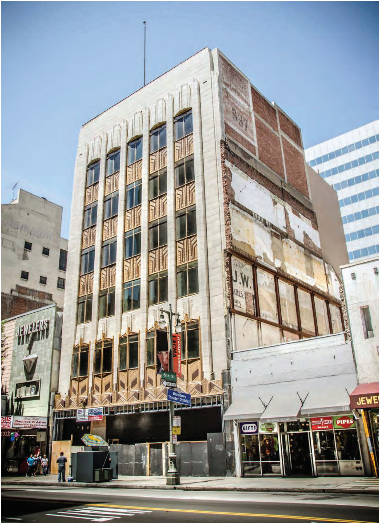
F & W Grand Silver Building, 537-41 S. Broadway, May 20, 2013 (Photograph from Curbed LA)
