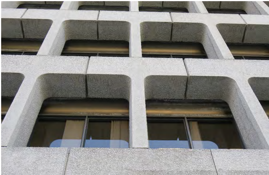
Close-up of upper floors and granite aggregate cladding at the north façade, view south (ARG, 2017).
