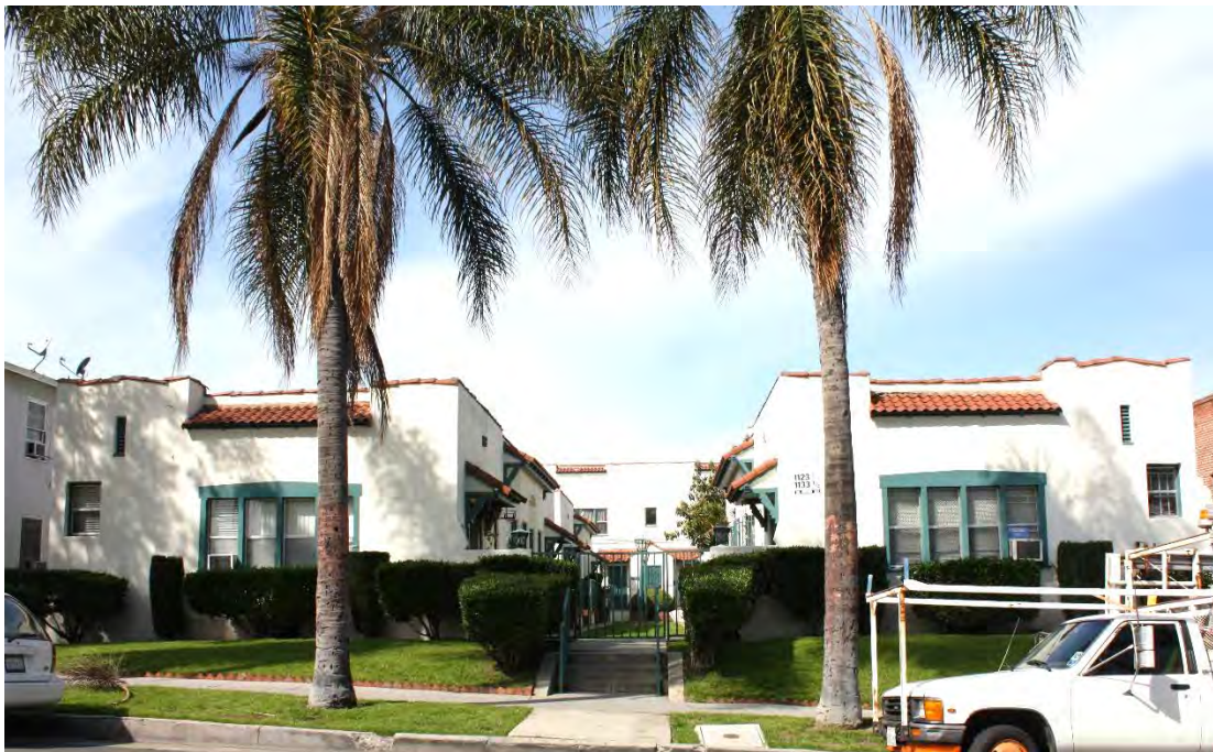
1123 – 1133 South Norton Ave, protected by Country Club Park HPOZ, 1923, William F. Bowen, architect.
