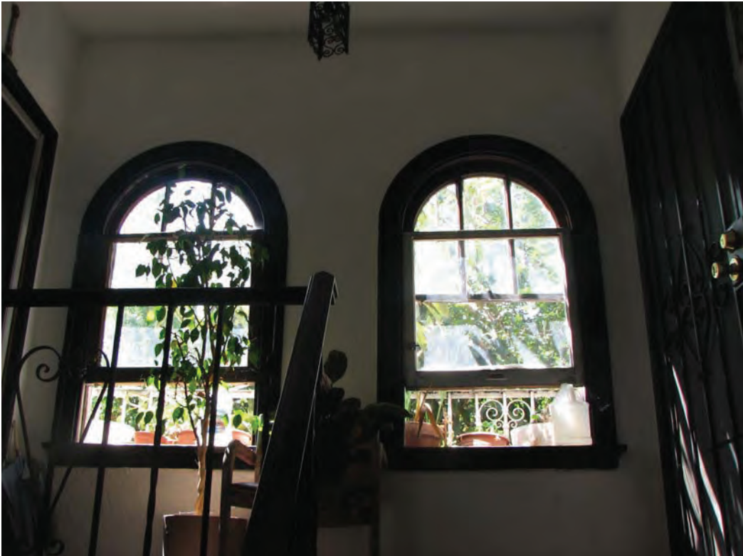
Norton Flats, arched windows, 412-420 N. Norton Avenue, August 27, 2015 (Photograph by Charles J. Fisher)
