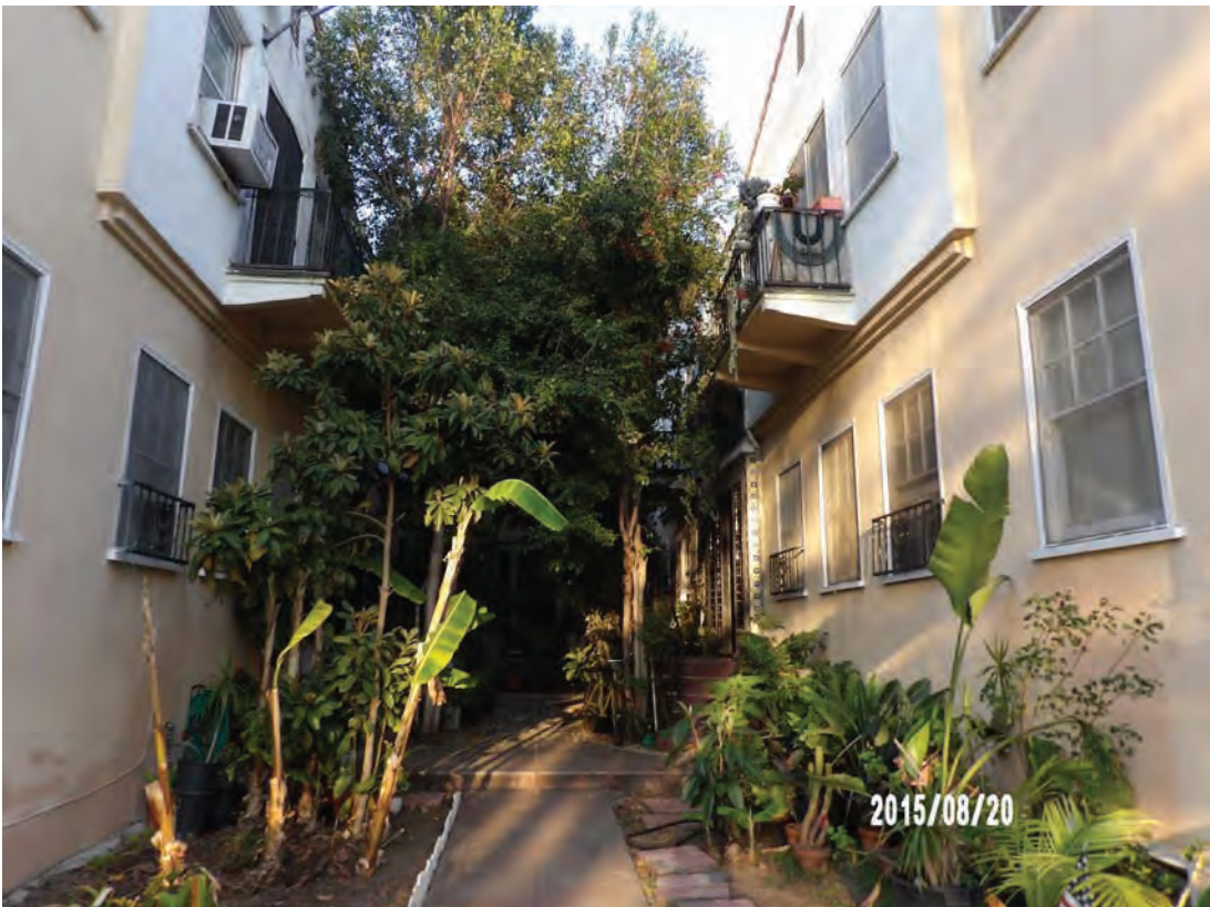
Norton Flats, courtyard, 412-420 N. Norton Avenue, August 20, 2015 (Photograph by Carlos Miranda)
