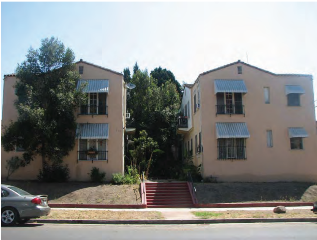
Norton Flats, 412-420 N. Norton Avenue, August 27, 2015 (Photograph by Charles J. Fisher)
