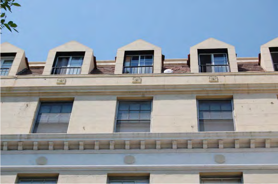
Detail of dormers across front parapet; windows are to former maid's rooms
