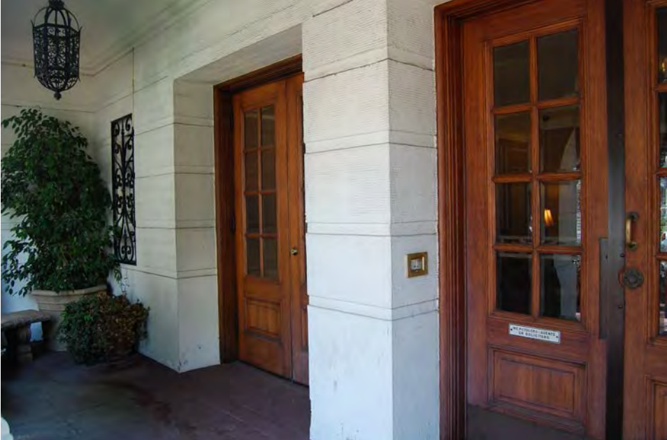
Original French doors at building entry to lobby, facing south
