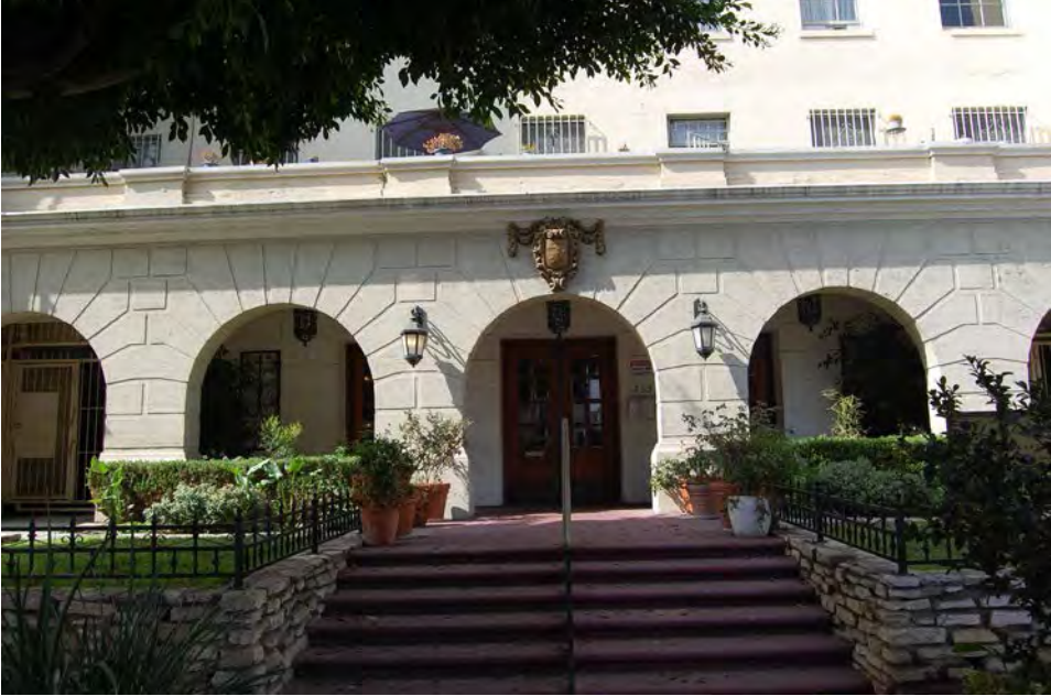
Detail of street entrance loggia, east (front) façade; also showing original garden retaining wall
