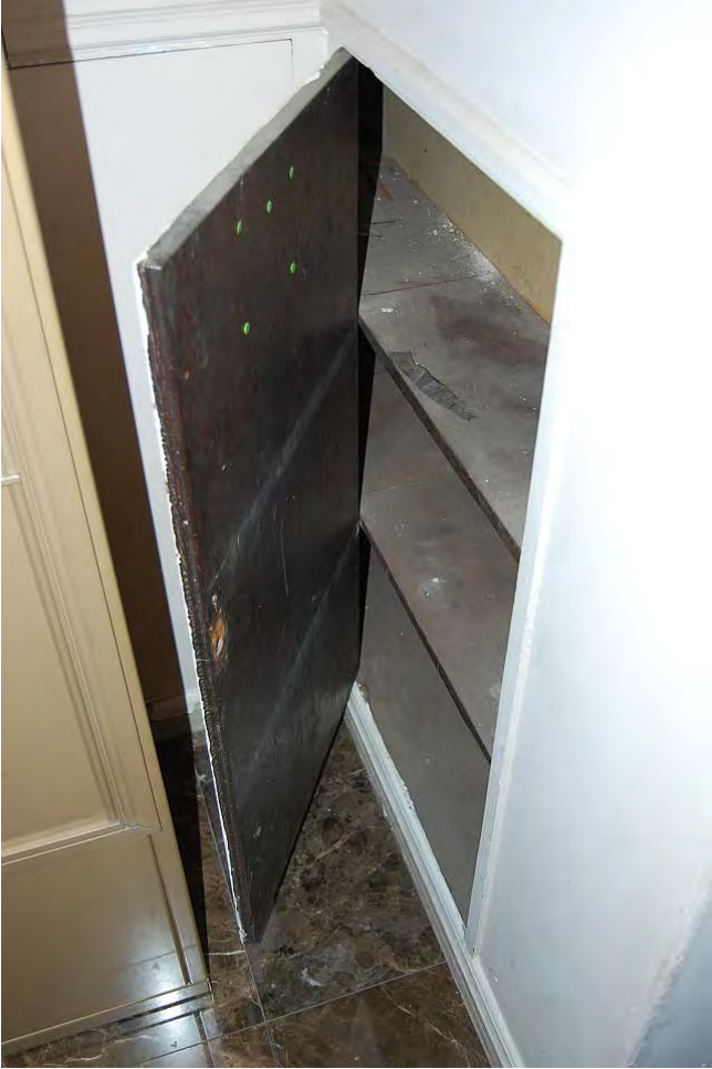
Original built-in closet behind lobby
