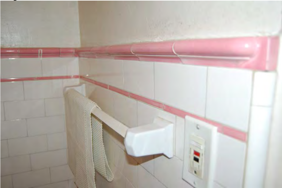
Original bathroom tile
