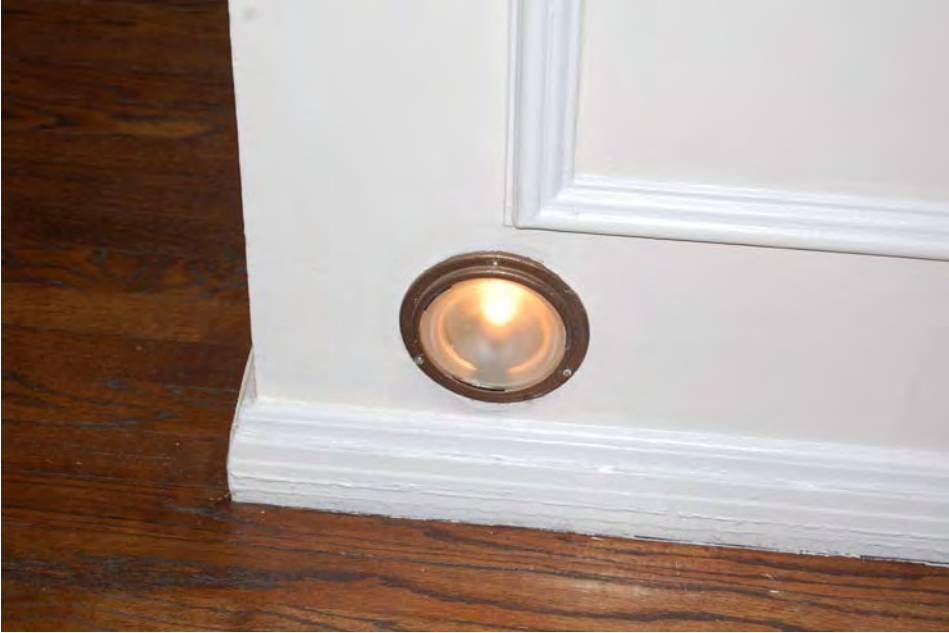
Detail showing original built-in night-light
