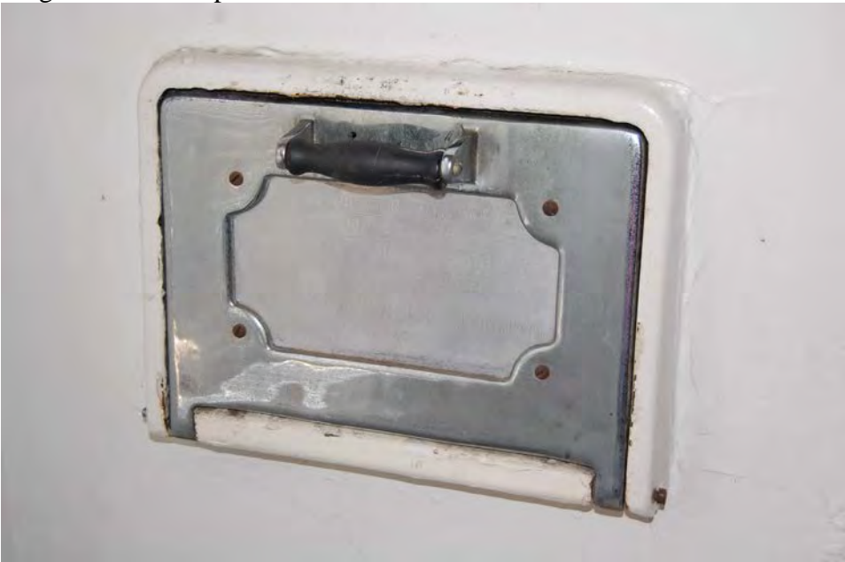
Original trash compactor door
