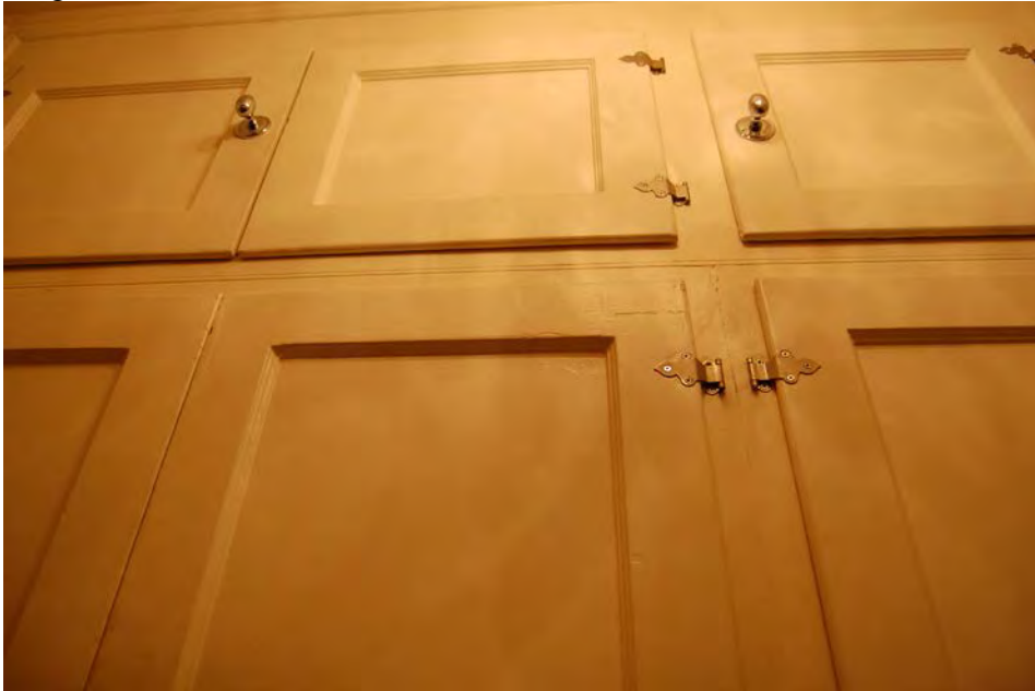
Original built-in linen closet
