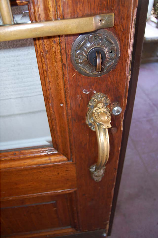
Original front door handle and lock
