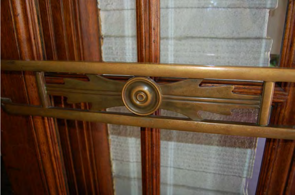
Original interior bronze door push on front doors, detail
