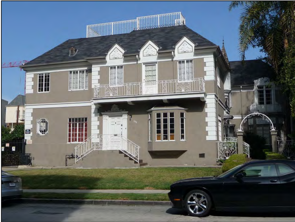
Primary (west) façade with courtyard to south, view northeast (ARG, 2017).
