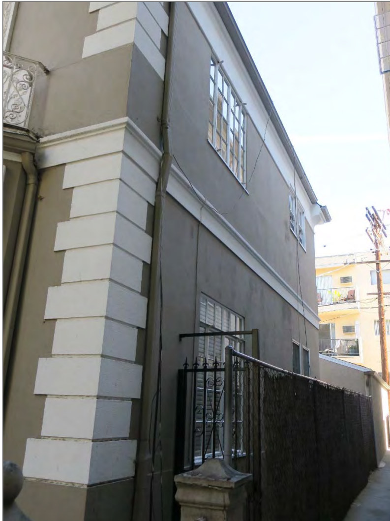
South façade, view to northeast (ARG, 2017)
