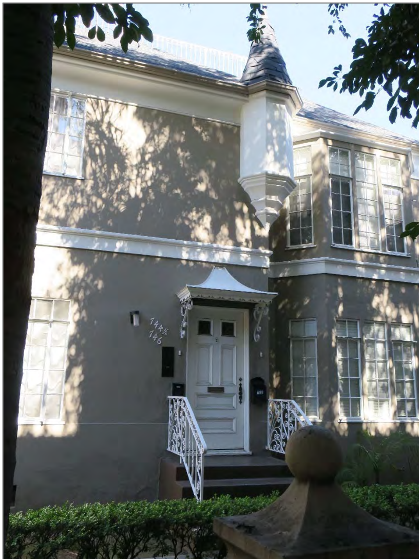
Courtyard unit entry and turret on south façade, view to northeast (ARG, 2017).
