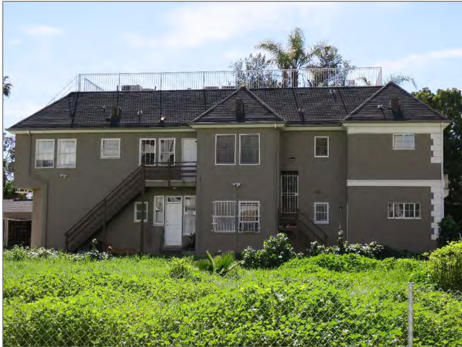
North façade, view south (ARG, 2017).
