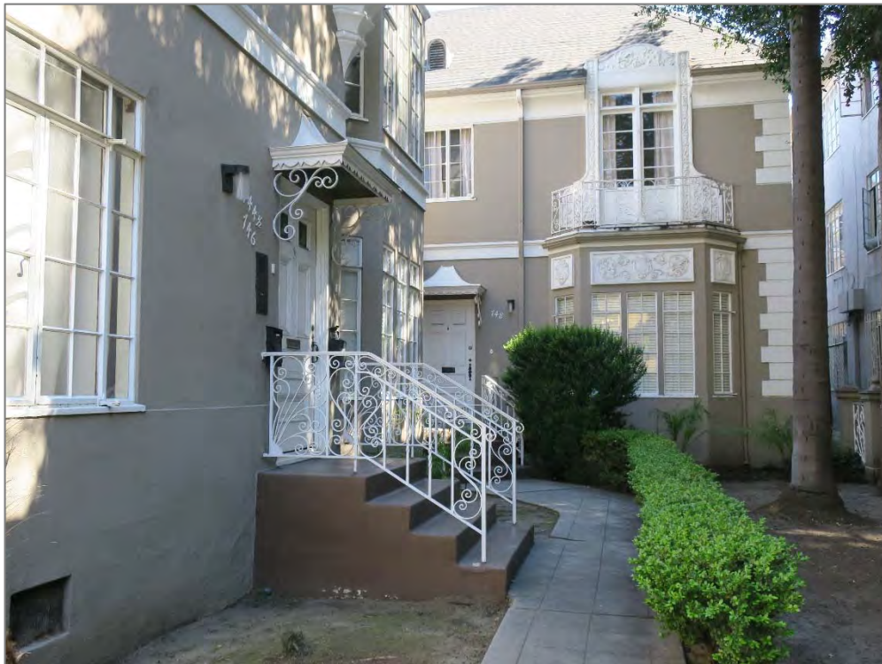
South and west courtyard façades, view to northeast (ARG, 2017).
