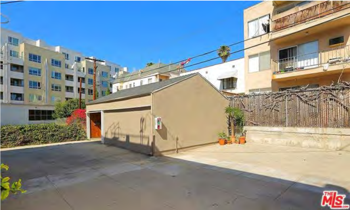
Garage at southeast of parcel, view southeast. Note: Condition of pavement. Photograph courtesy of the MLS, July 2015.
