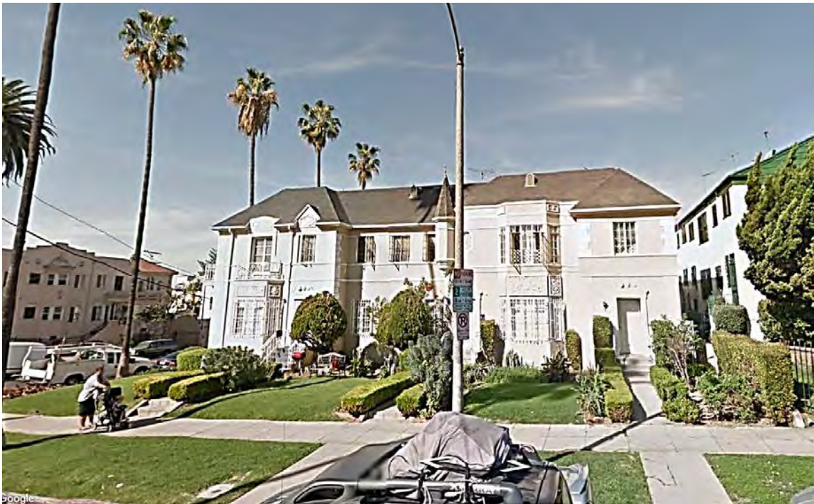
104 N. Catalina Street, from Google, at the corner of 1 st Street and Catalina Street, view west.
