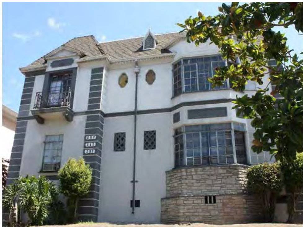
HCM 1115: The Altman Apartments, 412 South Catalina Street, view east.
