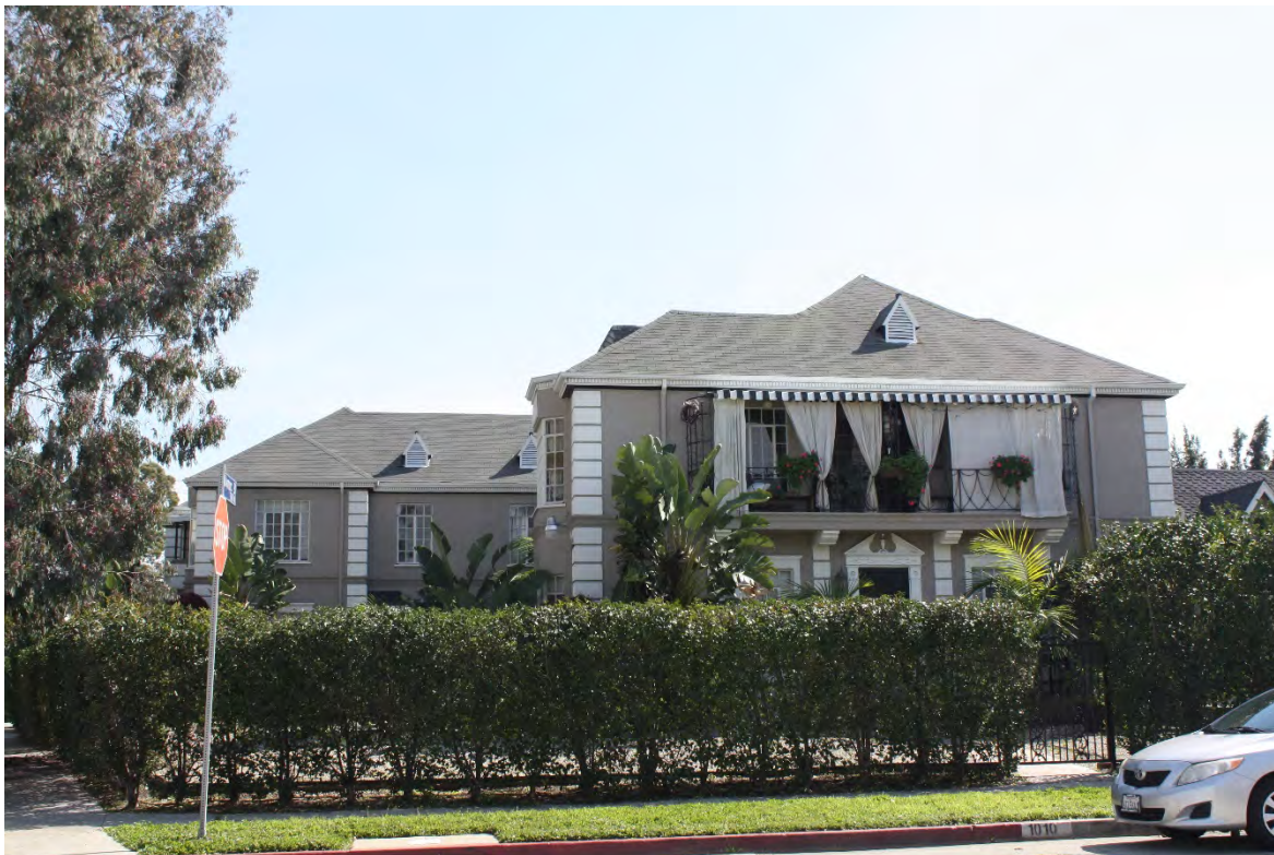
1000 S. Dunsmuir Avenue, view east. Photograph: Anna Marie Brooks, March 2017.
