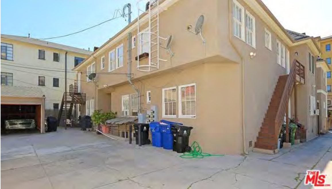
One of two garages, this one at south; Rear/east elevation; north elevation; driveway. Note: Condition of pavement. Photograph courtesy of the MLS, July 2015.
