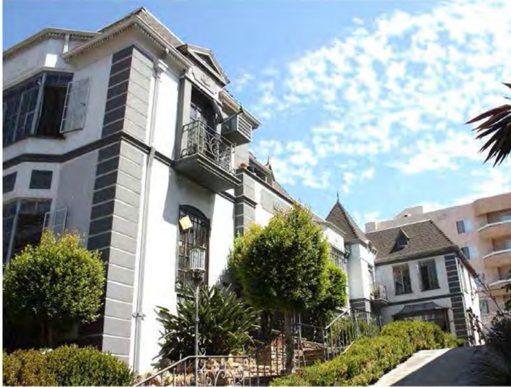
HCM 1115: The Altman Apartments, 412 South Catalina Street, view northeast.
