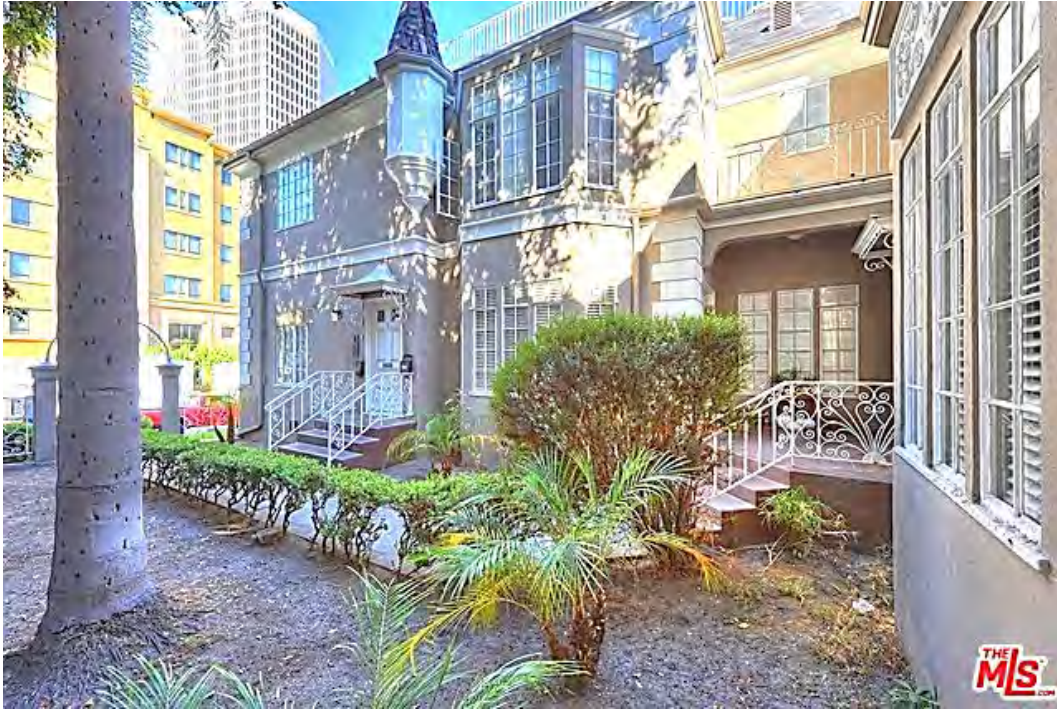
View lengthwise of courtyard, view northwest. Photograph courtesy of the MLS 2016.
