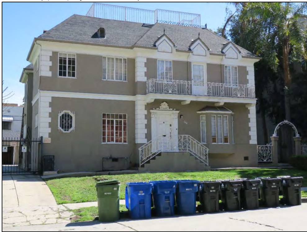
Primary (west) façade, view southeast (ARG, 2017).
