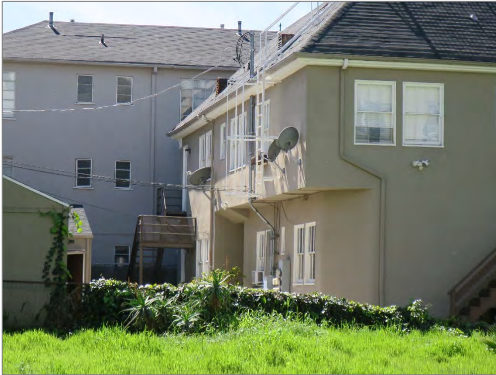
East and portion of north façades, view southwest (ARG, 2017).
