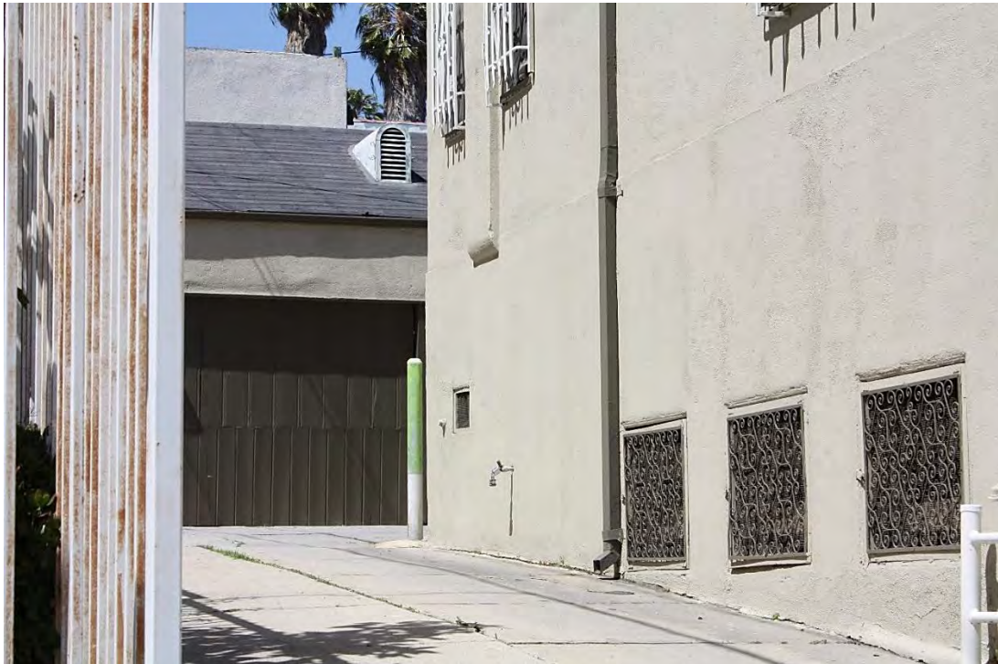
Driveway from 1 st St. to garages at north of building, view north. Photograph: Anna Marie Brooks, May 2017.
