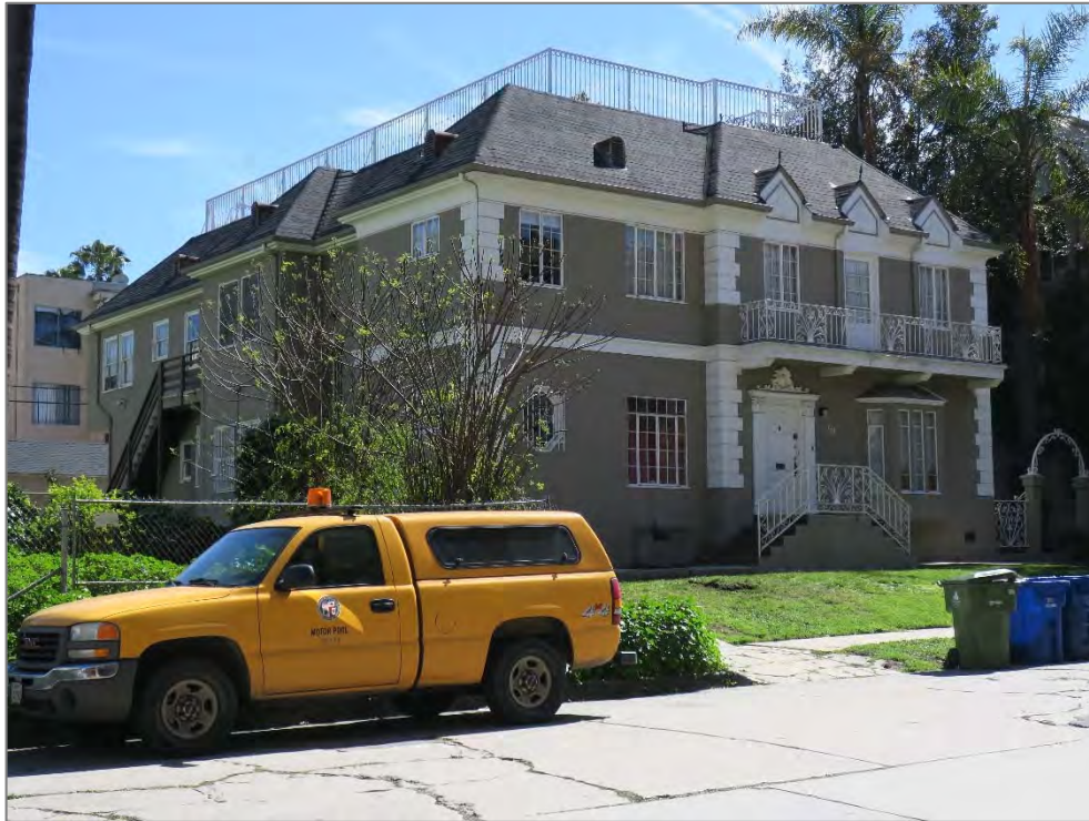
Primary (west) and north façades, view southeast (ARG, 2017).
