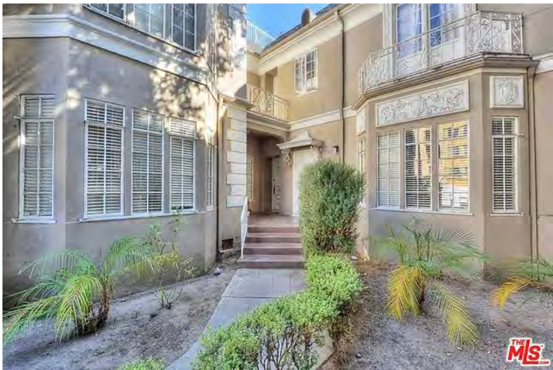
View into northeast entries from courtyard, northeast. Photograph courtesy of the MLS 2016.
