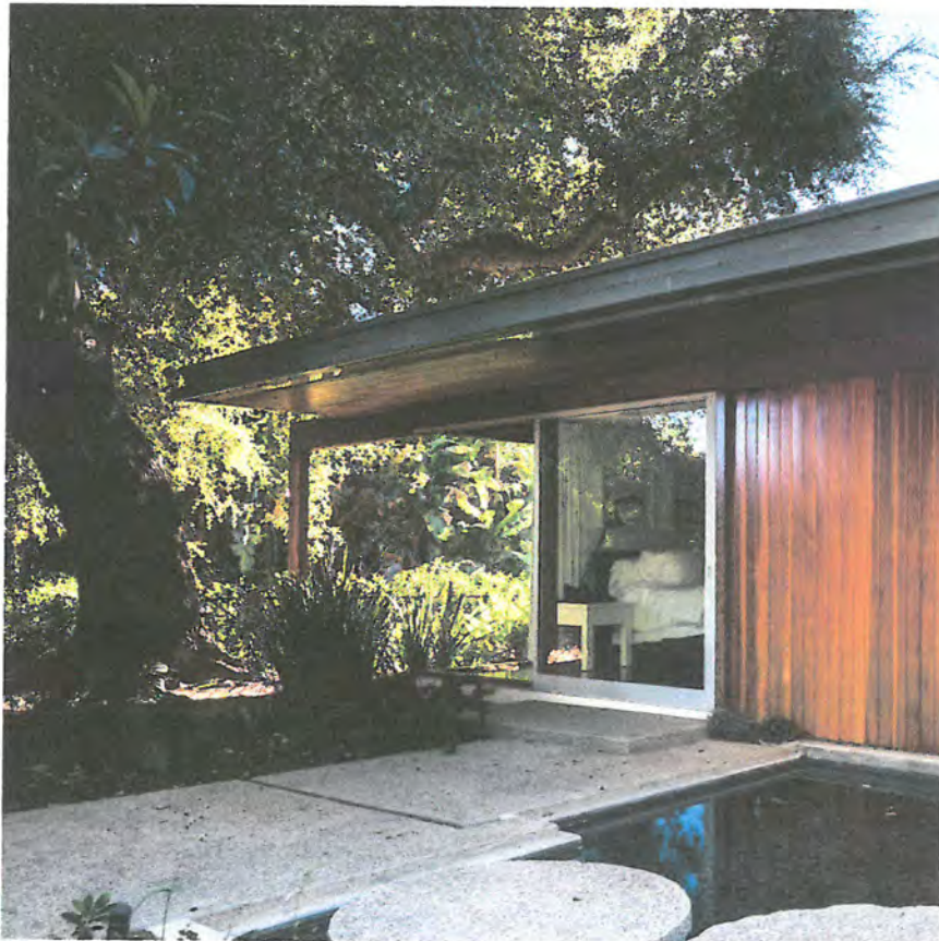
Contemporary Figure 6. East elevation, south end. Camera facing SW. Milton Goldman House, 2016. Photo by Darren Bradley.
