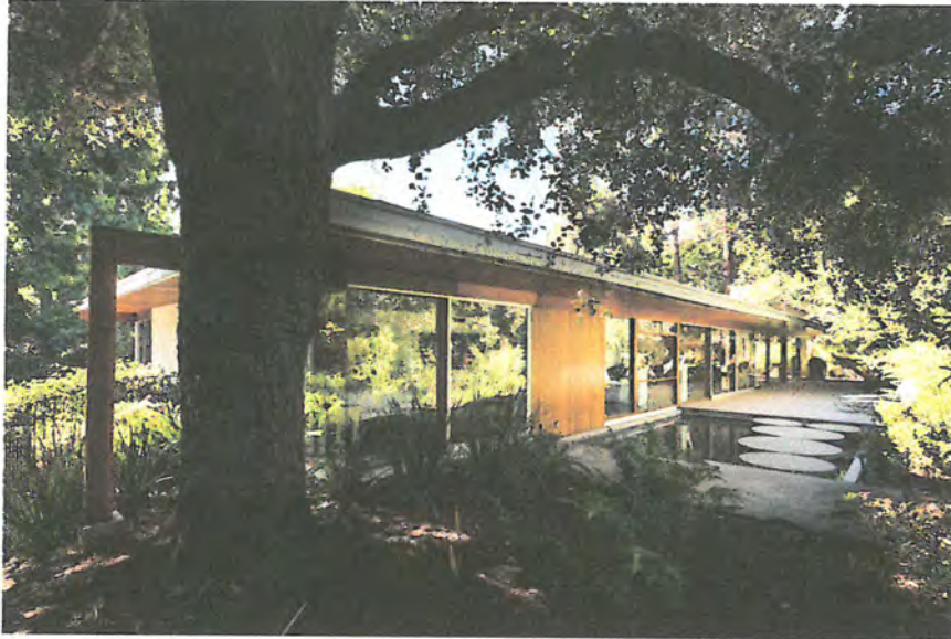
Contemporary Figure 5. East elevation. Camera facing NW. Milton Goldman House, 2016. Photo by Darren Bradley.
