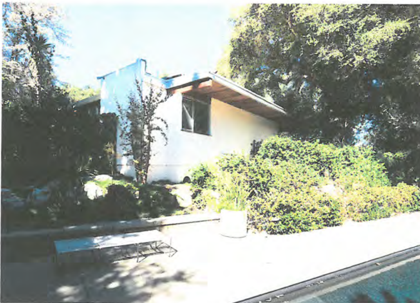
Contemporary Figure 4. South elevation. Camera facing NE. Milton Goldman House, 2016. Photo by Darren Bradley.
