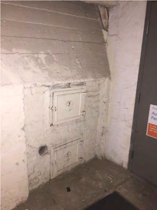
Figure 55. Incinerator on East side of basement
