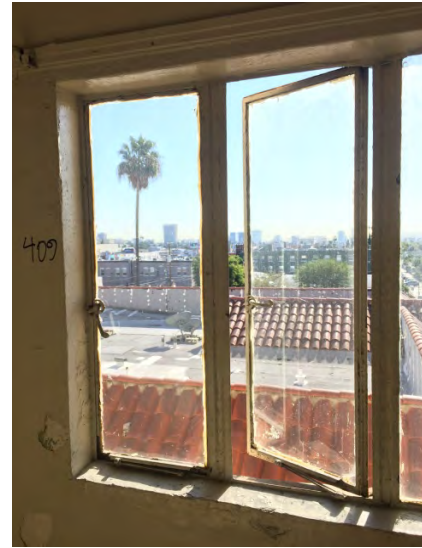
Figure 40. Steel casement window
