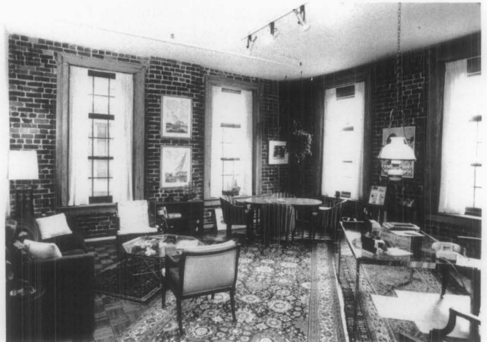
Figure 10. In this case plaster has been removed from perimeter walls, leaving brick exposed. In removing finishes from historic masonry walls, not only is there a loss of historic finish, but raw, unfinished walls are exposed, giving the interior an appearance it never had. Here, the exposed brick is of poor quality and the mortar joints are wide and badly struck. Plaster should have been retained and repaired, as necessary.
