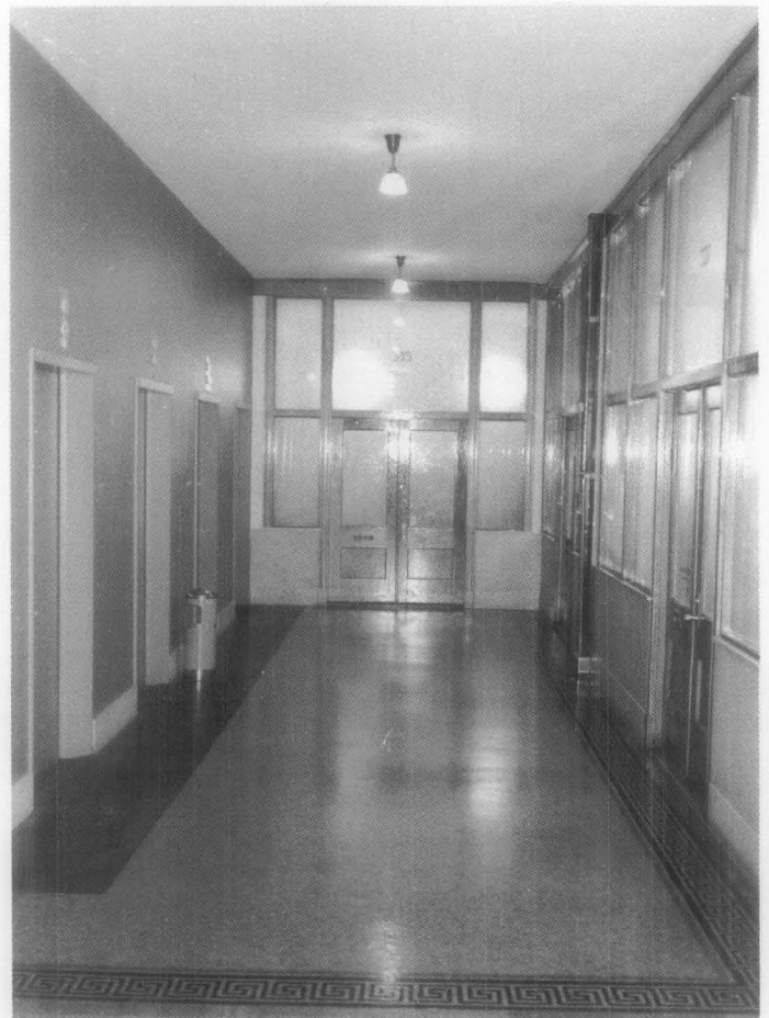
Figure 6. This corridor, located in the historic Monadnock Building in Chicago, has glazed walls, oak trim, and marble wainscoting, and is typical of those found in late 19th and early 20th century office buildings. Despite the simplicity of the features, a careful attention to detail can be noted in the patterned tile floor, bronze mail chute, and door hardware. The retention of corridors like this one should be a priority in rehabilitation projects involving commercial buildings.
