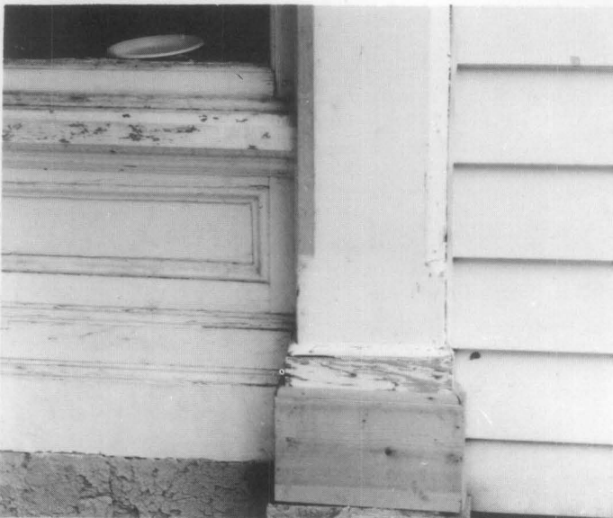
Figure 9. Rather than replace an entire wooden storefront when there is only localized deterioration, a new wooden component can be pieced-in, as seen here in this column base. The new wood will need to be given primer and top coats of a high quality exterior paint—either an oil-base or latex system. Also wood that is flaking and peeling should be scraped and hand-sanded prior to repainting. Photo: H. Ward Jandl
