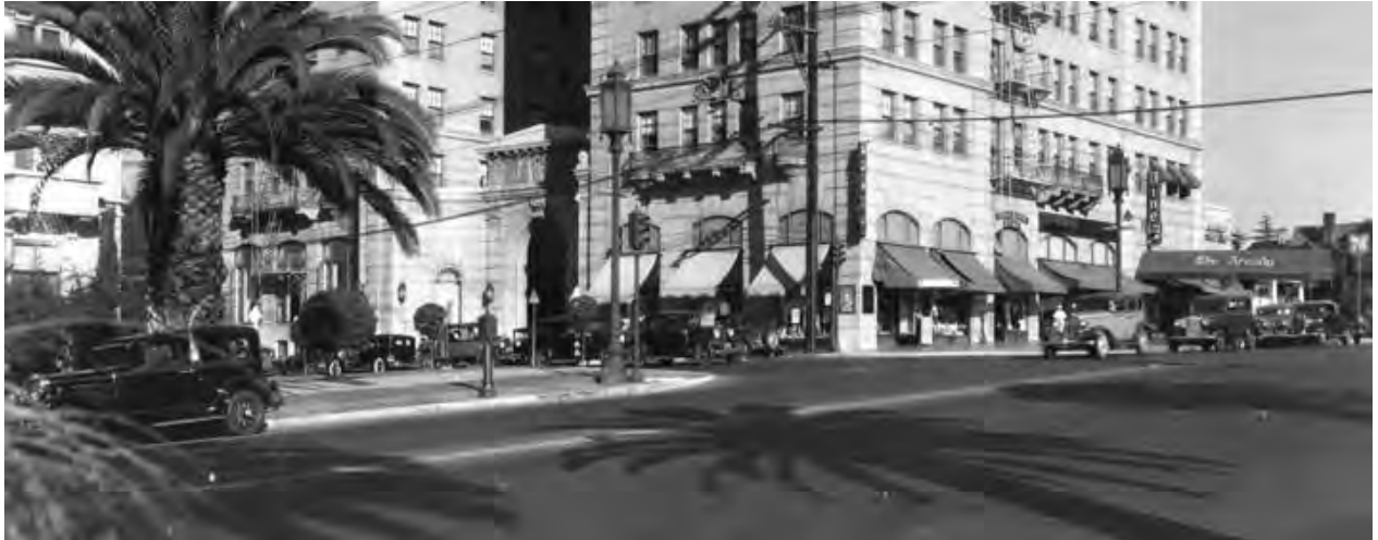
Initial arched entry was located between the two primary wings. It was damaged by earthquake in 1971 and removed.
