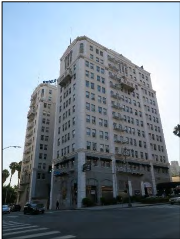
Primary, west and south elevations, view northeast (2017)
