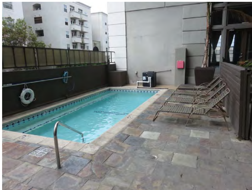
Pool and surrounding deck installed in 1982. The pool is located in the exact position of the original arched entry portal which is visible in the historic photo. This alteration fundamentally changed the function of this area from an entrance and courtyard, to what is effectively now a private deck between the two flanking wings of the building, with no relationship to the street.
