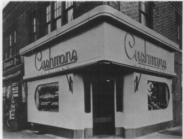
Figure 4. This storefront in New York City designed by Raymond Loewy typifies the streamlined look of the 1930's. Added to an earlier building, the front utilizes glass, stainless steel and neon to make a modern statement. This is a good example of a later storefront which has acquired significance and should be retained in any rehabilitation.
