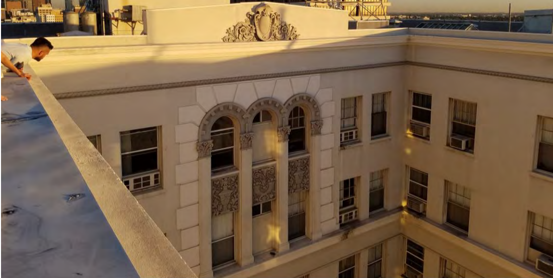
Upper façade ornamentation and cornice details. The window openings are evenly spaced. Window air conditioning units have a minor impact on the integrity of the appearance of these primary elevations, although there is no real alternative without major intervention to the interior.
