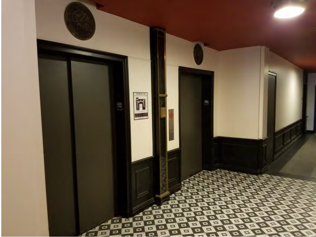
Upper floor upgrades include the elevator area, including repainting and installation of new floor tiles. The original bronze mail chute was retained on all floors. Oval panel is the former elevator indicator, left in place although not functional.
