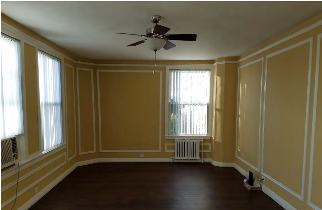
Existing apartment units, after renovation, retain typical details, including millwork on wall surfaces, and window framing
