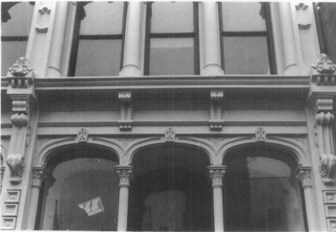
Figure 8. When the Grand Opera House in Wilmington, Delaware, was rehabilitated, missing cast-iron columns were cast of aluminum to match the original; in this particular case, because these columns do not carry great loads, aluminum proved to be successful substitute. Photo: John G. Waite
