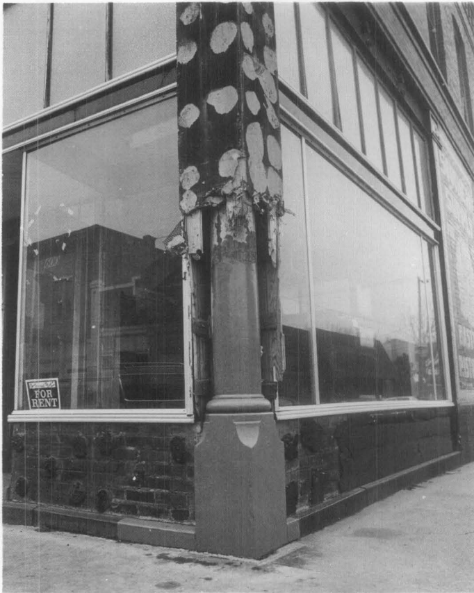
Figure 6. Storefronts of the 1940's, 50's, and 60's were frequently installed by attaching studs or a metal grid over an early front and applying new covering materials. If the existing storefront is a relatively recent addition with little or no architectural merit, begin by removing the covering materials in several places as was done here. If this preliminary investigation reveals evidence of an earlier front, such as this cast-iron column, carefully remove the later materials to assess the overall condition of the historic storefront. The black mastic visible on the lower masonry panels was used for installing pigmented structural glass. Some attachment methods for modern facings, such as mastic or metal lath, may have seriously damaged the original fabric of the building, and this must be taken into account in the rehabilitation process. Photo: Bob Dunn
