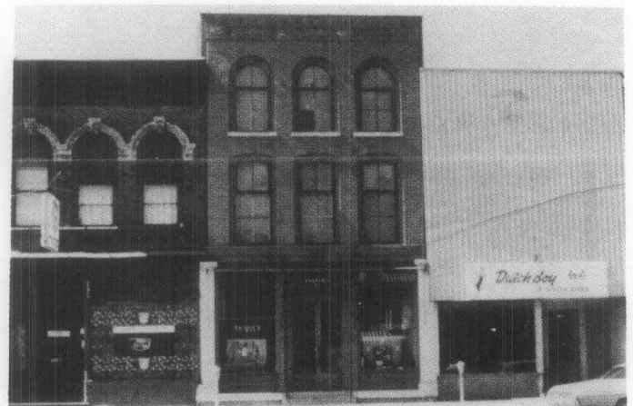
Figure 12. This photograph of three late 19th century commercial buildings clearly shows the impact of preserving and rehabilitating storefronts. The one on the right has been totally obscured by a "modern" front added in the 1950's. Although inappropriate alterations have taken place on the left storefront, it is still possible to determine the original configuration of the doors and display windows. The storefront in the middle has remained intact. Although in need of some minor maintenance work, the appeal of the original design and materials is immediately apparent.
