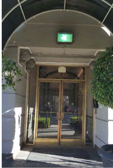
Detail, Current entrance off Wilshire Boulevard, opening into the corridor that accesses the main entry.
