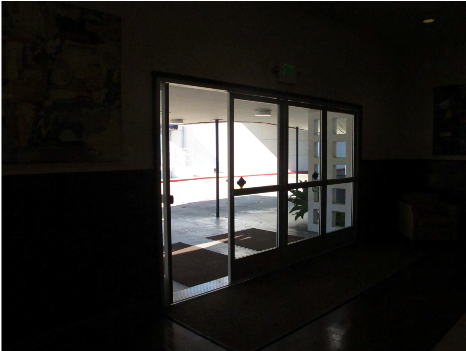
Detail: Auditorium entry masonry block
