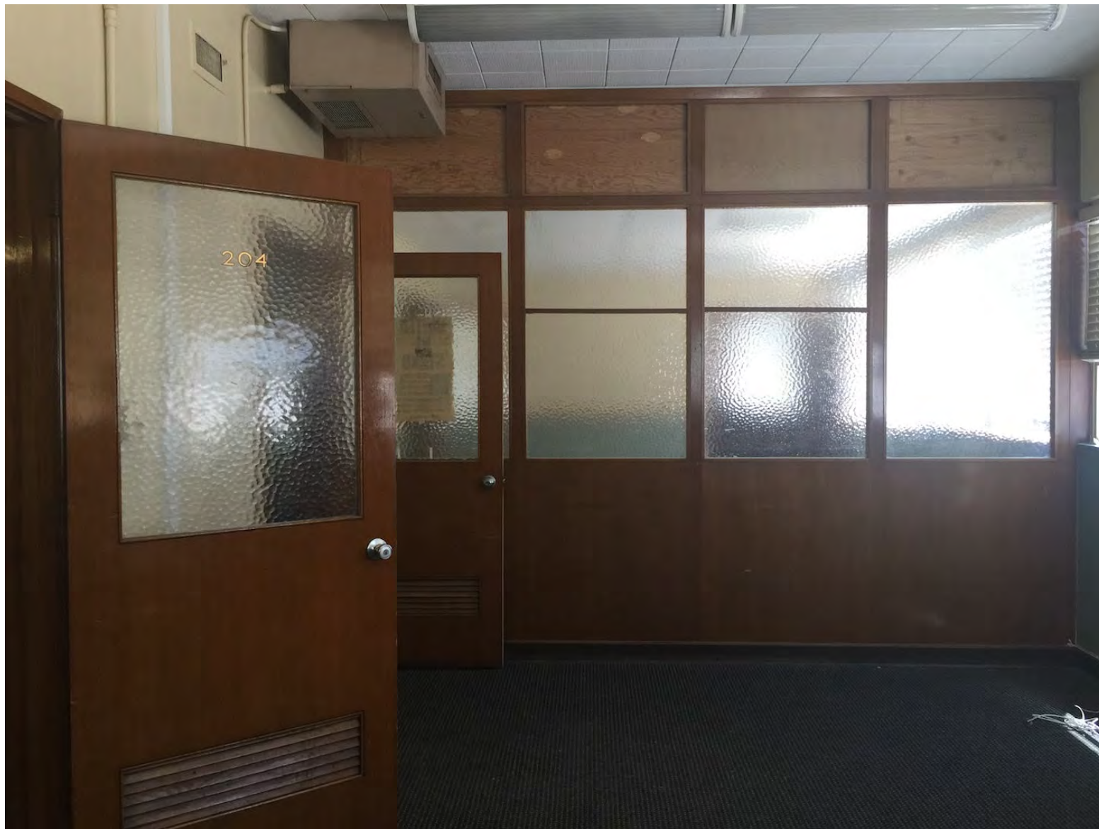
Second floor office
