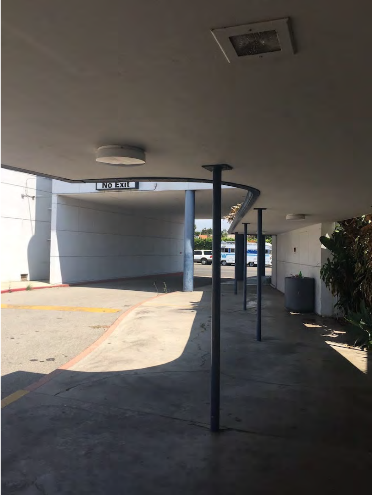
Porte cochere and street entry
