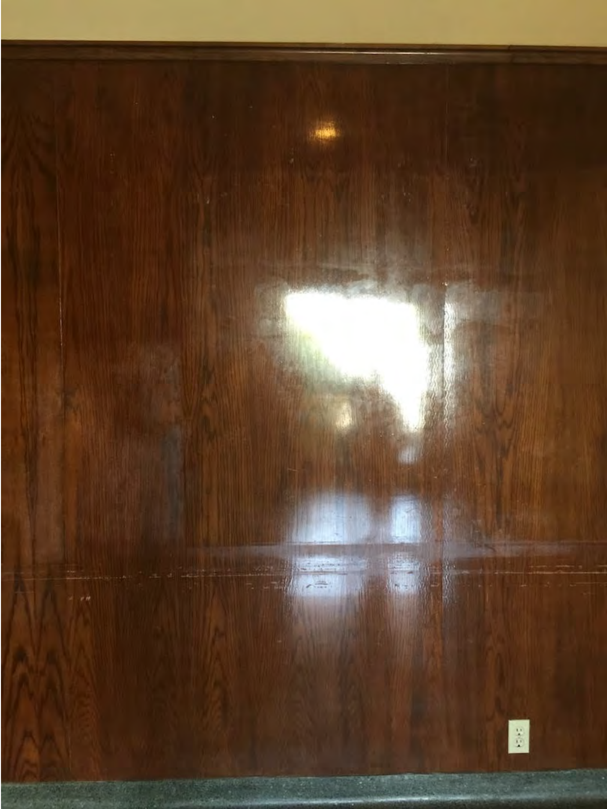
Detail: Wood paneling
