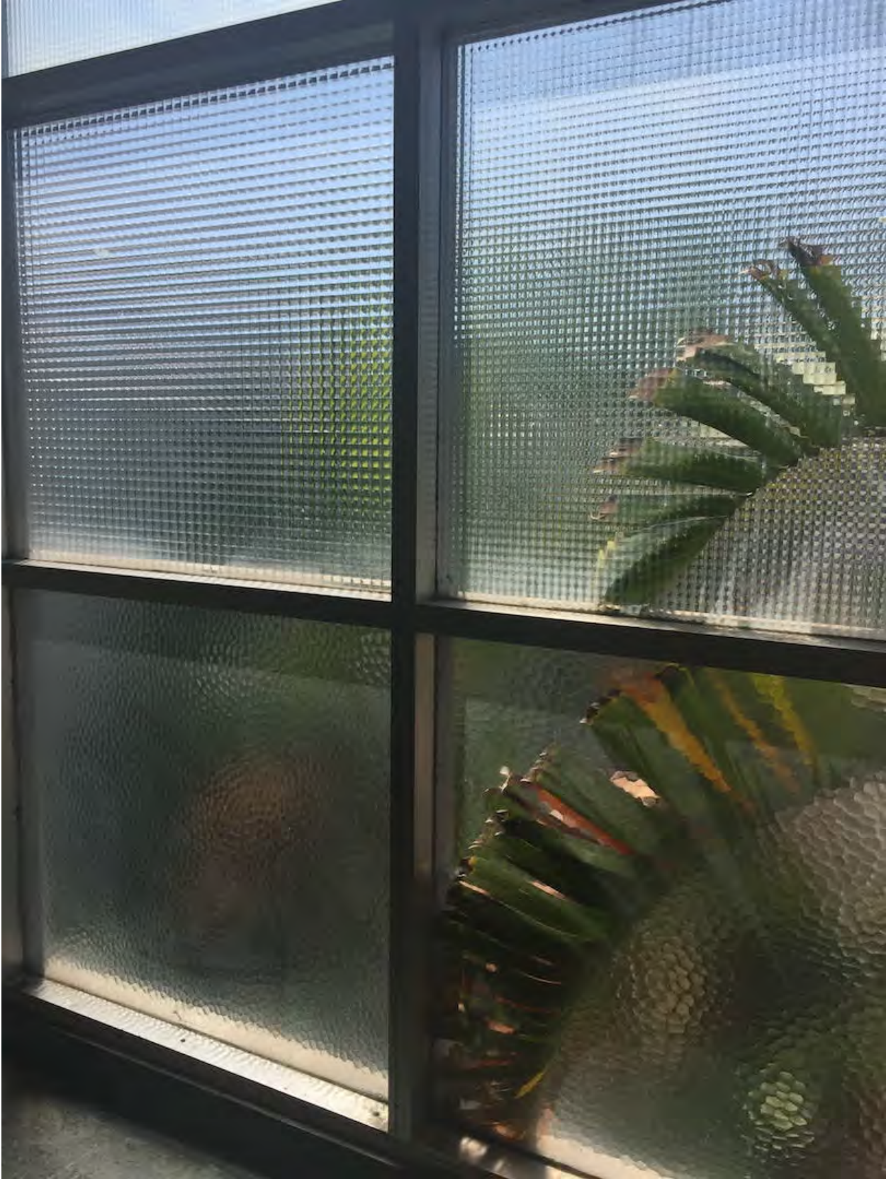
Detail: Stairwell window
