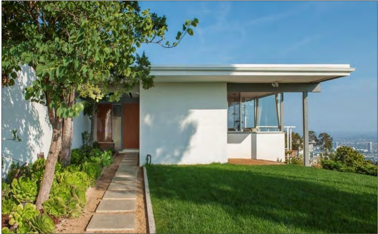
Figure 3: Chuey Residence, west elevation, view east of main entrance (source: MLS, 2017)
