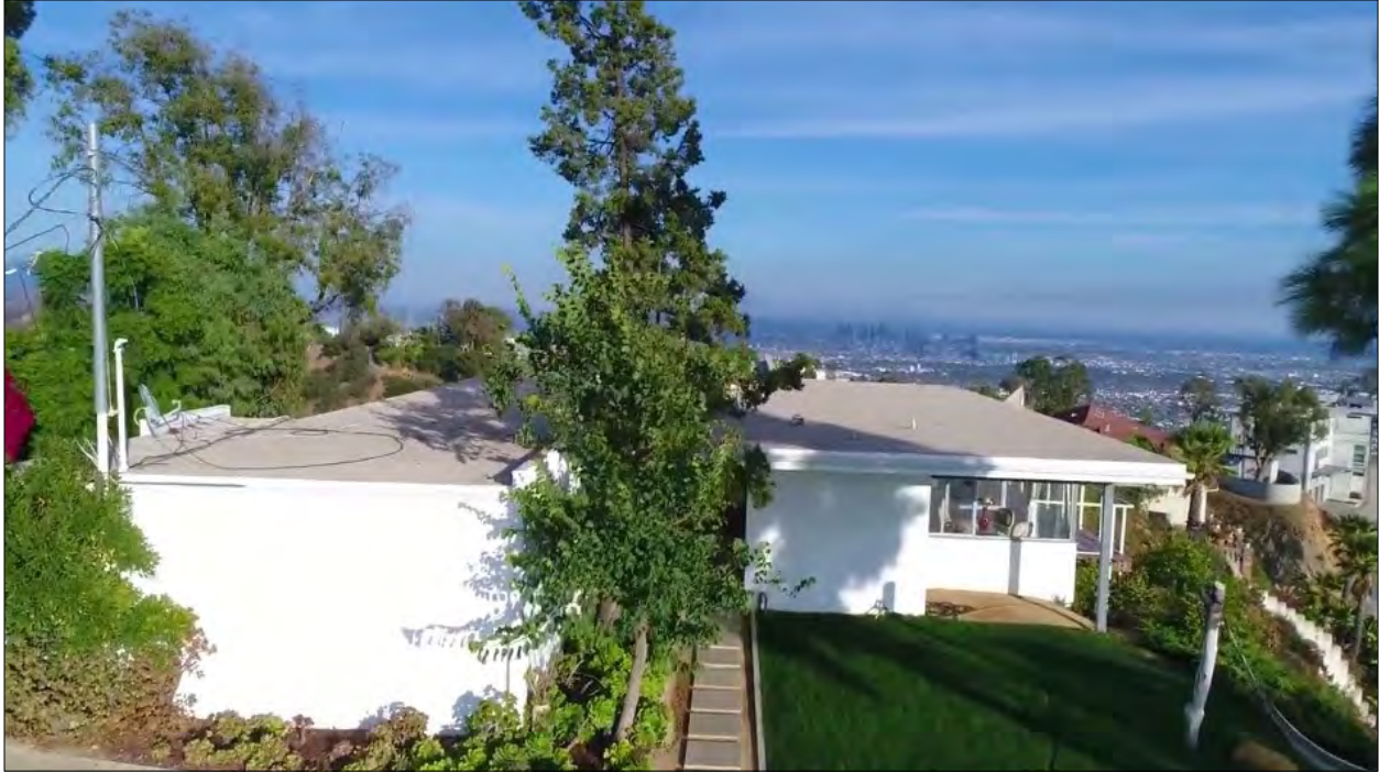
Figure 1: Chuey Residence, west elevation, view east (source: Berlyn Media, 2017)
