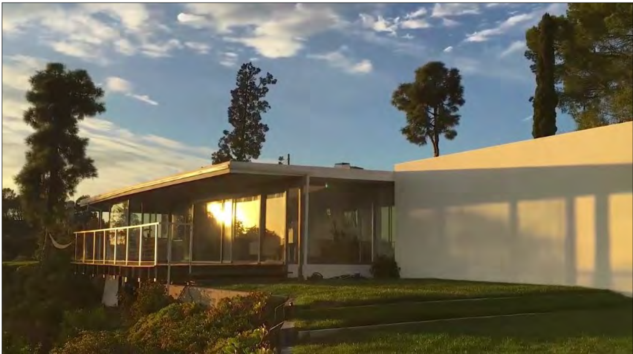
Figure 8: Chuey Residence, south elevation, view northwest (source: Berlyn Media, 2017)
