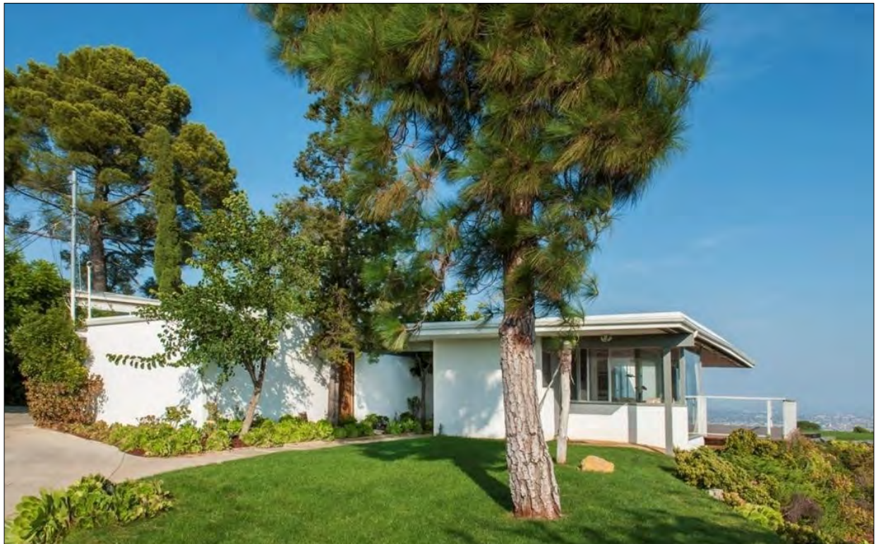
Figure 2: Chuey Residence, west elevation, view northeast (source: MLS, 2017)
