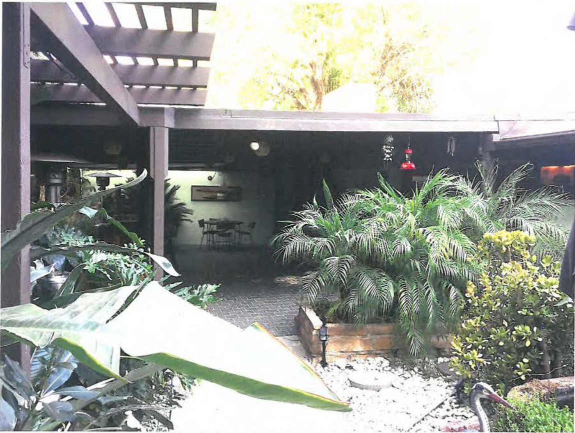
6134 Jumilla Avenue, new wooden lattice shade structure in foreground dating from 1989.
