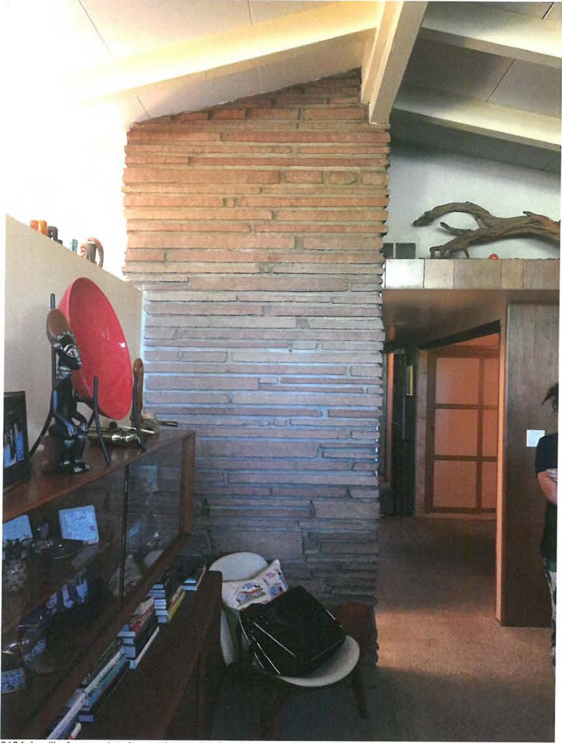
6134 Jumilla Avenue, interior sandstone detail wall between living room and kitchen.
