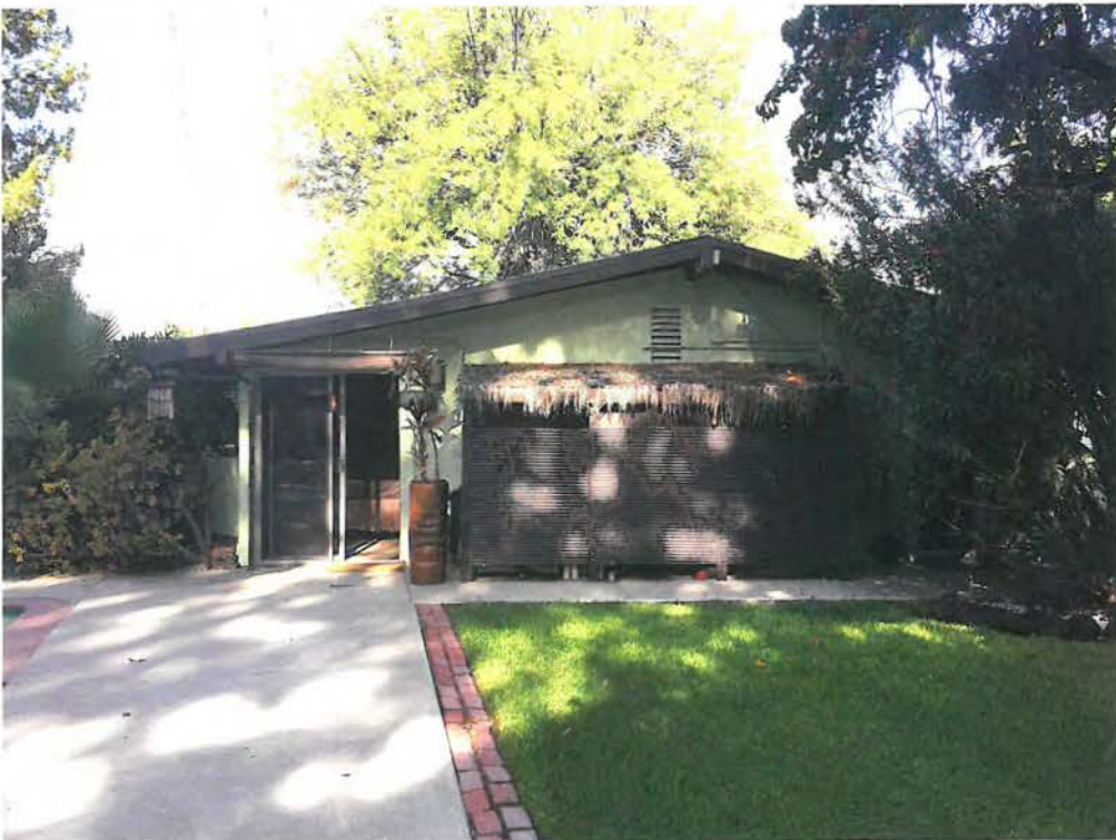
6134 Jumilla Avenue, east façade
