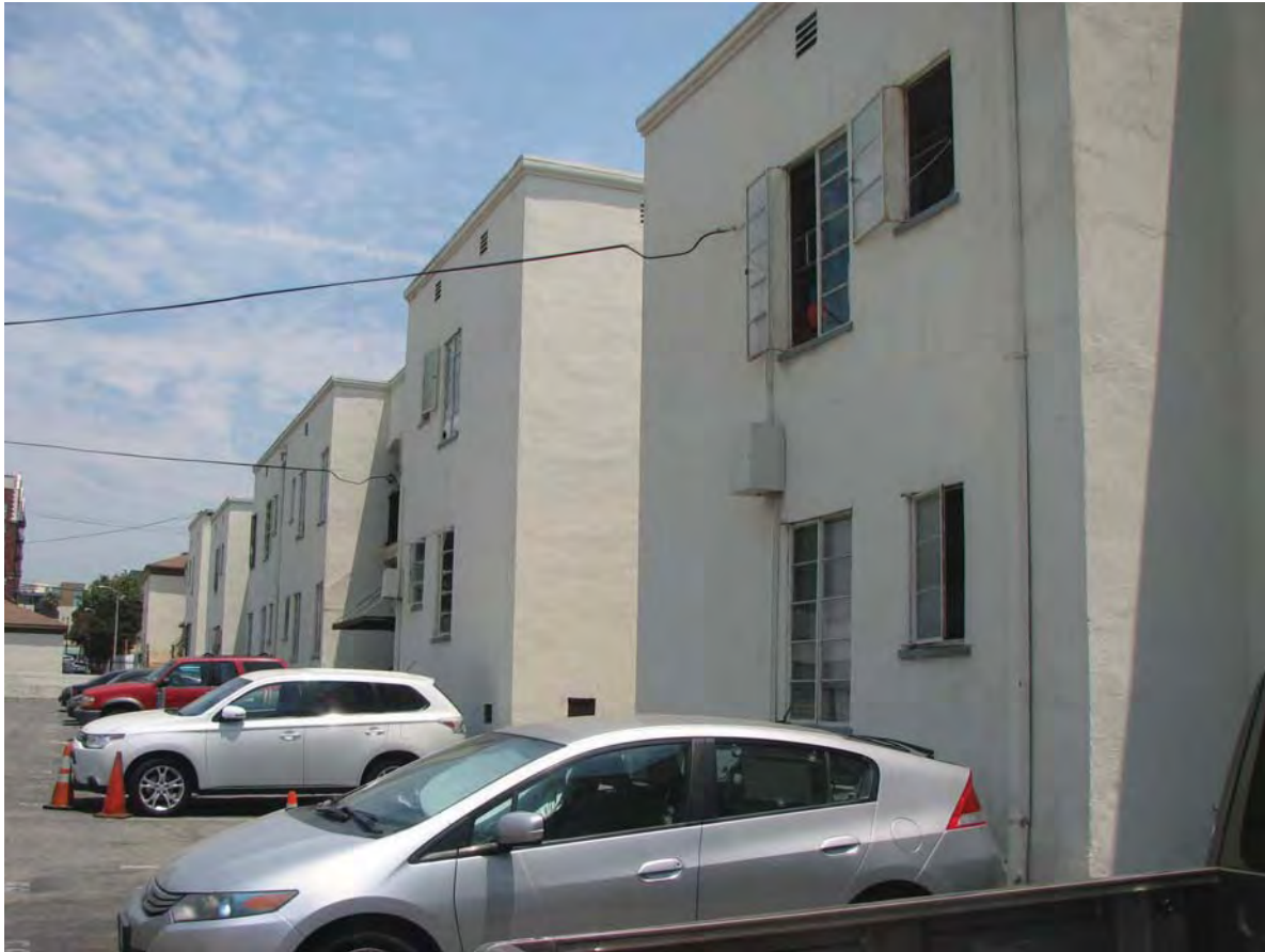
Selma Las Palmas Courtyard Apartments, rear facades, 1535-55 N Las Palmas, July 13, 2017 (Photograph by Charles J. Fisher)
