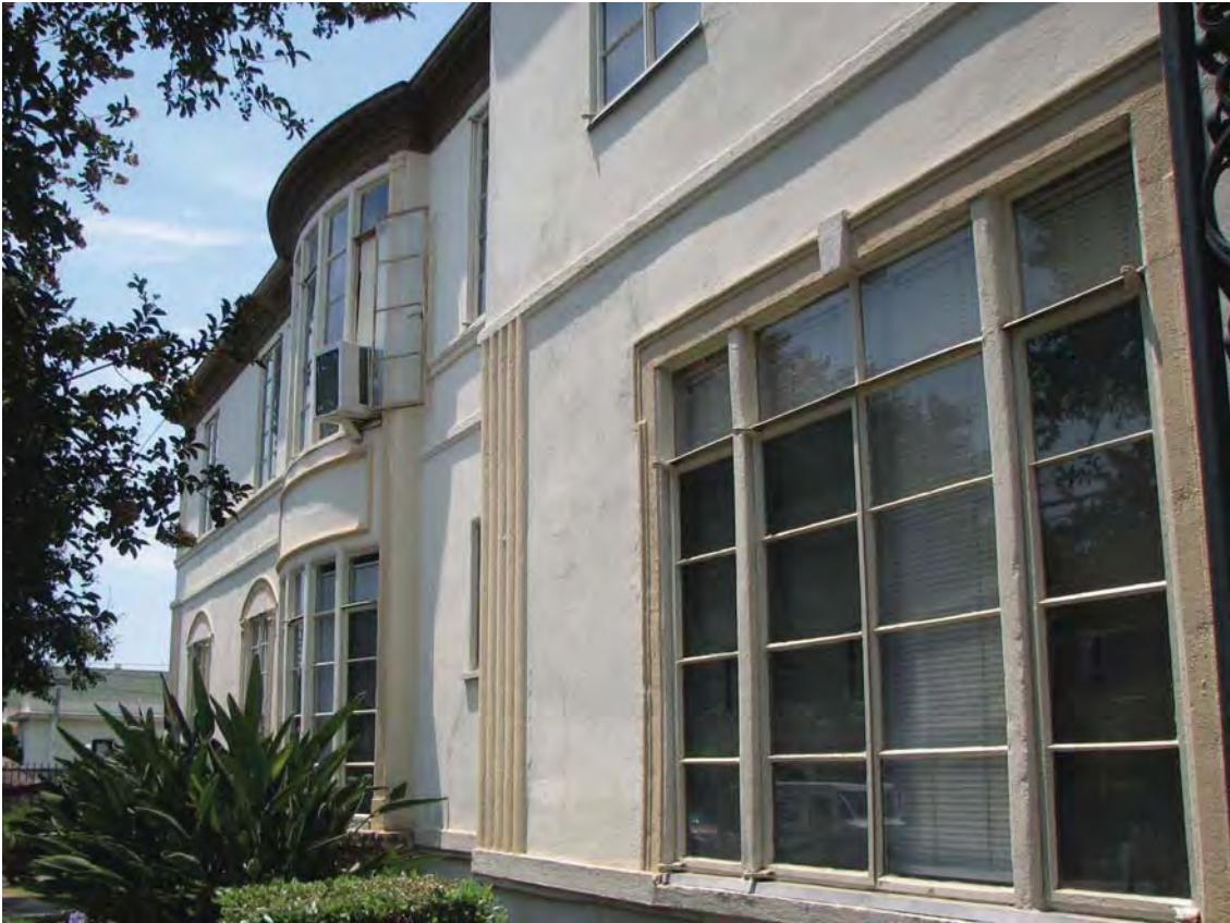
Selma Las Palmas Courtyard Apartments, 1535 N Las Palmas Avenue, July 13, 2017 (Photograph by Charles J. Fisher)
