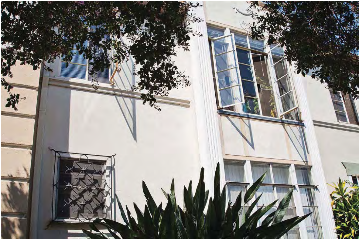
Selma Las Palmas Courtyard Apartments, steel casement windows & an original window grate, 1545 N Las Palmas Avenue, September 11, 2017 (Photograph by Susan Hunter)
